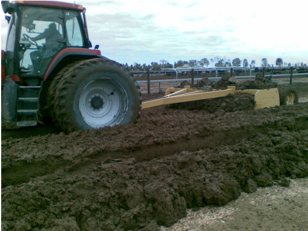
Photograph 3 – Pen cleaning using a box scraper under wet conditions
