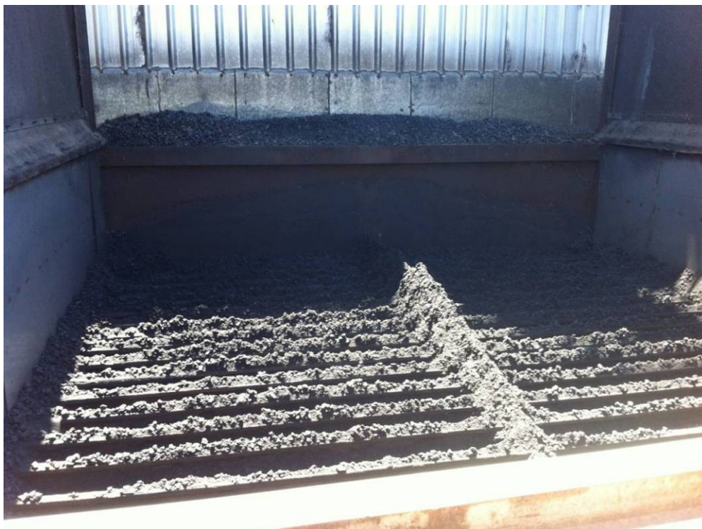
Photograph 25 – Coal bunker opening
