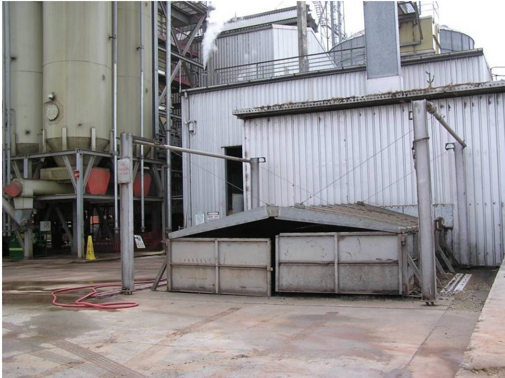
Photograph 24 – Coal bunker – covers in place
