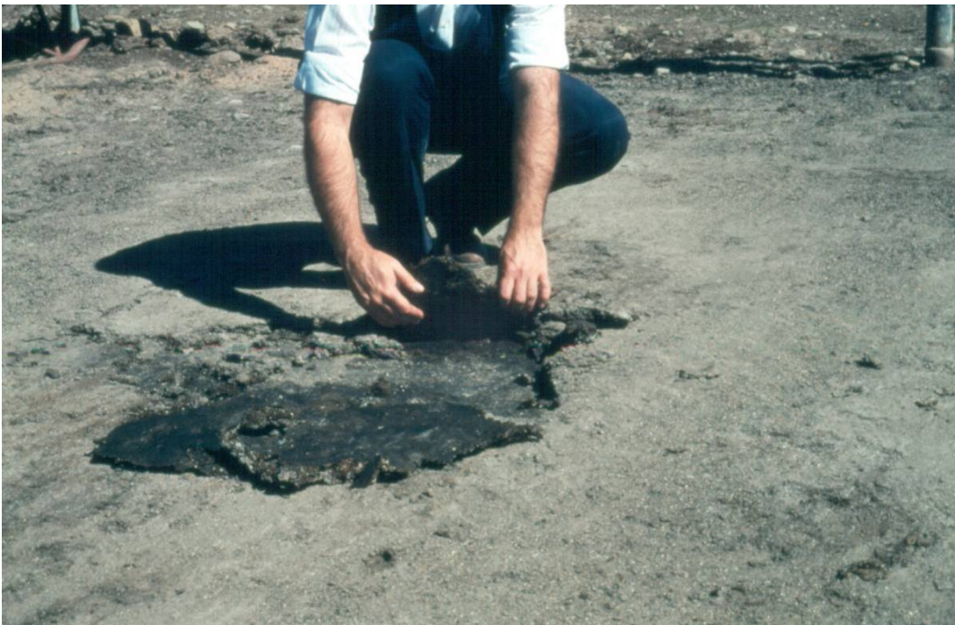
Photograph 4 – Example of the compacted manure interface layer
