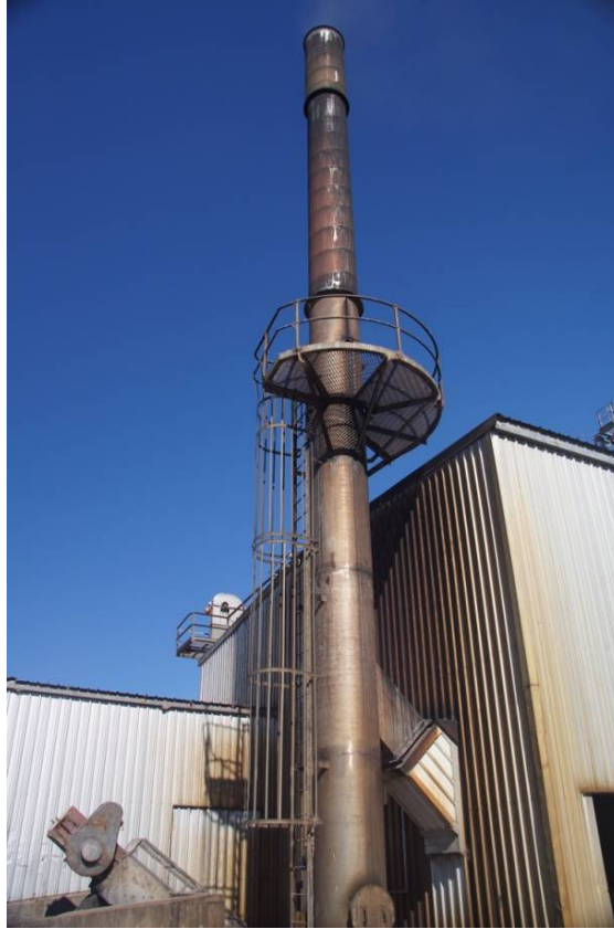
Photograph 28 – Flue with platform at mid height
