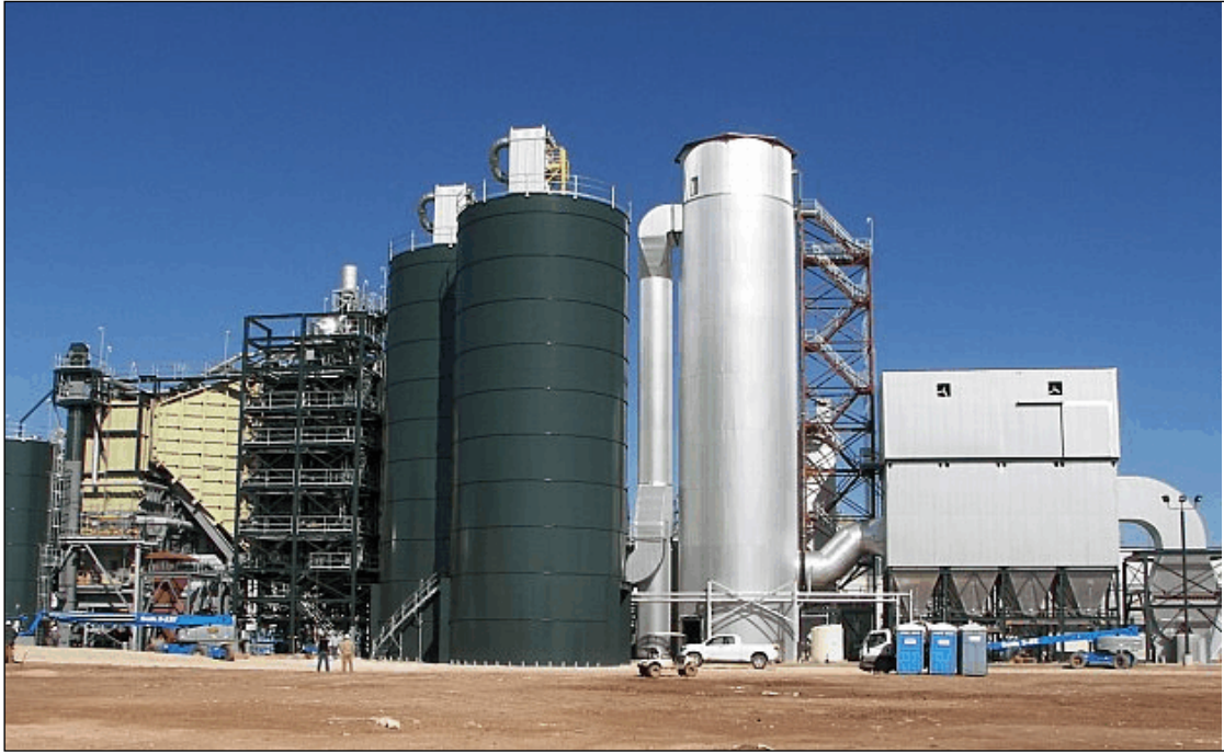
Photograph 9 - Panda Energy beef feedlot manure combustion facility
