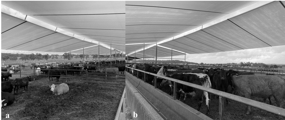
Figure 19. A and B show the shelter structure over the Tullimba research feedlot pens
