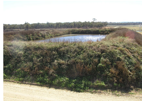
A turkey nest storage situated high above the feedlot allows gravity flow of water around the site.
