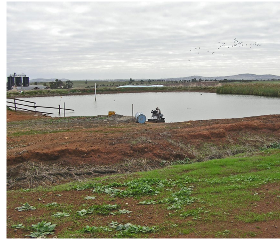
Water storage at a higher elevation than the feedlot allows gravity flow of water.
