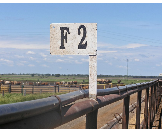
Polyethylene water pipeline attached to top rail of fence will allow water to heat up during hot weather and is not recommended.
