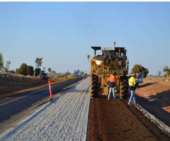
Stabiliser machine mixing binder agent into road base material.
