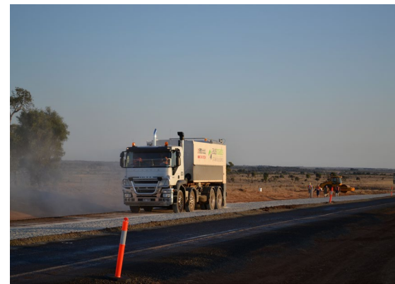
Spreader truck spreading dry binder agent onto base material.
