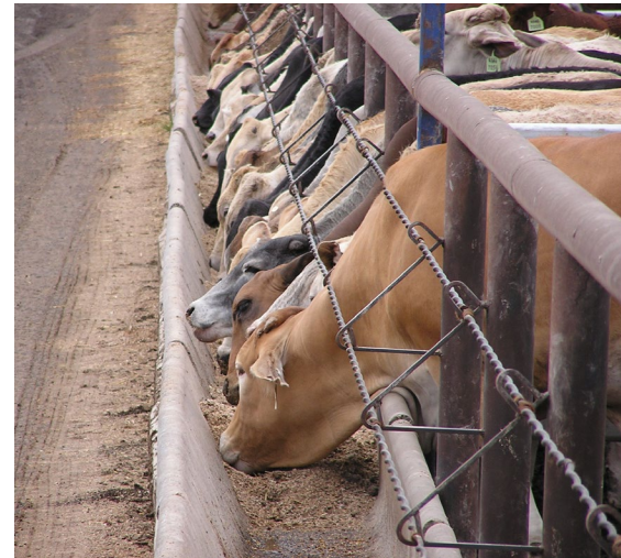
Individual pre-cast section feed bunk Type C. This cable arrangement makes trough cleaning more difficult; a single rail is usually sufficient to confine cattle.
