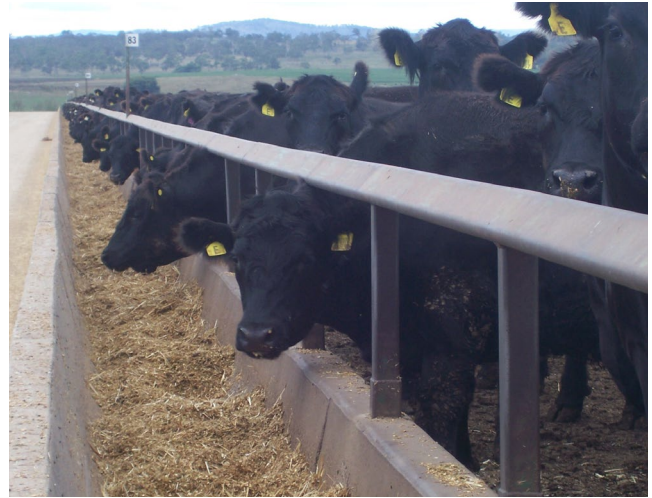
Single steel bar cattle restraint with posts cast into the back wall of the feed bunk
