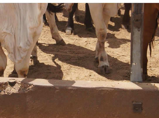
A rusted or broken post has been replaced with a new post bolted to the back of the wall.
