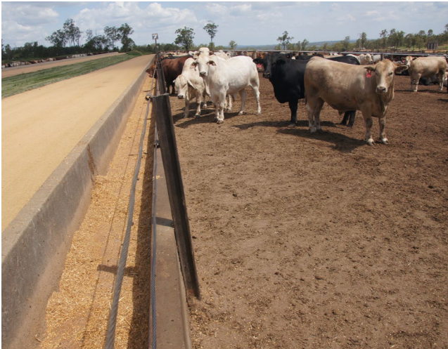
External posts of old cheap railway line will inhibit cleaning along the feed apron and lead to damaged posts and bunks.
