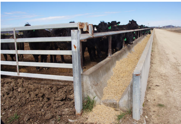
Feed Bunk type F with steel posts bolted to the top and rear of the back wall, with a single-bar cattle restraint. A steel bollard prevents damage to the end of the feed bunk.
