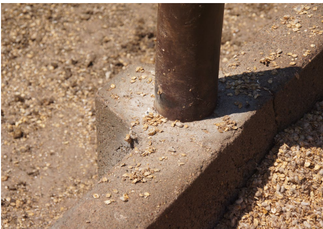
Local thickening of the feed bunk wall is strong but may make cleaning difficult.
