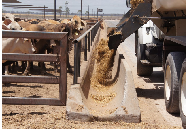
A concrete apron extending onto the feed road will reduce any impact on the feed truck load cells and give more control on feed delivery. The apron should slope gently away from the bunk, but still allow the truck driver to see into the bunk.
