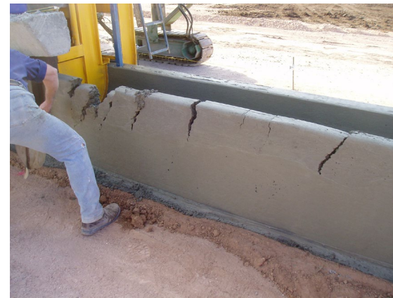
Good concrete mix with consistent moisture content is essential throughout the whole slip-form process—or problems will occur.
