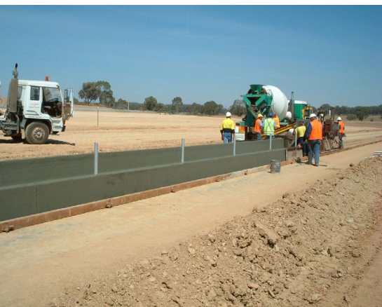
Finished concrete surface of feed bunk should be sprayed with curing oil immediately to minimise shrinkage and cracking.
