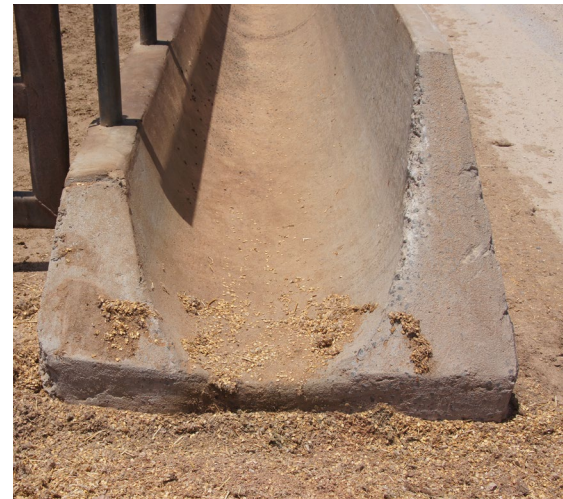
Feed Bunk Type G on concrete apron. Front wall slopes towards the pen.
