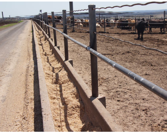
Feed Bunk Type D An old design with a cross-sectional area that does not hold enough feed, and the back wall is too low.
