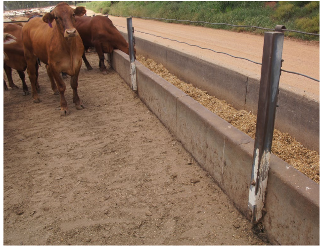
Posts bolted behind the back wall are more readily replaced but can hinder cleaning along the feed apron.
