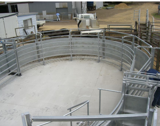
Parallel curved race with no inner sheeting.
