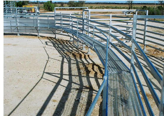
Catwalk on bugle yard
