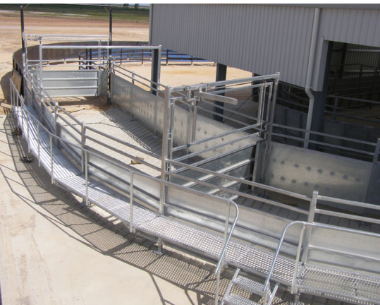
Forcing pens (bugle) with slide gates and catwalk with safety handrail.
