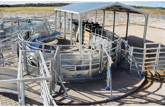
Complete handling centre with roof cover over crush area.
