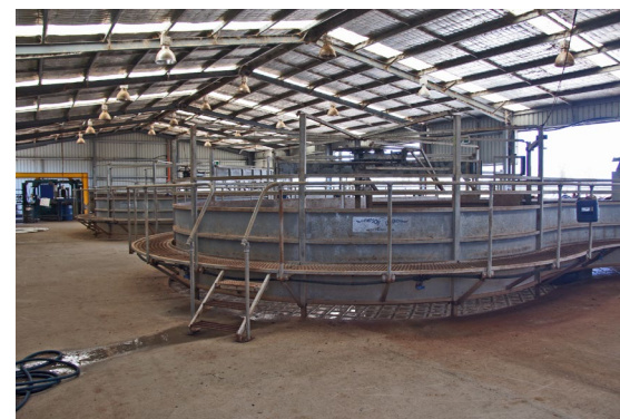
Steel frame building over entire processing area. Lighting is provided with clear roof sheets and artificial lamps.
