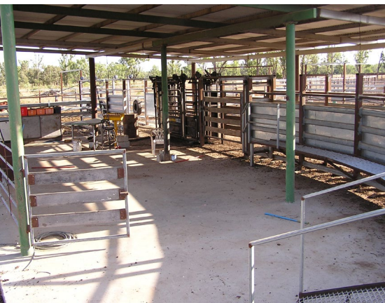
Steel and timber roof over crush, race and handler working area only.
