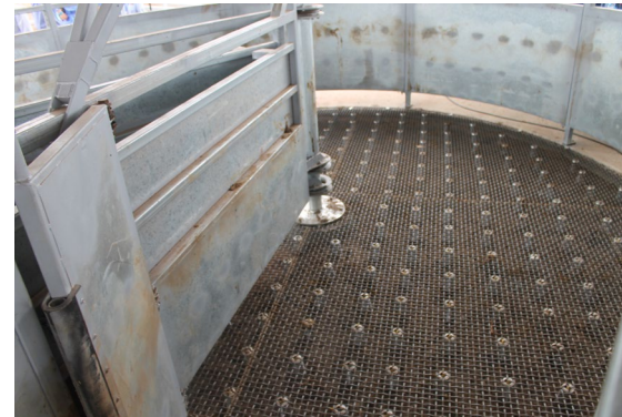
Suspended woven-mesh floor. The mesh is securely attached to the top of aluminium stirrups.
