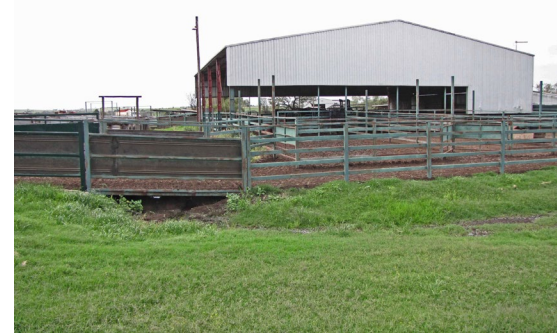
Steel frame building over entire processing area. One third of the shed is fully enclosed for storage and two side walls are half-sheeted from the top for protection against rain and wind. The north-facing wall is not sheeted.
