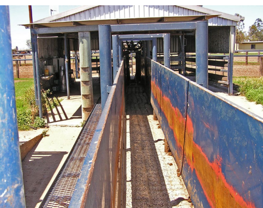
Steel frame structure over crush with half-sheeted walls. Sharp contrast between dark shadows and bright sunlit areas could make cattle baulk.
