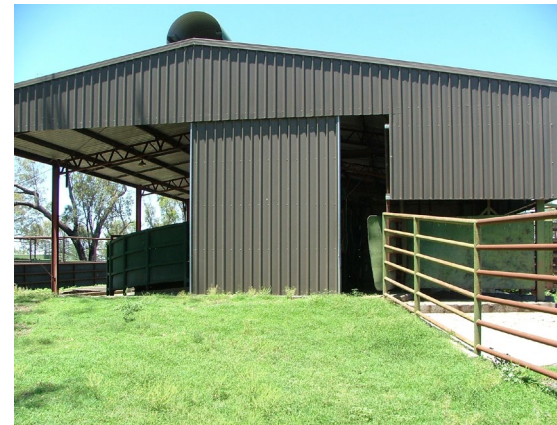
Steel frame building over the entire processing area. It is partially enclosed for protection against rain and wind, with a roof vent for ventilation.
