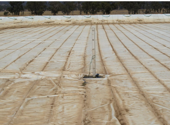
Covering emergency water storages helps reduce water evaporation and prevent access by wildlife and pests.
