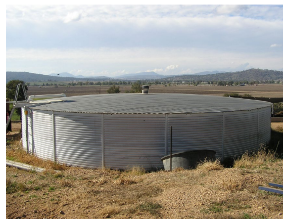
Steel or corrugated iron water storage tanks are available in a range of sizes and capacities.
