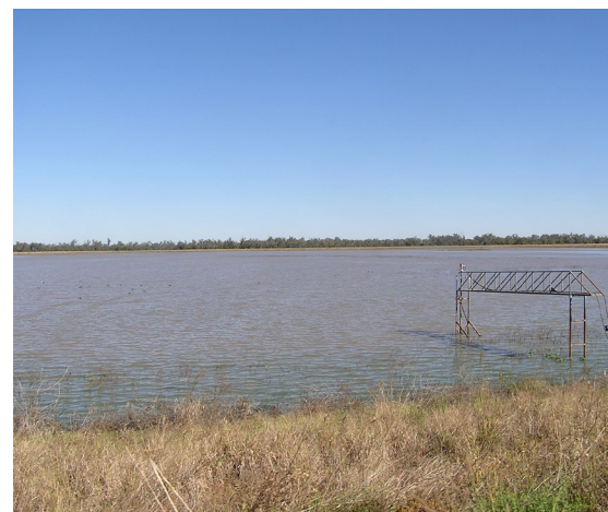
Land surface diversions need off-stream storages. Losses from evaporation and seepage can be large.
