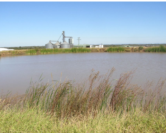
Uncovered turkey nest storage near a feedmill
