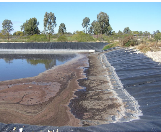
Synthetic liner to minimise water seepage
