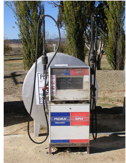
Fuel bowser with fuel-dispensing nozzle having a trigger valve mechanism, and product clearly identified.
