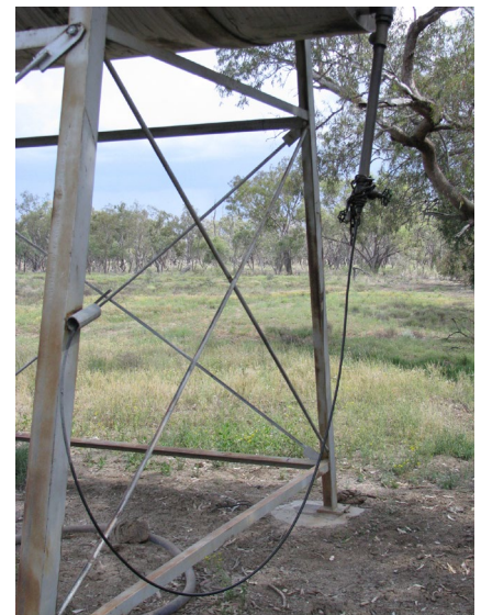
Feet pads above ground and secured to concrete pad with well-braced legs.
