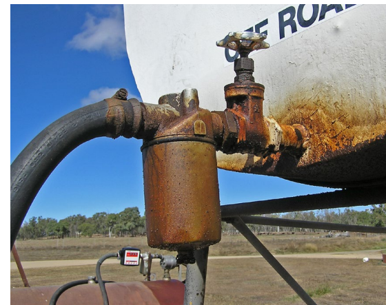
Isolation valve on dispenser is kept turned off except when dispensing fuel. Rust on the tank and outlet pipe needs to be treated.
