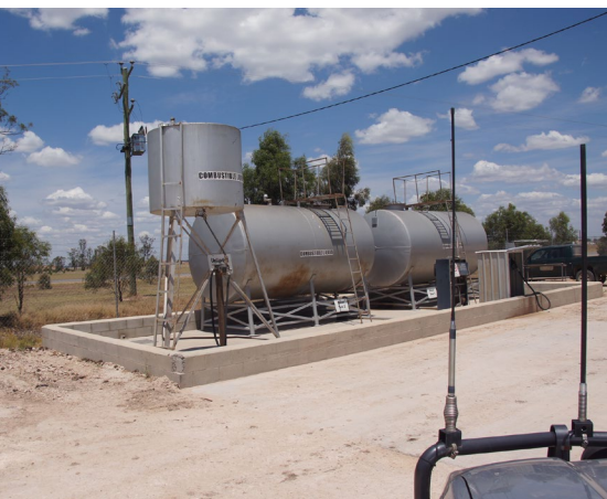
Impervious bunding around fuel storage tanks must be large enough to contain the combined capacity of the tanks plus 20 minutes of fire-control water.
