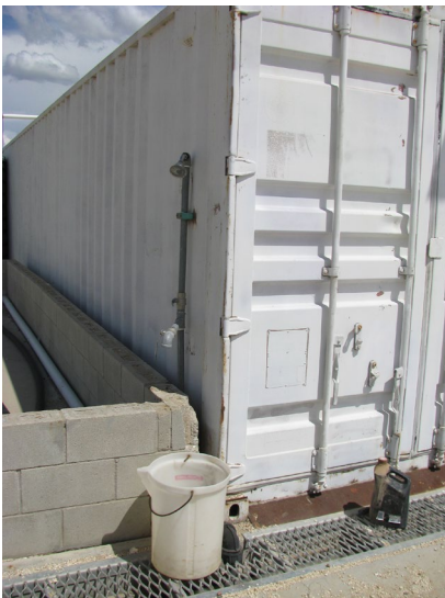
Shipping containers make an excellent storage facility for chemicals. Note the drain at the front of the container and shower on the left.
