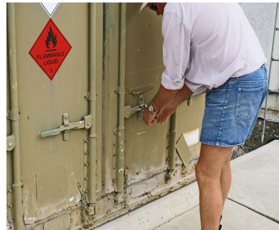
Security - The chemical store must be kept locked to prevent unauthorised entry, with windows and vents designed to keep out children or others.
