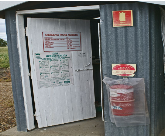
Appropriate signage should be clearly visible on the exterior of the storage facility.
