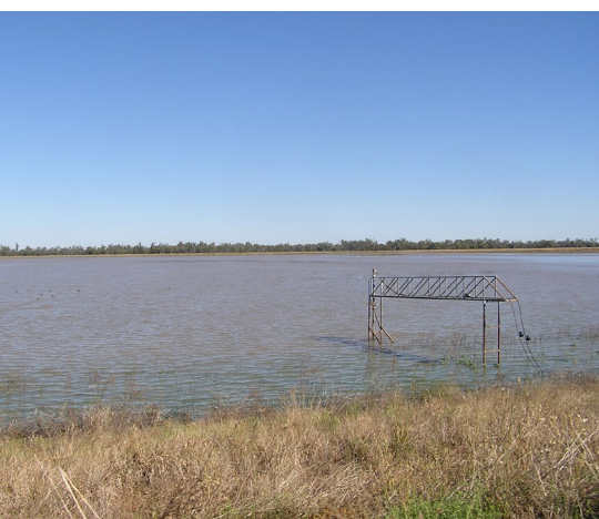
Large open-water storage areas can lose over 800 mm/year through evaporation.
