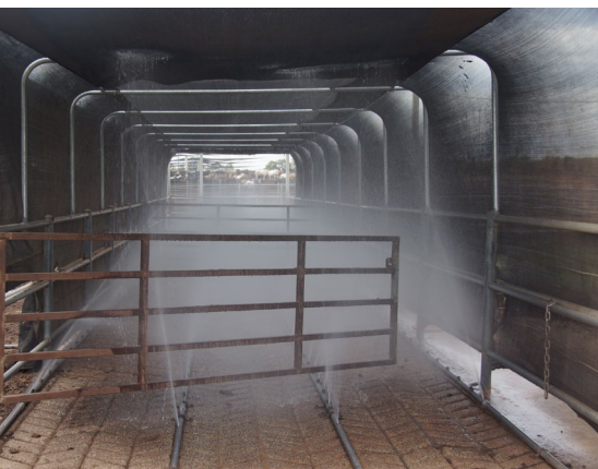
Soaking yard covered with shade cloth which redirects the spray water back down over the top of the animals
