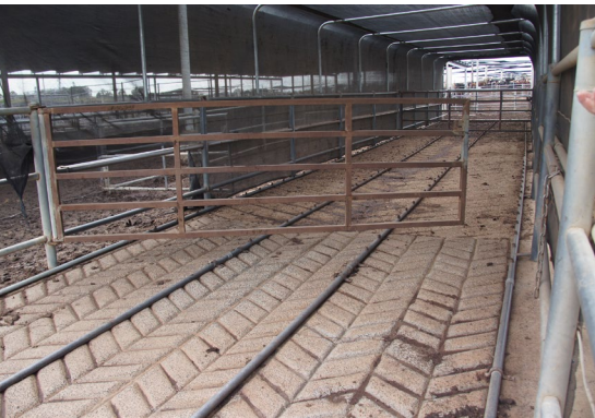
Gates provide access for cattle and equipment; hinged or overhead sliding gates are commonly used in a cattle wash.
