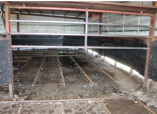
Overhead gates are safer and more practical than hinged gates for operators in confined areas, but are more expensive to construct and require mechanical assistance to operate.
