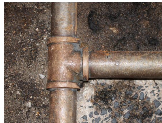
Holes drilled in pipes create a quick and cost effective spray system.
