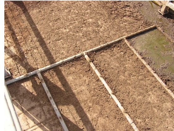
Above ground pipes can restrict drainage flow and trap manure. Nozzles can become clogged with manure.
