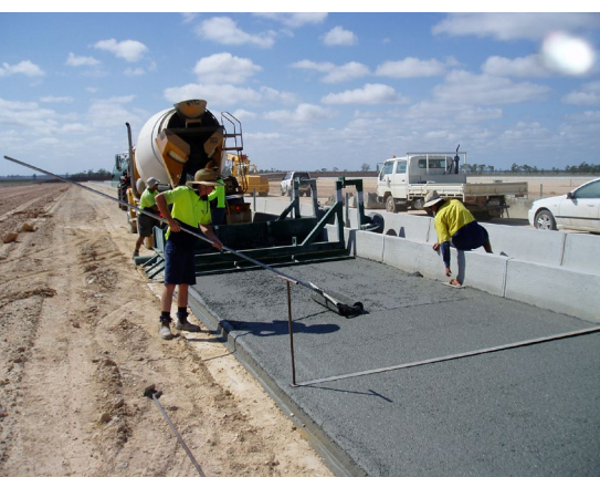
... for concrete works
