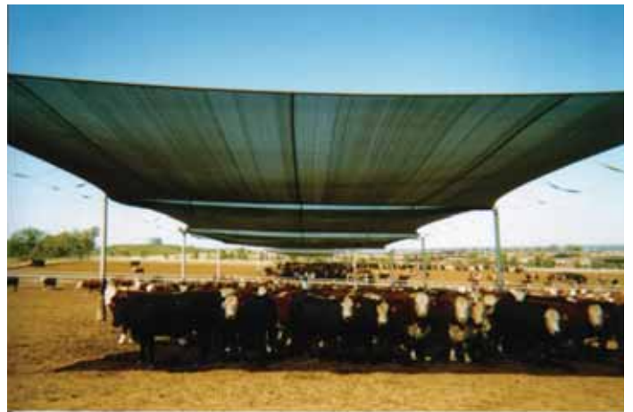
Figure 1: Feedlot shadecloth structure Photo courtesy of Rockdale Beef Pty Limited
