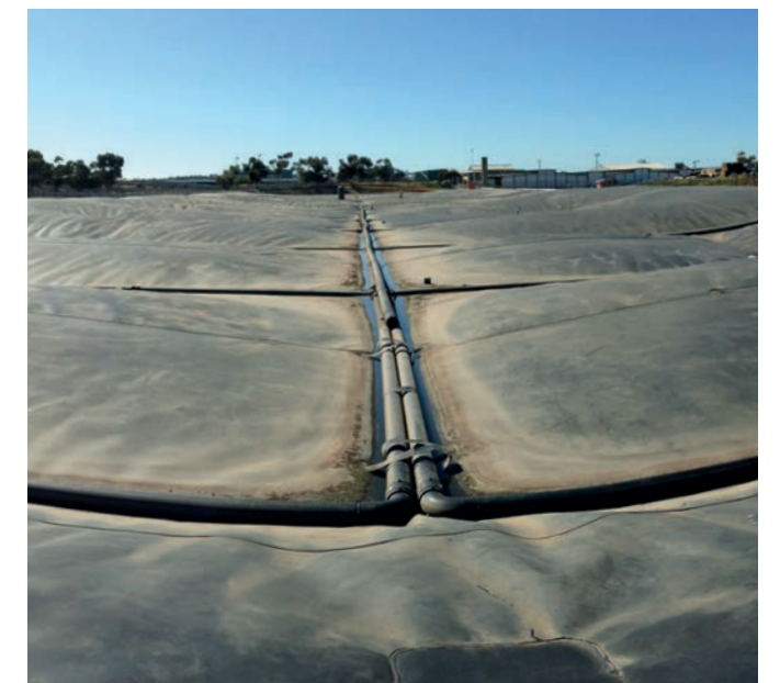
» Past success (2015-16): Covered anaerobic lagoons helped to generate energy, reduce greenhouse gas emissions and improve the quality of water discharged from Thomas Foods International's Murray Bridge plant.
