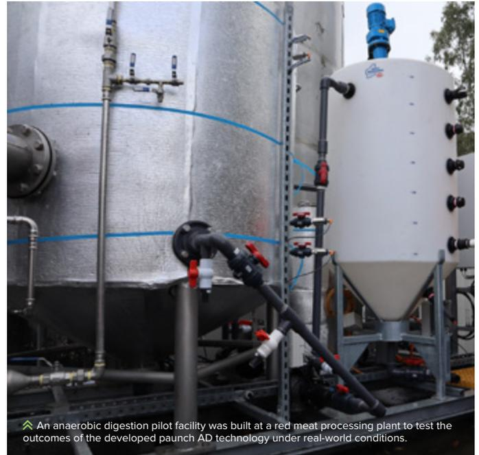
➡ An anaerobic digestion pilot facility was built at a red meat processing plant to test the outcomes of the developed paunch AD technology under real-world conditions.
