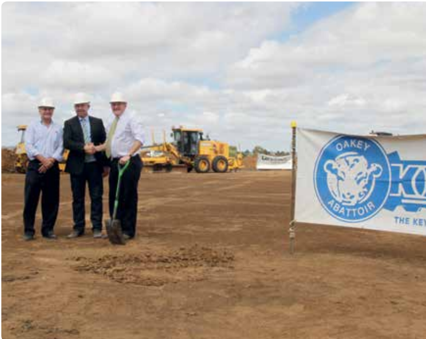
Turning the sod at the new waste-to-energy technology project at Oakey Abattoir: (L-R) Michael Bambridge – managing director of CST Wastewater Solutions, Pat Gleeson – general manager of Oakey Abattoir and the then Federal Minister for Industry, Ian Macfarlane.
