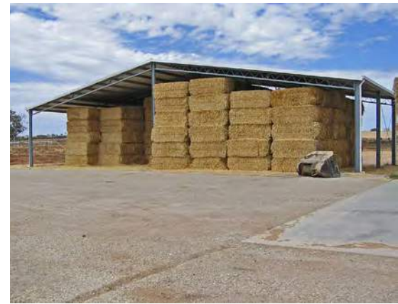
The large span of a steel framed, fixed roof open shed provides unrestricted access. Downpipes take roof water away from the storage area.
