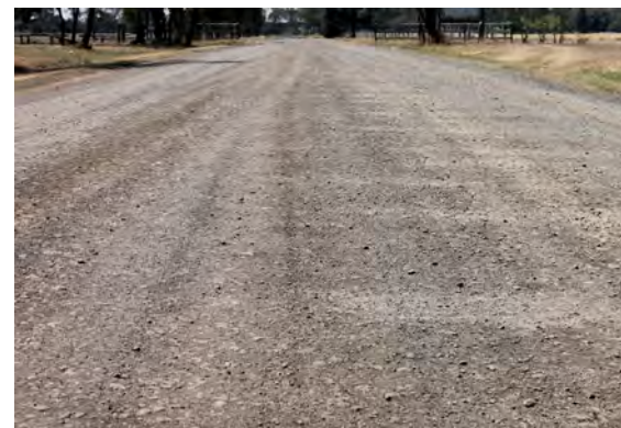
Unsealed road with a well-maintained and shaped crown, shoulder and v-drains
