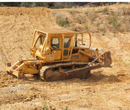
Bulk earthworks start with dozers...
