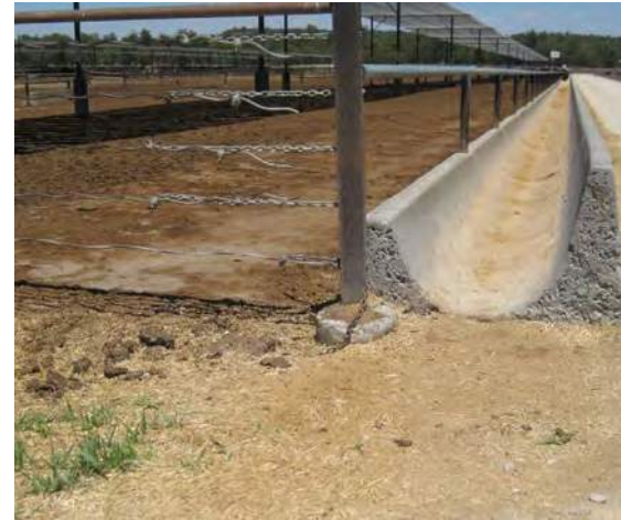
Feed bunk Type F on top of concrete apron.
