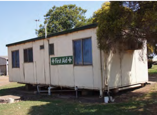
Modular relocatable building (a 'donga') used for a First Aid post.
