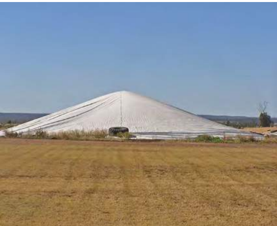
Covered grain stockpile in a bunker storage with small earthen walls.
