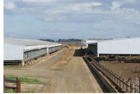
Roof water collection system
