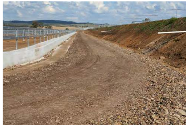
Feed roads need 2–3% slope for adequate drainage.
