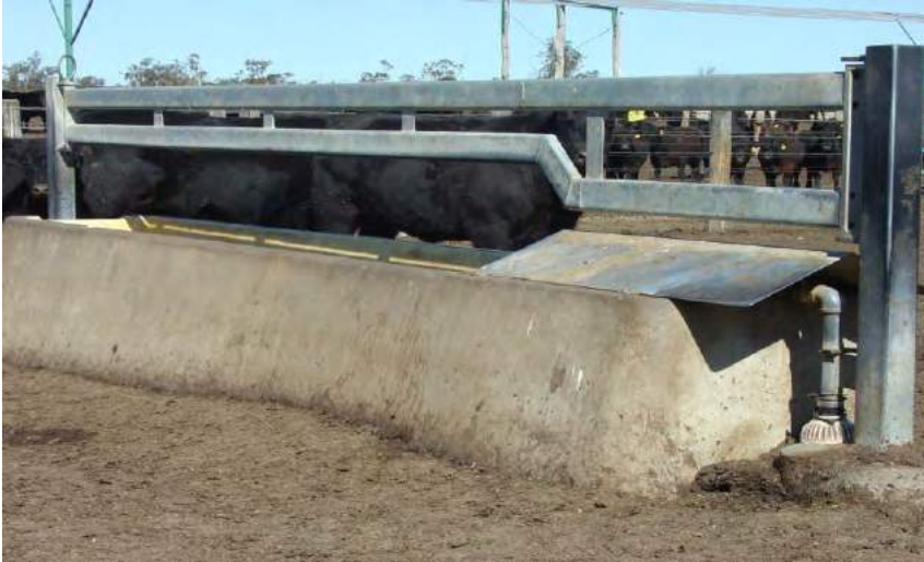
Trapeze-shaped water trough with galvanised float cover, and hinged neck rail to prevent cattle getting into the water trough. A boot cover on water inlet pipe prevents material from entering PVC delivery pipe. (Position E)
