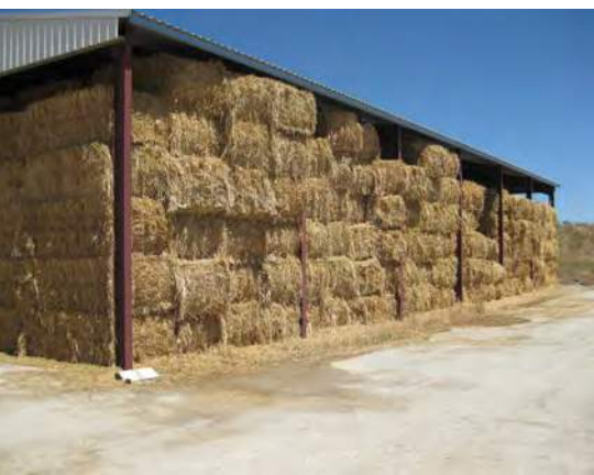
A steel framed, fixed roof open shed. Bales are more likely to be stacked on the stringed side to increase stack stability (as opposed to the unbraced side).
