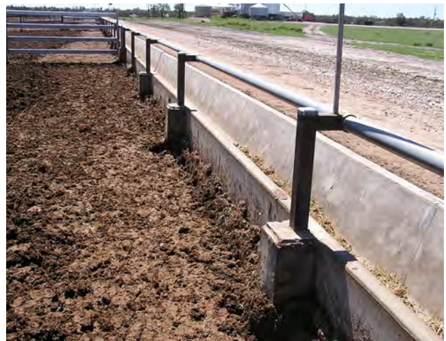
Intruding posts will make apron cleaning difficult.
