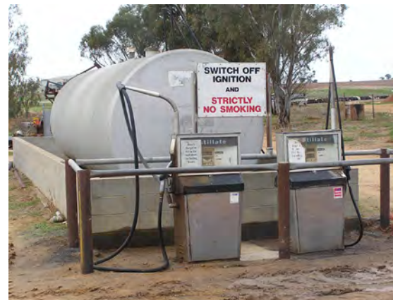
Diesel and petrol fuel storage with bowlers. Bunding behind and to each side of the facility is effective against spills; however it could fill with water after rain and has to be drained.
