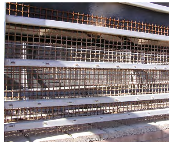
Mesh sheeting on high pressure race offers the operator protection from the animal whilst washing.
