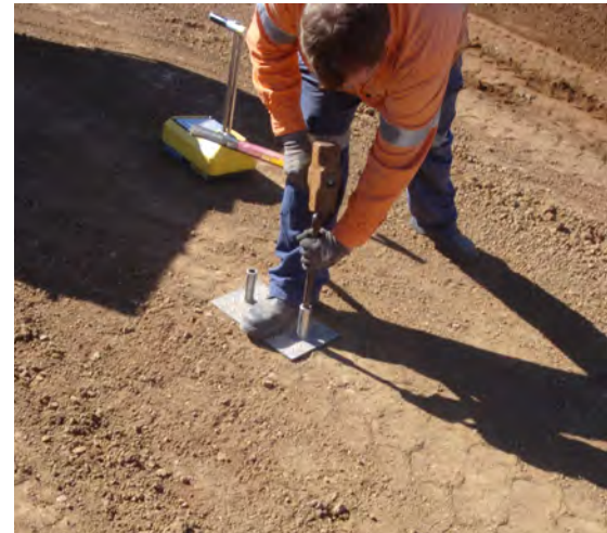
Field testing soil strength
