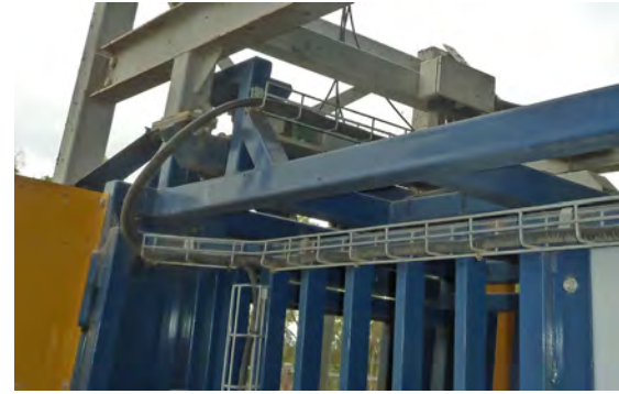
All cabling for control and electronics should be protected from damage.
