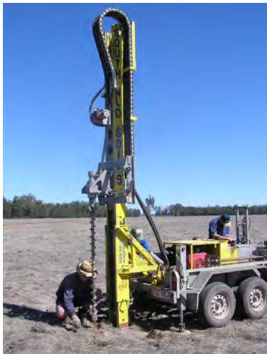
Soil sampling rig using spiral auger
