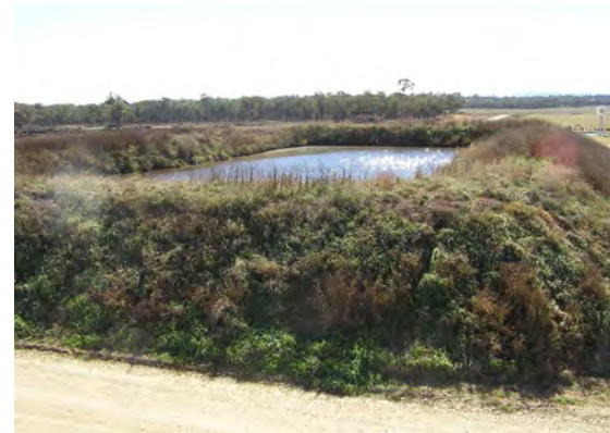
A turkey nest storage situated high above the feedlot allows gravity flow of water around the site.
