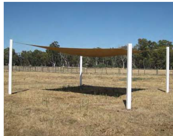
Spelling paddocks with artificial shade – steel posts supporting suspended shade cloth
