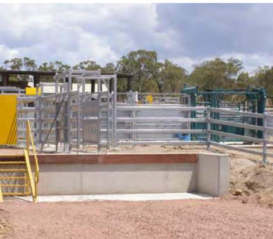
A single deck loading dock
