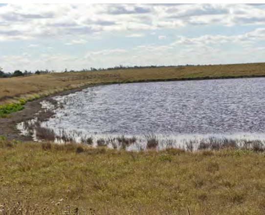
Holding pond with well-grassed batters (to resist erosion) and with sufficient freeboard.
