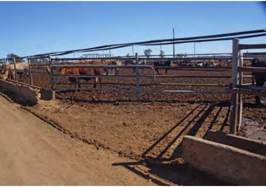
Access gate at the top end of the pens
