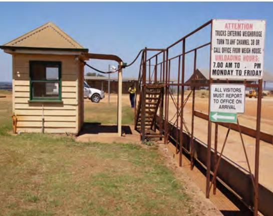
Weighbridge with good signage and a long sampling platform, allowing load to be inspected or sampled without repositioning the trailer.
