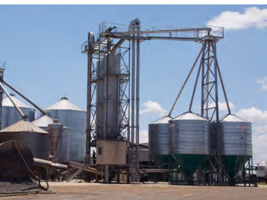
Feeding system – storage, processing and delivery
