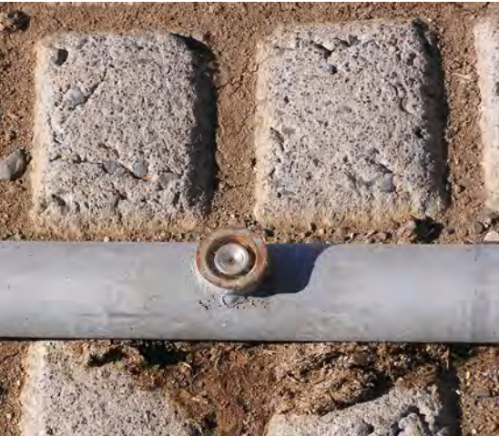
Spray nozzles need protection from the hooves of animals.
