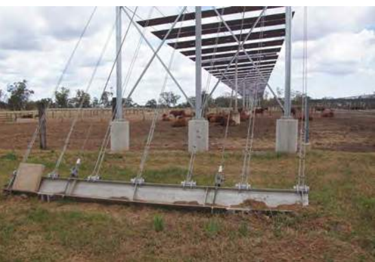
Shading material is often supported on cable suspended between columns, posts or supports. Infrastructure must be engineered for rain, hail and wind loadings.
