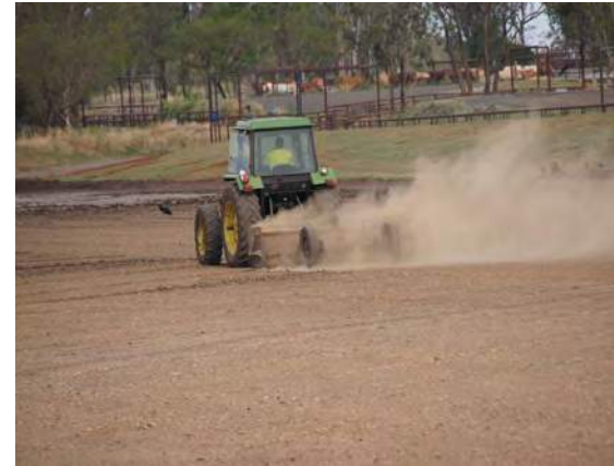
Maintenance of the base of the sedimentation system with a box scraper. Dual sedimentation structures before the holding pond will allow one to be de-silted while runoff is diverted to the other.
