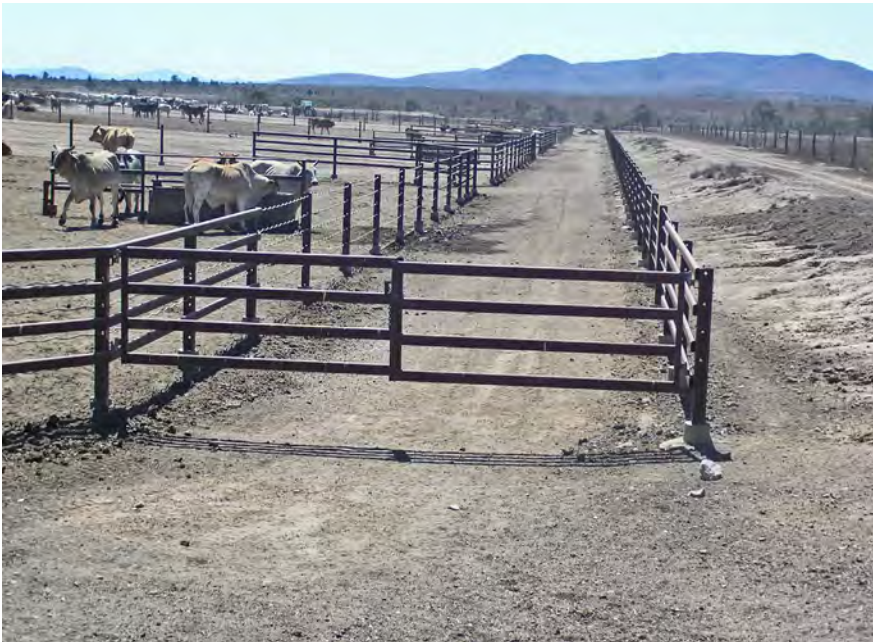
Wide lanes require wide gates. Double gates are preferable when lane width exceeds about 4.5m.
