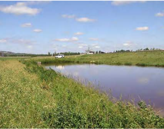
A well-grassed embankment will resist erosion.
