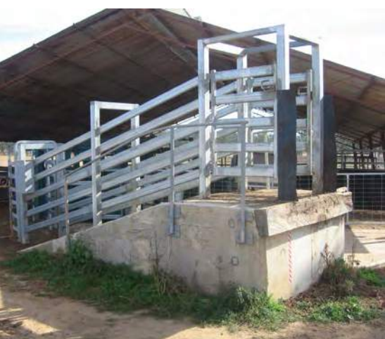
Single deck steel loading ramp
