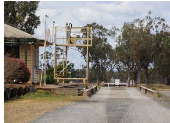
The length of approach will depend on the overall length of the weighbridge. Note proximity to the site office.
