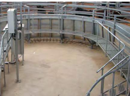
Curved V-race with full inner and outer sheeting and a catwalk with safety handrail.
