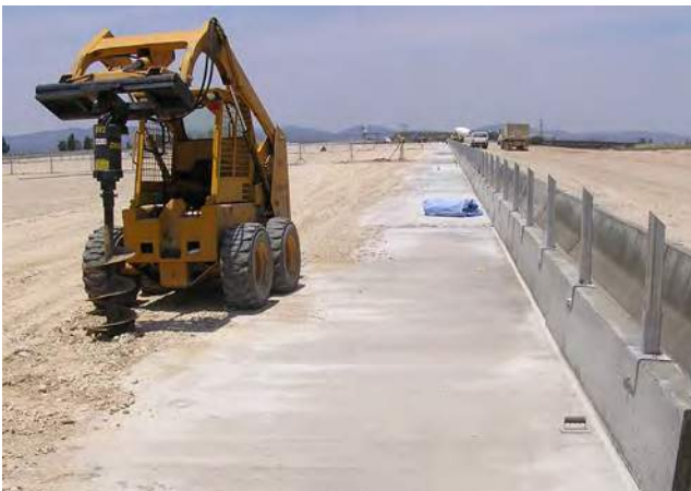
Concrete apron on the pen side of the bunk provides a stable base against mud holes, and allows easy cleaning.
