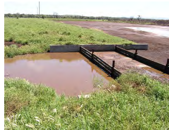
Horizontal timber slat control weir after a storm, with floating material retained in the sedimentation basin.
