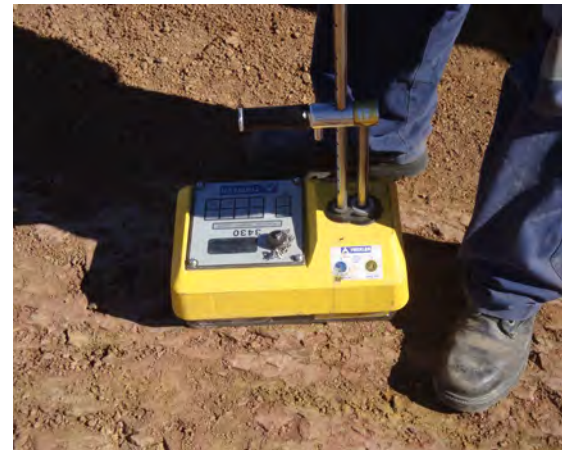
Field testing soil compaction
