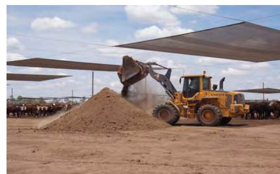
Shade structures should be high enough for machinery. Higher shade structures offer better ventilation but limit the area of shaded footprint and have higher wind loading.
