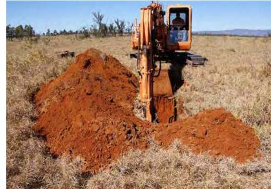
Test pit excavation. Separate the soil horizons or changes in soil texture during excavation to allow soil samples to be collected from each type of material encountered.
