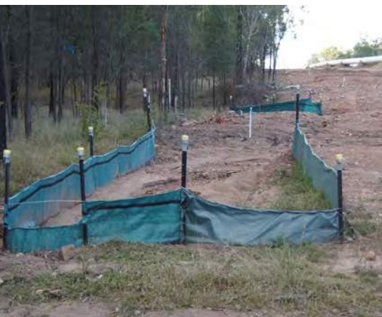
Effective erosion control measures should be installed to protect the working area and newly formed surfaces.
