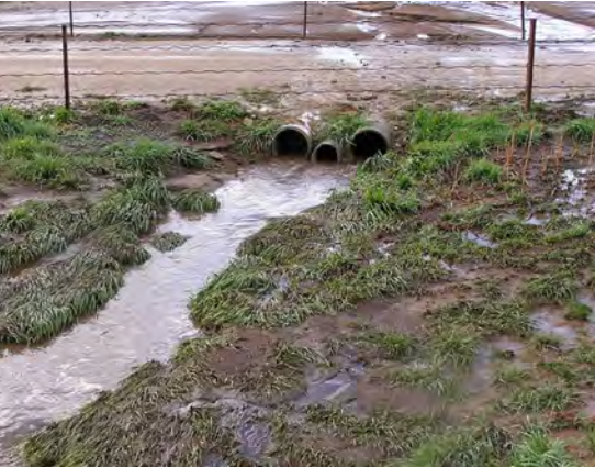
Use the ratio of rainfall to surface runoff (runoff coefficient) to calculate for adequate drainage.
