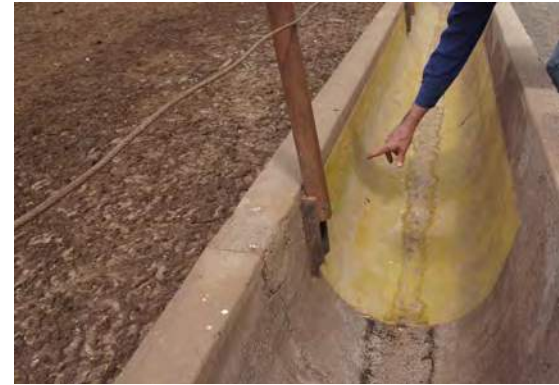
Sealing the inside of the feed bunk with epoxy resin will protect the surface from chemical attack and abrasion.
