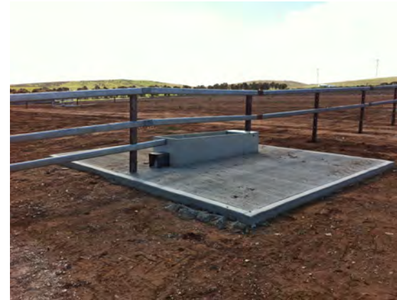
Aprons allow cattle to access to the trough under all weather conditions and allow access for cleaning (Position A).
