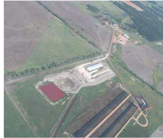
Manure and effluent utilisation area adjacent to a feedlot site.
