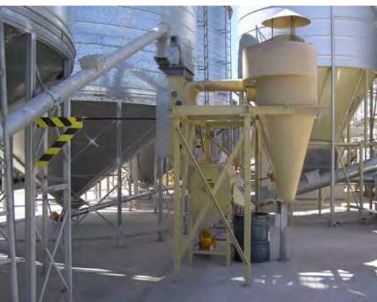
Grain scalper and cyclone to remove unwanted vegetable material and dust.
