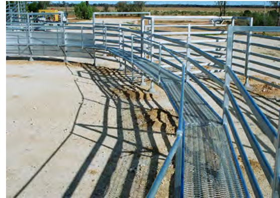
Catwalk on bugle yard
