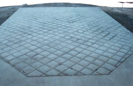
Stamped concrete with continuous square pattern orientated at 45° to cattle flow.
