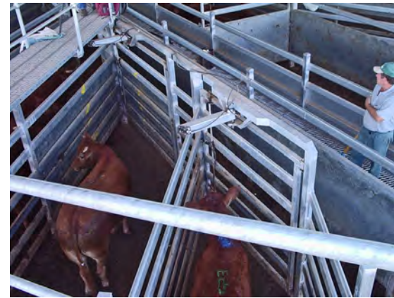
Pneumatically-swing gates used in stacking pens.
