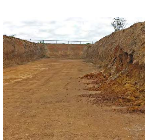
Hillside pit with near vertical walls. Side walls that are too steep may collapse on impact of machinery, or from erosion when empty.
