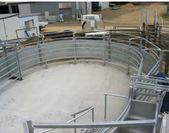
Parallel curved race with no inner sheeting.
