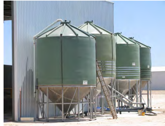
Liquid ingredients can be stored in various types of storage vessels and configurations. These are conical-bottom, HDPE tanks.
