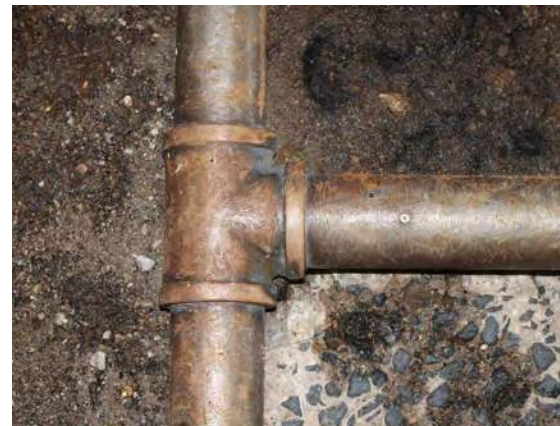
Holes drilled in pipes create a quick and cost effective spray system.
