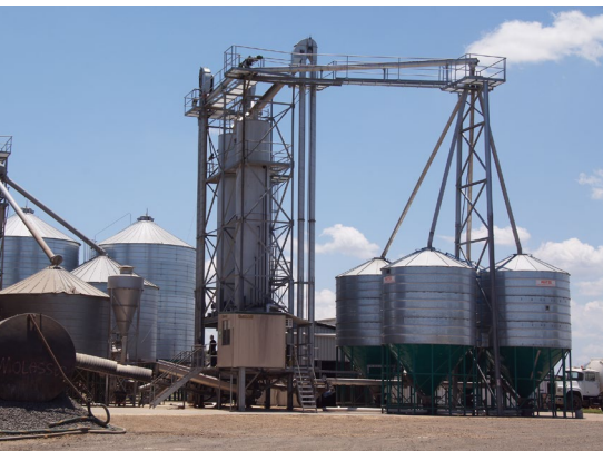
Feeding system – storage, processing and delivery
