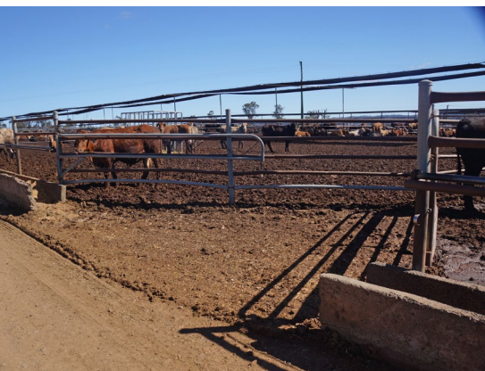
Gates giving vehicle and livestock access to pens from the feed alley
