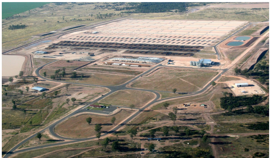
Overall site layout: All vehicles enter from the lower left of the photograph. After going past the office, cattle trucks turn to the left while feed delivery trucks continue straight on.
