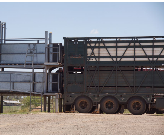
Loading and unloading ramps
