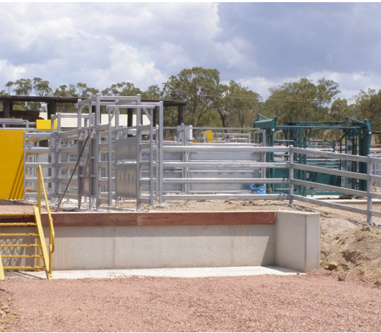
A single deck loading dock
