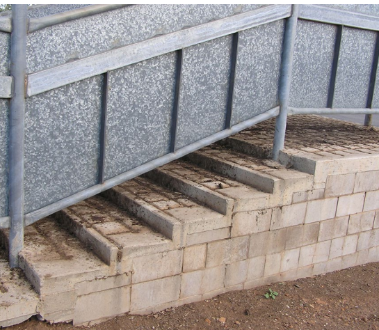
Concrete ramp with steps with pattern stamped into concrete to provide a non-slip surface.
