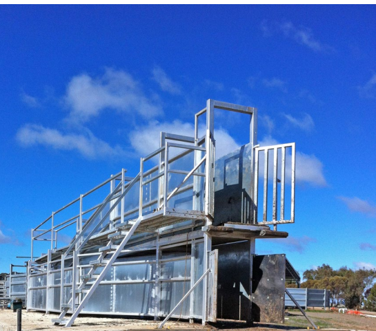
Swing out (batwing) gates and fully sheeted lead-up race and loading ramp.
