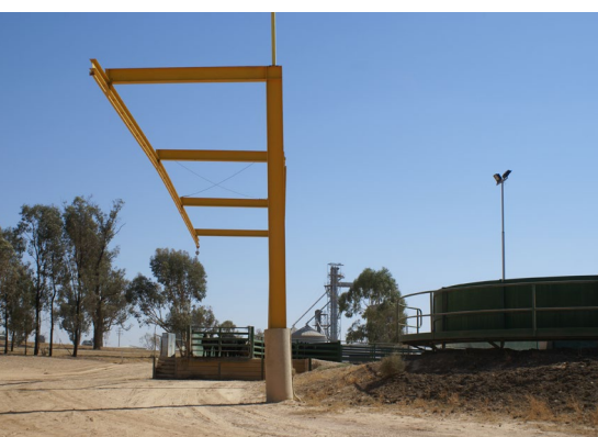
A gantry over parking area for a double deck livestock transport vehicle. Truck drivers would be attached via harness to the gantry for safe working on the top deck of the vehicle
