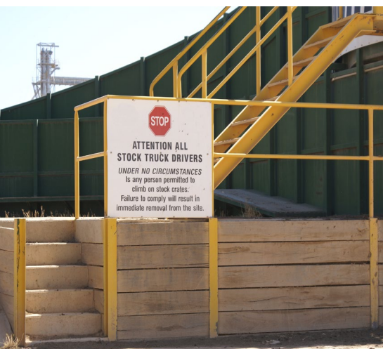
WH&S inclusions on a loading facility sign, with railing and handrails on stairs for operator access
