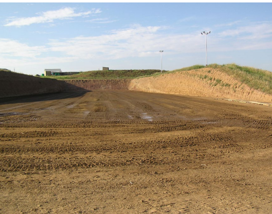
Hillside pits excavated into the side of the slope. The natural slope provides adequate drainage for the open end of the pit.
