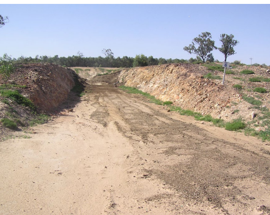
A pit excavated into gently sloping site. Cut soil material has been used to raise height of the embankment, but contains rocks.
