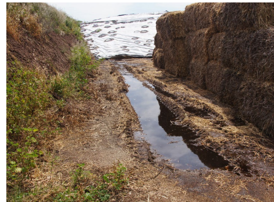
A poorly drained bunker floor allows leachate to remain in the bunker area. The soft floor allows ruts from machinery – exacerbating the problem.
