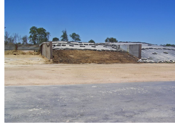
An above ground bunker stack with vertical concrete walls and end wall.
