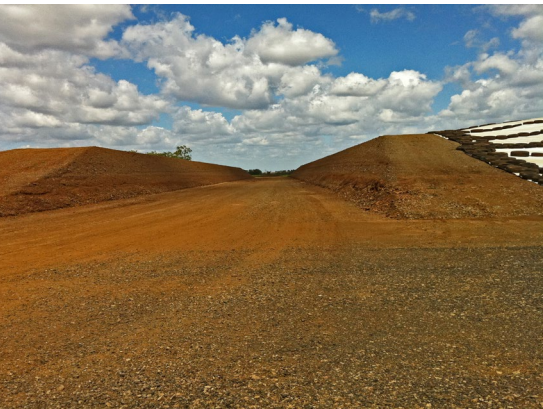
Open-ended, above ground bunker with compacted gravel base and clay walls. The walls are trimmed to the design batter and base to the design grade. A flat sloping end face allows water to drain from top of wall to ground level without eroding the face.
