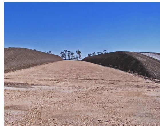
Above ground bunker storage with gravel base and compacted clay walls. The embankments are graded to the end of the storage and the top centres are overlaid with plastic to reduce erosion from stormwater run-off.
