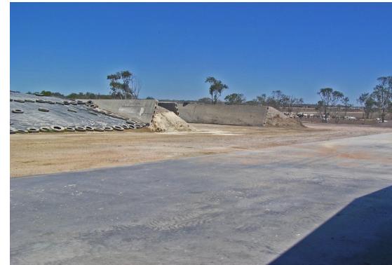
An above ground bunker storage with pre-cast concrete panels laid against the earth embankment. These bunkers are located next to the commodity shed for easy access.
