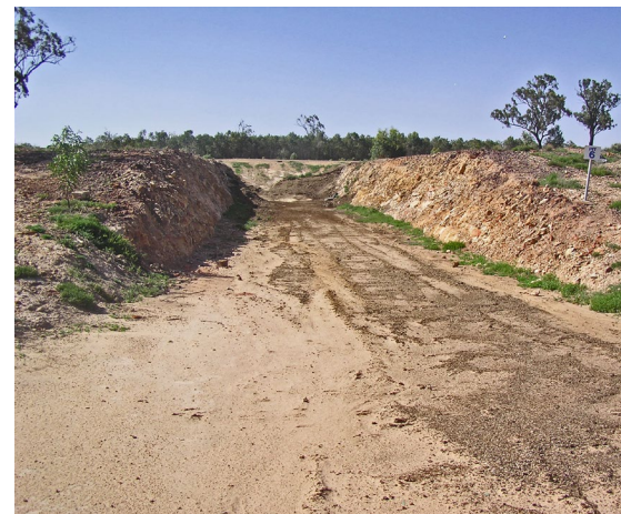
Rocks and tree roots in this earth bunker wall could contaminate silage and damage plastic covers.
