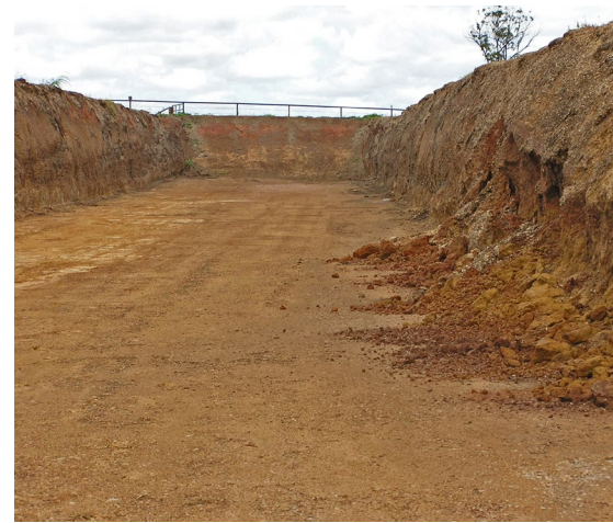
Hillside pit with near vertical walls. Side walls that are too steep may collapse on impact of machinery, or from erosion when empty.
