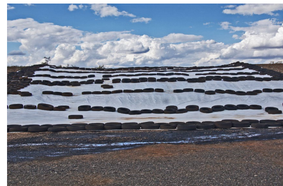
Silage pits should be situated in the CDA so that leachate can be directed and retained in the effluent drainage system.
