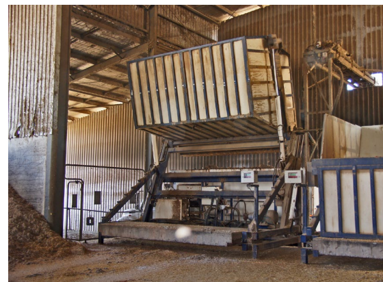
A dual batch-box system installed inside and at the end of the commodity storage.
