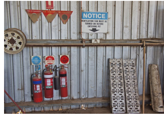
Workshops should have signage and portable fire extinguishers.
