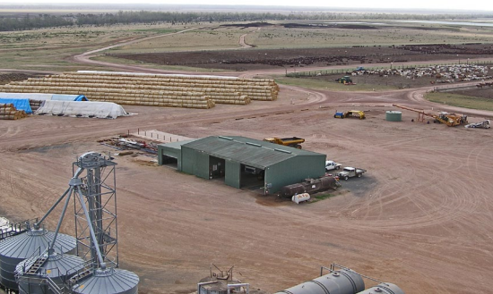
Machinery workshop at large feedlot with drive through design and external storage area for steel.
