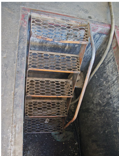
Access to pits should comply with the relevant WHS requirements, with fixed handrails.
