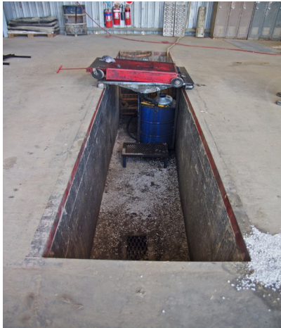
Inspection pit with stairs for access. Pit should have temporary fencing when not in use.
