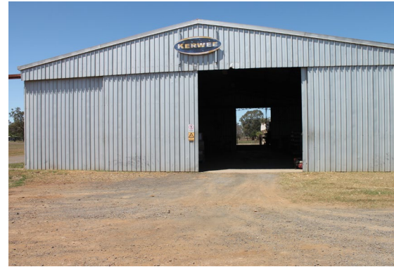
A large machinery workshop with double sliding doors and entry from both ends
