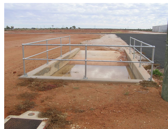
This single trafficable sedimentation basin is adequately sized for cleaning machinery, and has handrails for safety. Wastewater drains to bed level.
