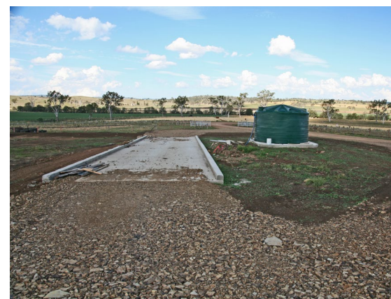
This concrete pad is of suitable length, but too narrow. Water is supplied, but the pad is flat and there is no controlled wastewater drainage system.
