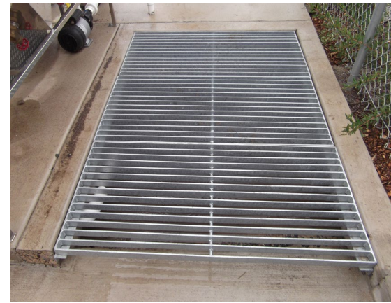
A non-trafficable sedimentation basin grated to prevent access. The heavy grate must be removed to clean out sediment and debris. Not accessible to typical feedlot machinery.
