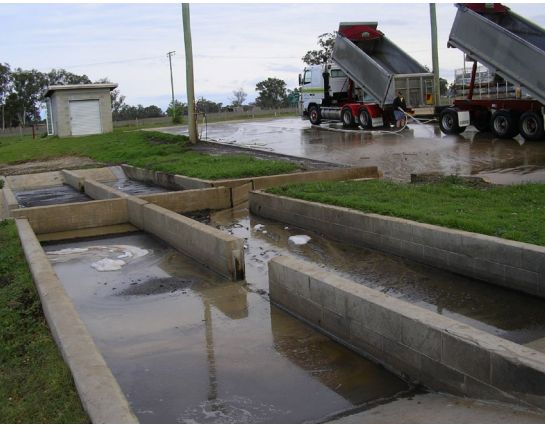
Quadruple trafficable sedimentation basin side by side arrangement. Wastewater is diverted into one or more bays.
