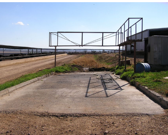
Drive in-reverse out design with platform for elevated access to vehicles. Wastewater drains to feedlot drainage system.
