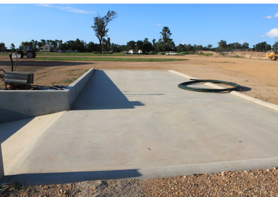
Concrete pad with suitable length and width for most feedlot vehicles, kerbed pad, adequate slope on pad and suitable wastewater collection system.
