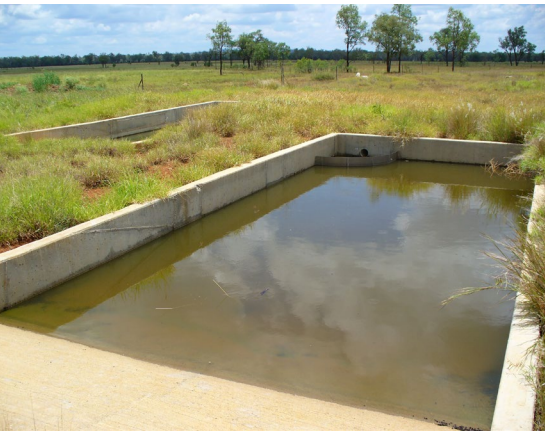
Dual trafficable sedimentation basins allow one to be taken offline to enable sediment to dry. Separate basins cost more than a side by side arrangement. These basins are adequately sized for cleaning machinery but do drain to bed level.
