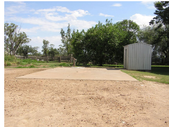
This concrete pad has suitable length and width and equipment storage, but it is flat with no wastewater containment.
