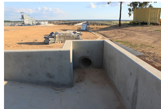
Trafficable sedimentation basin with offset weeping wall/bar screen segment. Wastewater drains to bed level.
