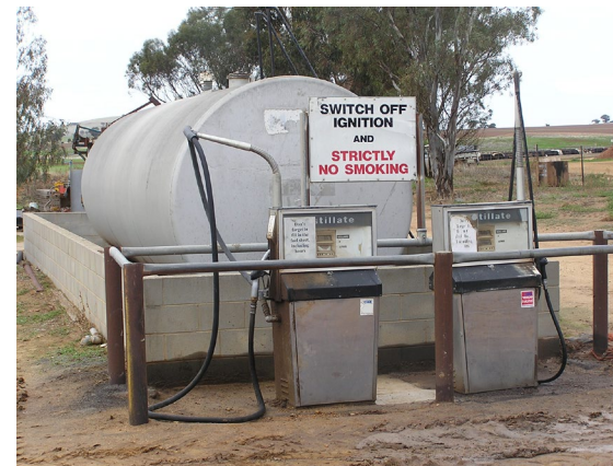
Diesel and petrol fuel storage with bowsers. Bunding behind and to each side of the facility is effective against spills; however it could fill with water after rain and has to be drained.
