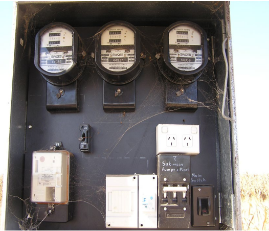
Power authority meters: electromechanical induction-rotating disc meter, with one meter for each phase
