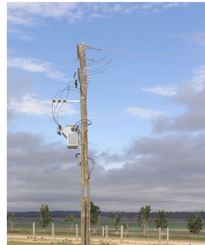
Overhead electricity – supply pole and transformer
