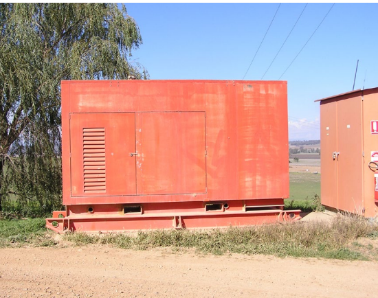
Self-contained backup generator on skid-mount
