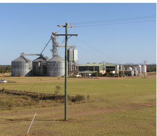
Overhead supply direct to on-site feed processing facility. This is located to avoid accidental contact with high machinery.
