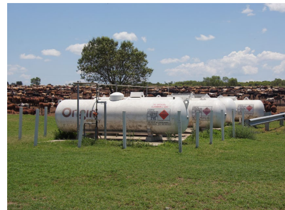
Banked LPG storage tanks – with bollard protection
