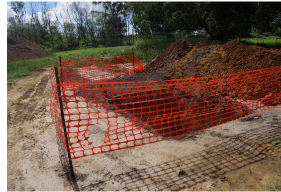
Safety barrier placed around excavated pit
