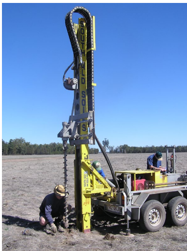
Soil sampling rig using spiral auger
