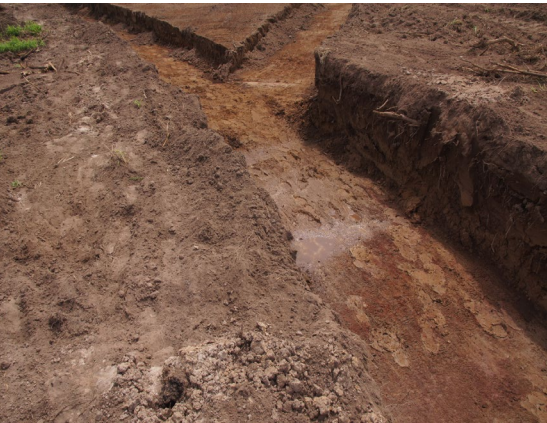
Shallow groundwater intersected during excavation.
