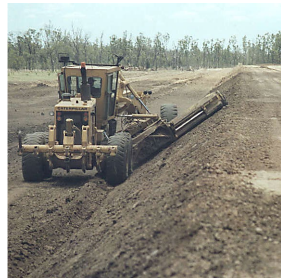
Smoothing embankments with a grader
