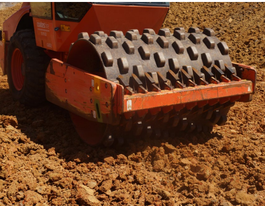
Soil fill in earthworks must be compacted. This sheepfoot compactor combines high speed and capacity compaction control.
