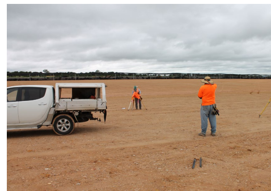
Step 1. Setting out earthworks
