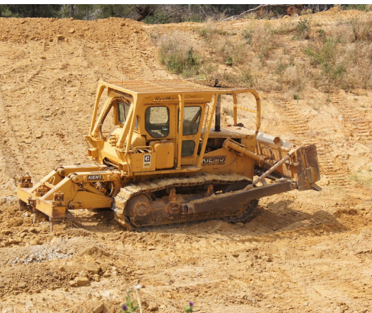
Bulk earthworks start with dozers...
