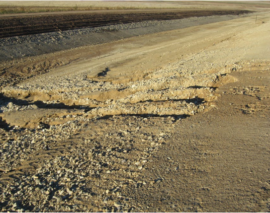
Effective erosion control measures should be installed to protect the working area and newly formed surfaces.
