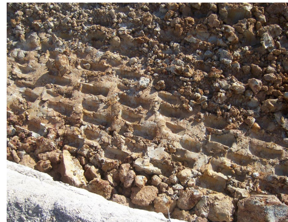
Optimum moisture level of soil permits a strong cast formed from sheep's foot roller compaction.
