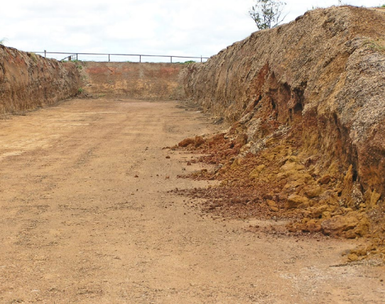
Batters that are too steep for the soil type and strength will collapse.
