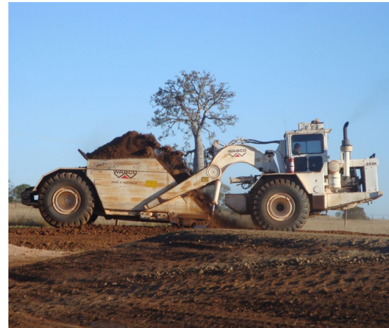
Step 3. Removing topsoil
