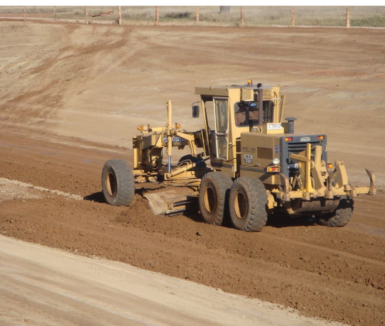
Graders are used for excavation, batters and precision finishing in the final shaping of surfaces (e.g. roads, pens, building foundations).
