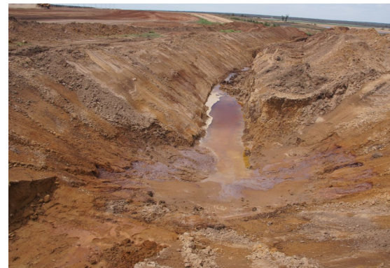
Problems may arise during construction earthworks. Groundwater encountered will need appropriate drainage.
