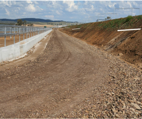
Acceptable limits for cut and fill slopes depend on soil type and strength, geology of the site and saturation.
