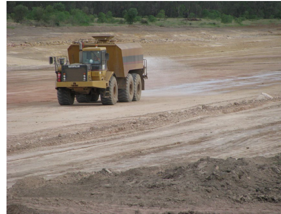
Dry surfaces may need spraying with water to allow the required degree of compaction.
