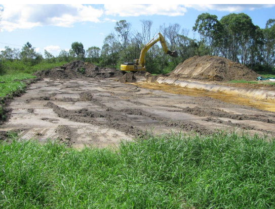
Step 2. Clearing vegetation
