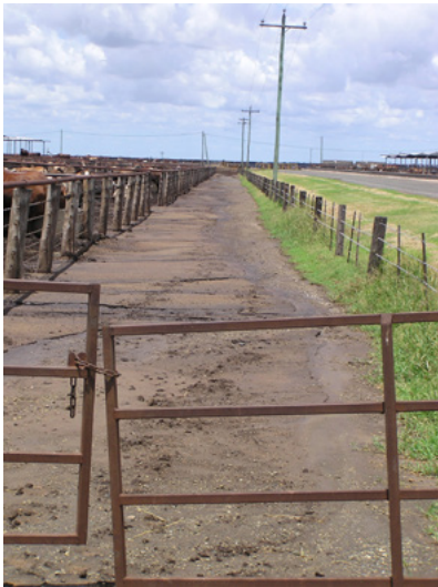
Drains below the pens direct runoff to the holding pond and need to be kept clean.
