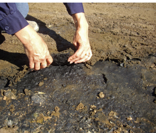
Manure interface layer over compacted gravel base
