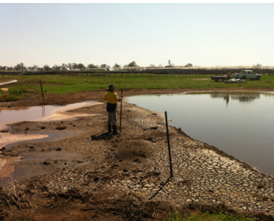
Solids that accumulate in the holding pond over time need to be removed eventually.
