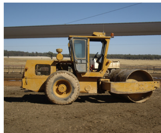
Newly placed gravel under shade being compacted with roller.
