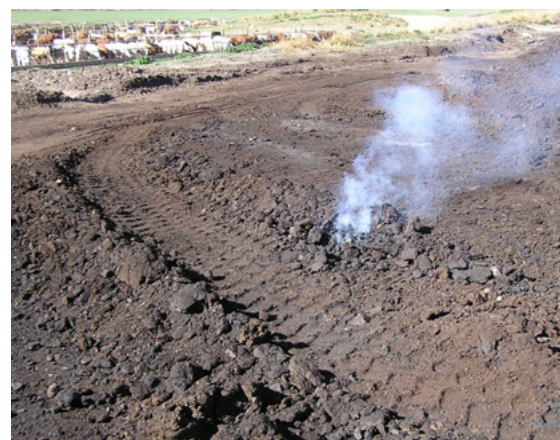
Unsuitable moisture content can lead to spontaneous combustion. Stockpile fires are difficult to extinguish.
