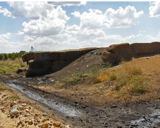
Runoff and leachate from the mortality composting area must be controlled.
