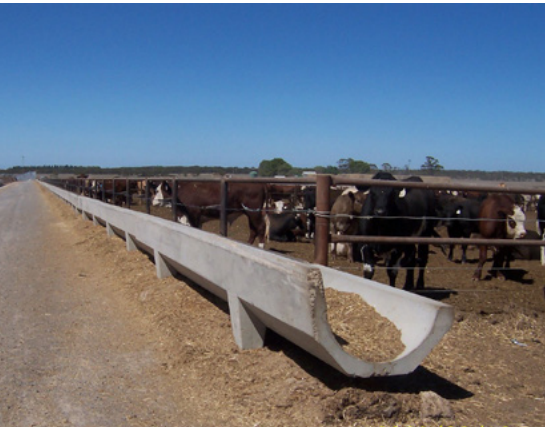
Spilt feed should be collected and taken to the manure storage or composting area.
