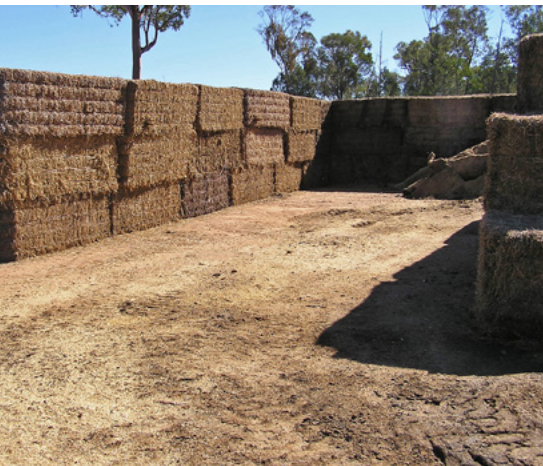
Areas for composting mortalities need a well-compacted base.
