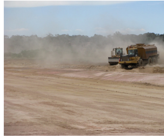
Good pen foundations help to reduce problems of odour or dust.
