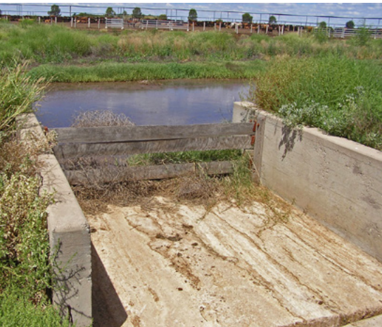
Vegetation growing into sedimentation basins and holding ponds provides a site for flies to breed.
