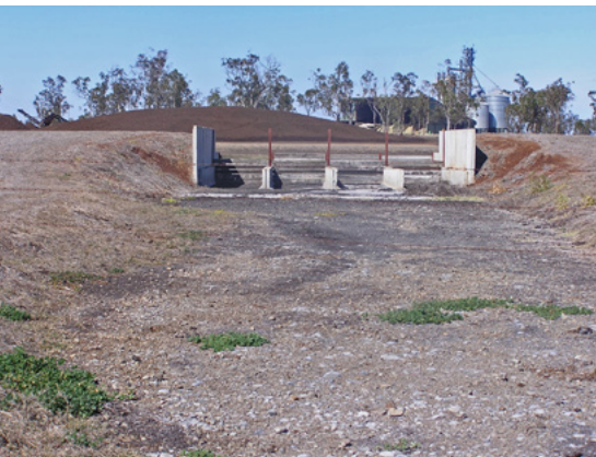
A weir filters effluent runoff and allows solids to settle in a sedimentation basin.
