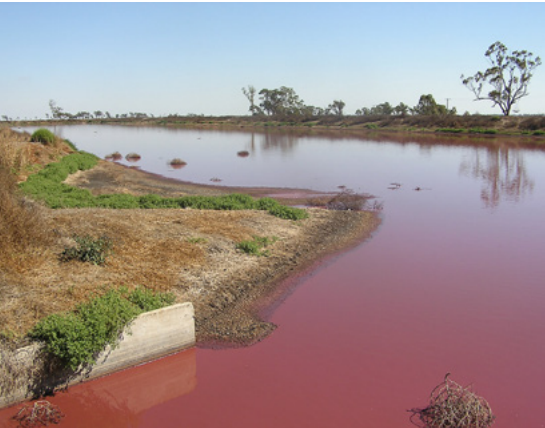
A holding pond retains effluent until it evaporates or can be used for irrigation.
