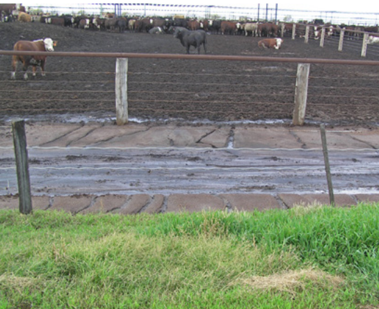
Drains direct runoff into a sedimentation system or holding pond.
