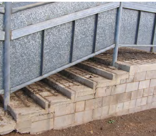
Concrete ramp with steps with pattern stamped into concrete to provide a non-slip surface.
