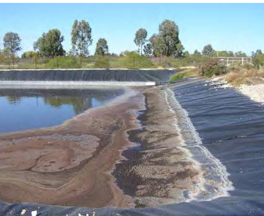
Synthetic liner to minimise water seepage
