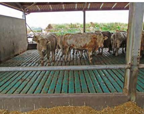
Parallel slatted flooring
