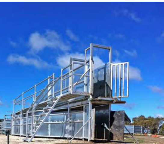
Swing out (batwing) gates and fully sheeted lead-up race and loading ramp.
