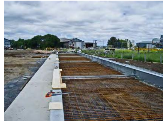
Weighbridge platform construction – concrete platform and reinforcing mesh needs to be well connected to the main lateral beams to prevent buckling.
