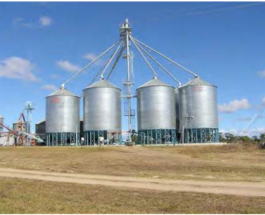
Gravity fall of grain through tubes from the bucket elevator to cone-bottom silos using a diverter. Greater height of bucket elevator is required for gravity fall of grain.
