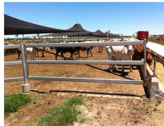
A gate in the pen fence line across the feed bunk apron allows easy access by pen cleaning and maintenance equipment, and by pen riders. Gates require a strainer assembly for support.
