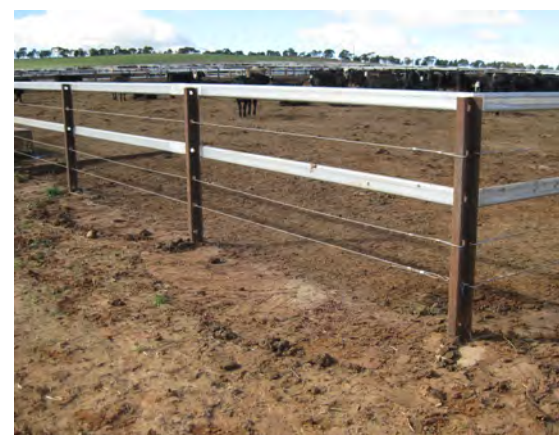
Steel top and belly rails with cables
