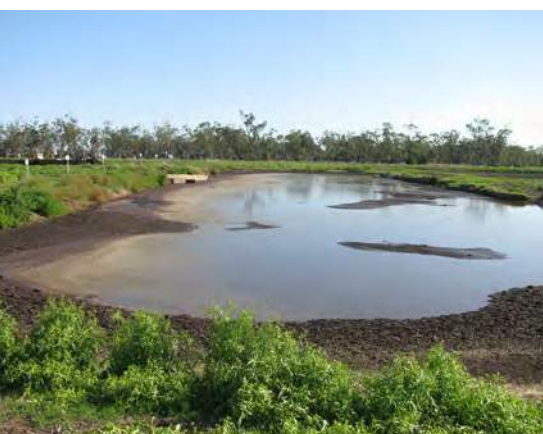
A sedimentation pond (5 m deep) that stays full of liquid. This pond has an inlet weir for incoming sediment and effluent runoff, and an outlet weir to a shallow, large surface area evaporation basin.
