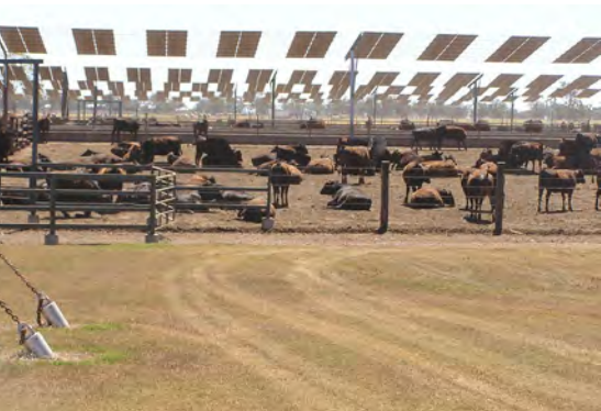
With galvanised iron sheets in hotter climates a pitch of 1:3 increases air movement and shade coverage in the afternoon.
