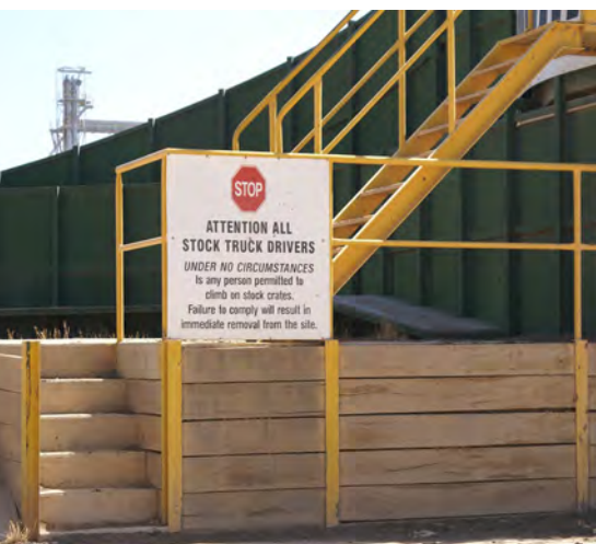
WH&S inclusions on a loading facility sign, with railing and handrails on stairs for operator access
