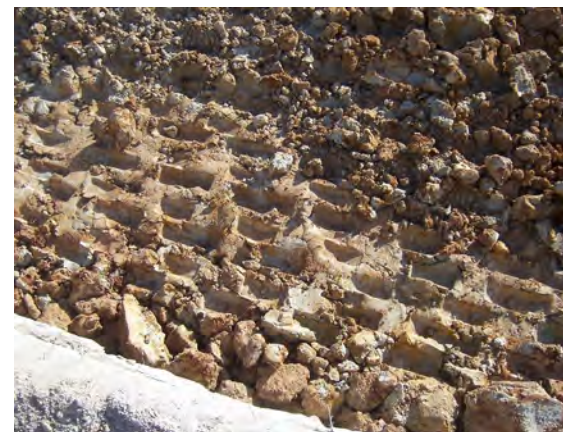
Optimum moisture level of soil permits a strong cast formed from sheep's foot roller compaction.
