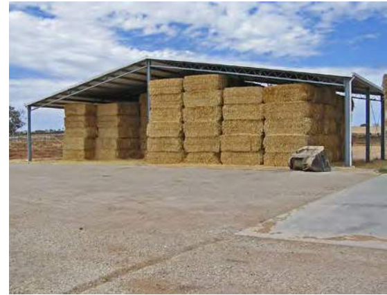
The large span of a steel framed, fixed roof open shed provides unrestricted access. Downpipes take roof water away from the storage area.
