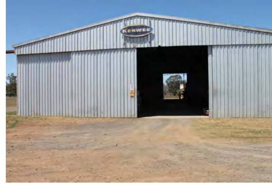
A large machinery workshop with double sliding doors and entry from both ends
