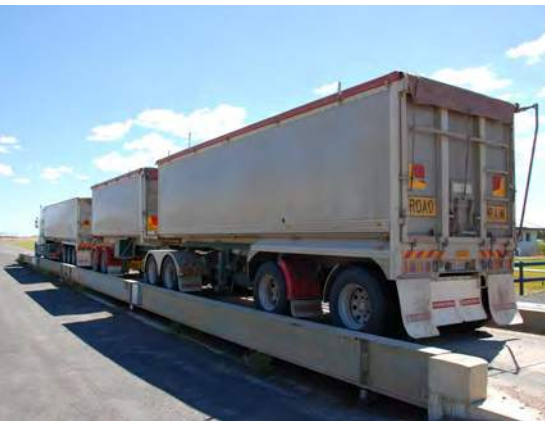
A multiple deck weighbridge allows the truck to be weighed in a single measurement.
