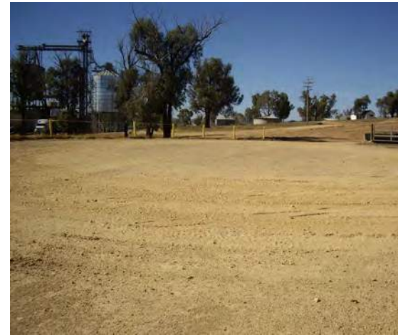
Even grading material on turnaround results in little displacement of coarse material.
