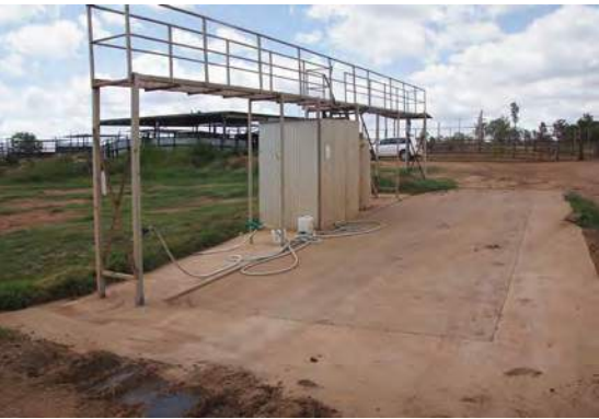
Drive-through design with platform along full length of washdown pad. Wastewater drains to feedlot drainage system.
