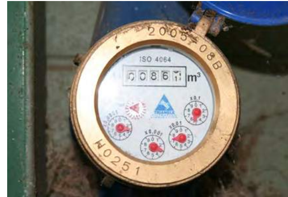
Flow meters may have analogue or digital display. Digital meters can have data loggers.
