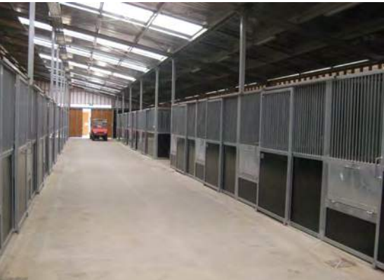
The aisle between two rows of stalls should be at least 3m wide.
