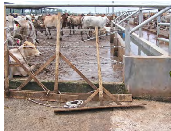
A water trough placed across the bottom fence will prevent proper pen drainage – a poor design choice.
