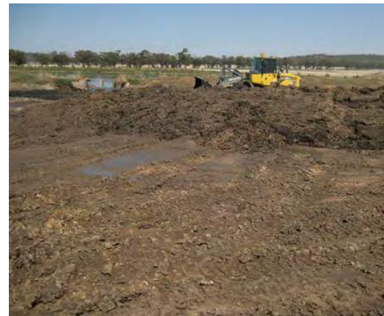
Cleaning out a sedimentation basin in relatively wet conditions is not desirable as wet sludge is difficult to handle, store and will not dry out.
