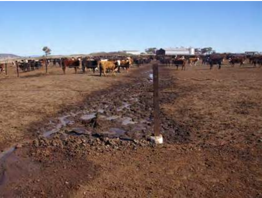
Pen to pen drainage is not desirable. Here a row of pens runs up the slope towards the feed mill with little cross slope. Runoff and manure flows through all pens before exiting at the lower end. This runoff is from a leaking water trough in a pen in the middle of the row.
