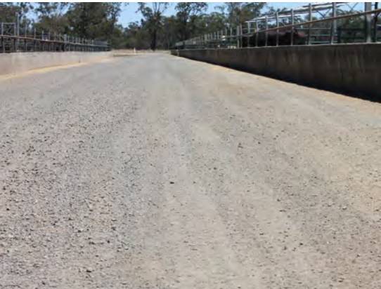
Road constructed from even grading material—well maintained by regular cleaning and grading.
