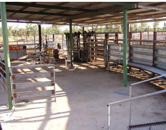
Steel and timber roof over crush, race and handler working area only.
