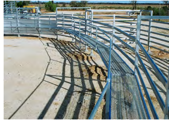
Catwalk on bugle yard
