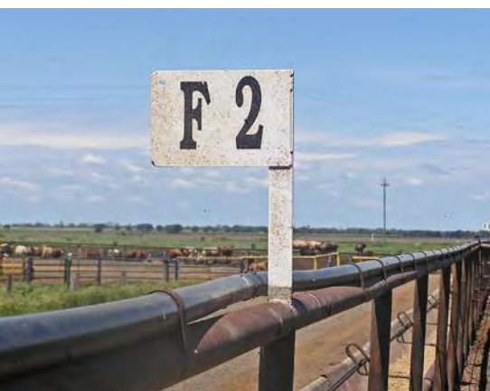
Polyethylene water pipeline attached to top rail of fence will allow water to heat up during hot weather and is not recommended.
