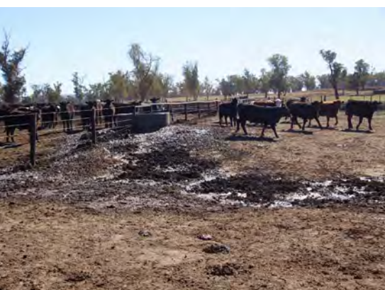
Leaking water troughs create wet spots in pens and should be fixed as soon as possible. A sewer system would have prevented this problem.
