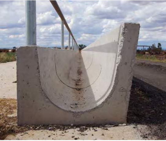
Feed Bunk type H cast in situ.
