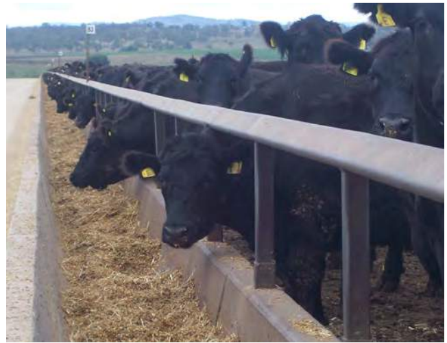
Single steel bar cattle restraint with posts cast into the back wall of the feed bunk
