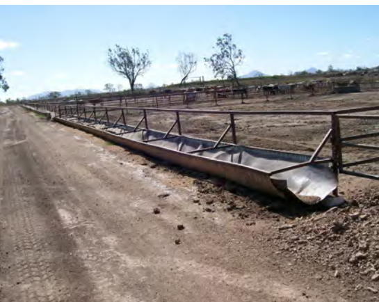
Bunk of corrugated steel half-pipe inside which rubber belting has been subsequently laid. Same issues as above.
