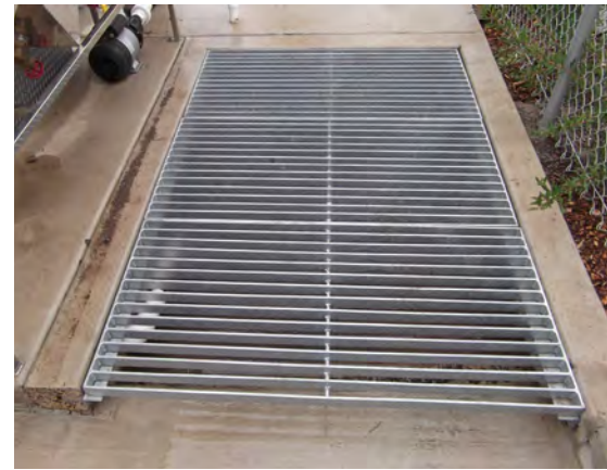
A non-trafficable sedimentation basin grated to prevent access. The heavy grate must be removed to clean out sediment and debris. Not accessible to typical feedlot machinery.
