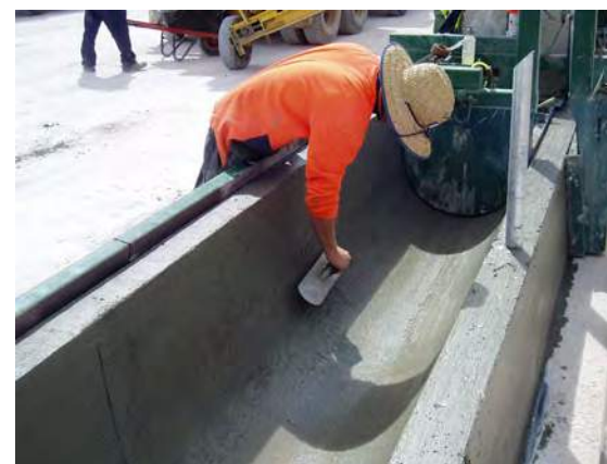
Feed Bunk G. The slip-form machine runs on prefixed rails, then the surface is steel trowelled.
