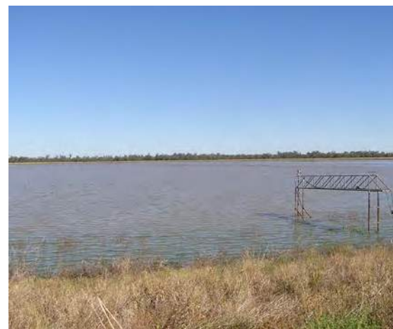
Land surface diversions need off-stream storages. Losses from evaporation and seepage can be large.
