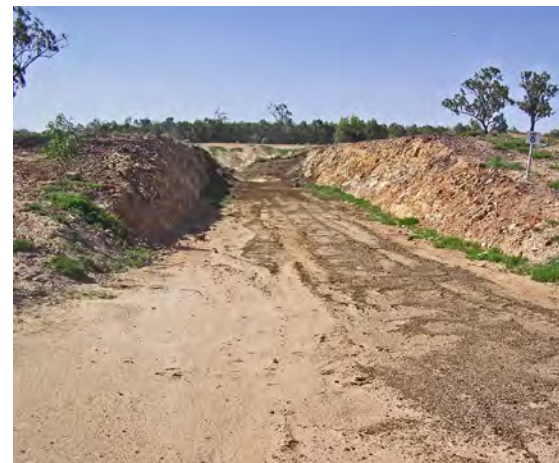
Rocks and tree roots in this earth bunker wall could contaminate silage and damage plastic covers.
