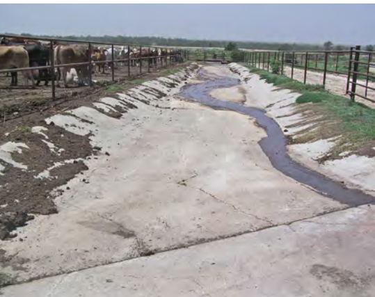
Concrete drains can be used in steep drain sections to prevent erosion. However, the drain must be wide enough to allow access by cleaning equipment.
