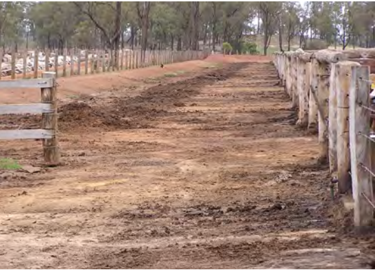
Cattle lane and catch drain – Option 1. The cattle lane is not fenced allowing free access by drain cleaning and under-fence pushing equipment. However, extra stockmen may be needed to move cattle.
