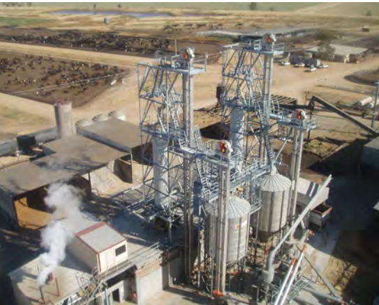
Large feed mill and commodity storage.
