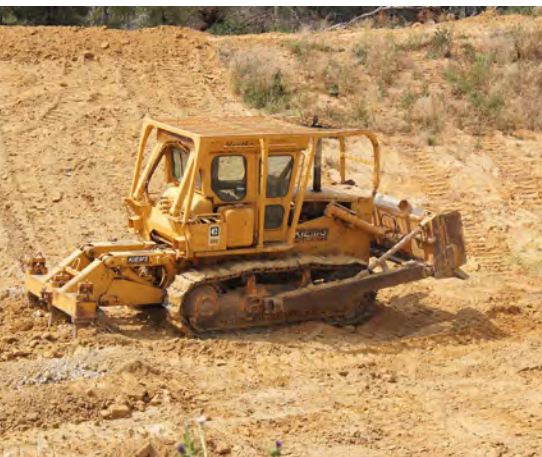
Bulk earthworks start with dozers...
