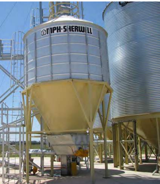
Live bottoms on cone-bottom silos provide a wider opening for handling products, such as moist grain, that tend to bridge.
