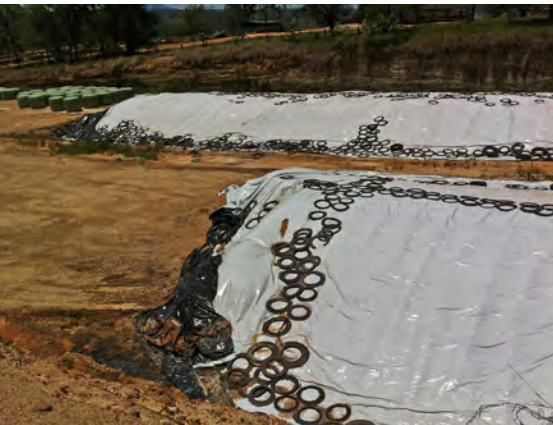
An above ground stack with no side walls. Note stack lay out on compacted earthen pad.
