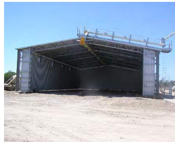
Grain can be temporarily stored under cover. This grain storage shed has a permanently mounted central discharge auger for loading the shed.
