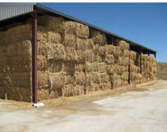
A steel framed, fixed roof open shed. Bales are more likely to be stacked on the stringed side to increase stack stability (as opposed to the unbraced side).
