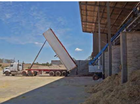
Sufficient space for easy access and tipping for large trucks and semi-trailers.
