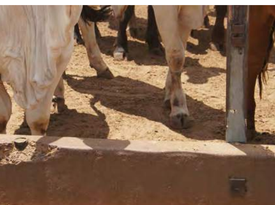
A rusted or broken post has been replaced with a new post bolted to the back of the wall.
