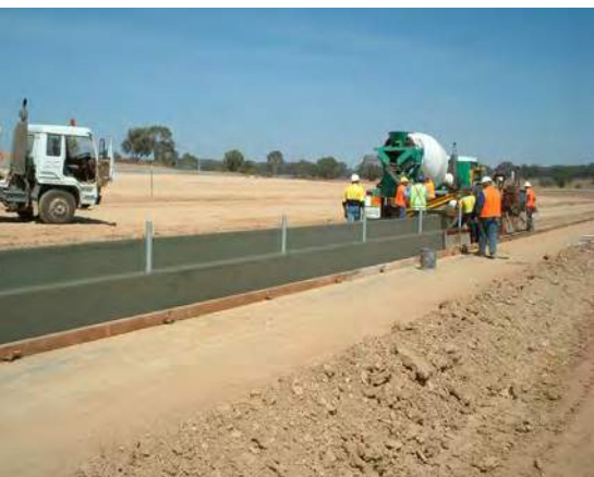
Finished concrete surface of feed bunk should be sprayed with curing oil immediately to minimise shrinkage and cracking.
