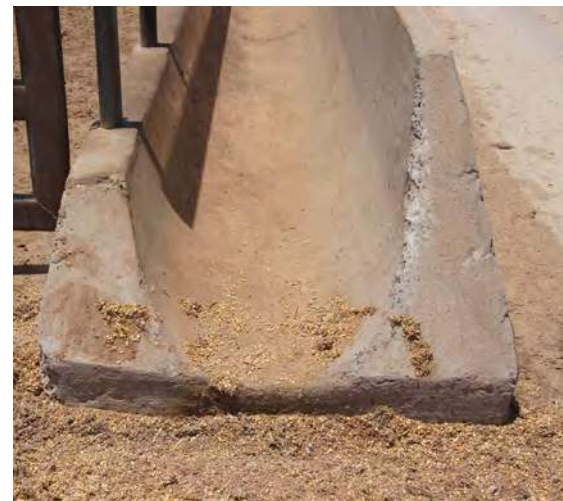
Feed Bunk Type G on concrete apron. Front wall slopes towards the pen.
