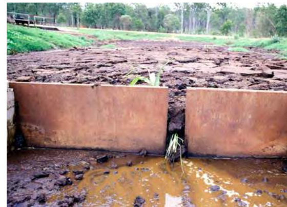
A vertical slot weir used in a sedimentation terrace
