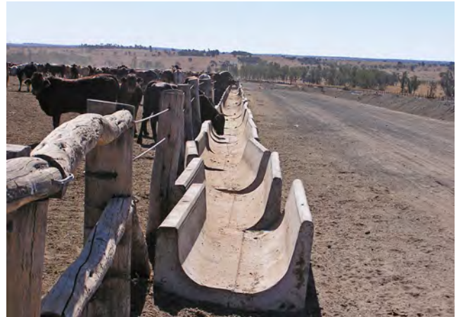
Without suitable anchoring, pre-cast bunk sections can be moved out of alignment.
