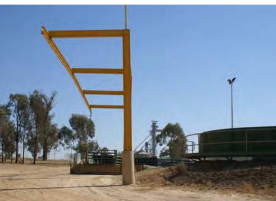
A gantry over parking area for a double deck livestock transport vehicle. Truck drivers would be attached via harness to the gantry for safe working on the top deck of the vehicle
