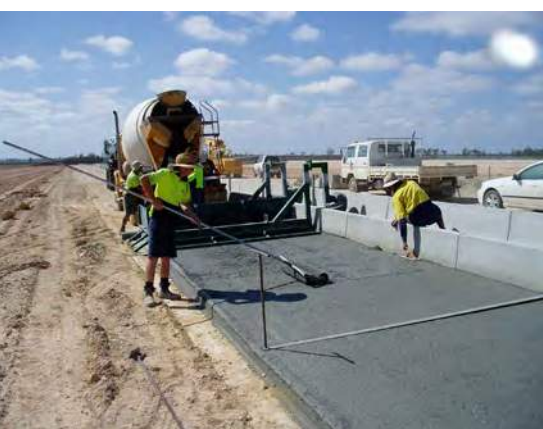
... for concrete works
