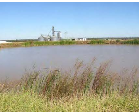
Uncovered turkey nest storage near a feedmill
