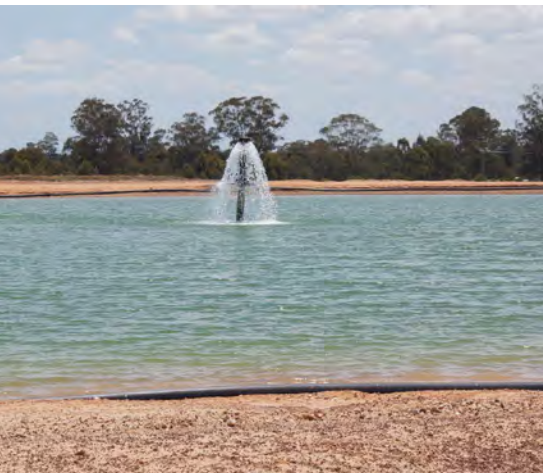
Fountains help aerate and cool artesian water and/or storage water during hot weather.
