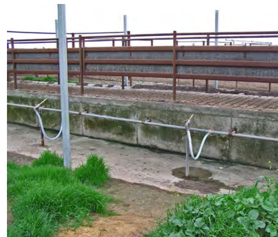
Short hoses from multiple takeoff points are easier to handle than a single long hose. Note the tap on the nozzle for flow control.
