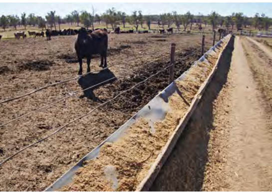
Feed trough made from rubber belting is difficult to clean internally and externally. Manure and spilt feed promote odour, flies and vermin.
