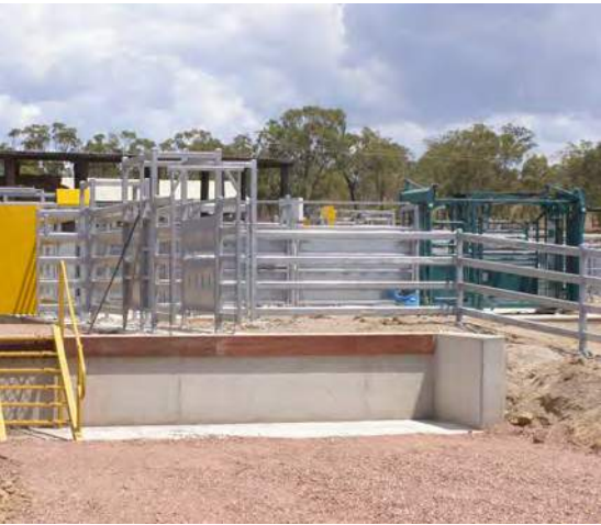
A single deck loading dock
