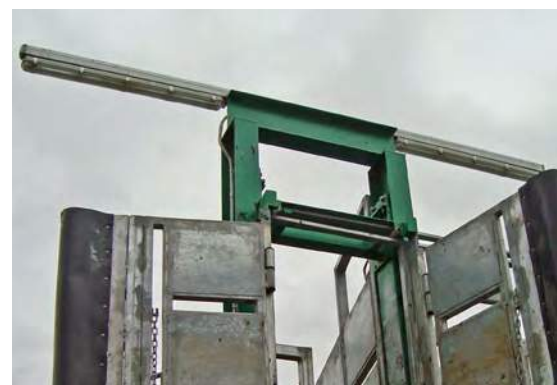
Fluorescent strip lights installed over loading ramp for night loading
