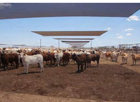
Shade structures – separate panels
