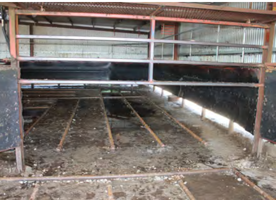
Overhead gates are safer and more practical than hinged gates for operators in confined areas, but are more expensive to construct and require mechanical assistance to operate.
