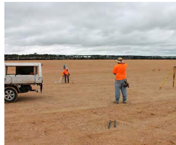
Setting out of works for a new feedlot site
