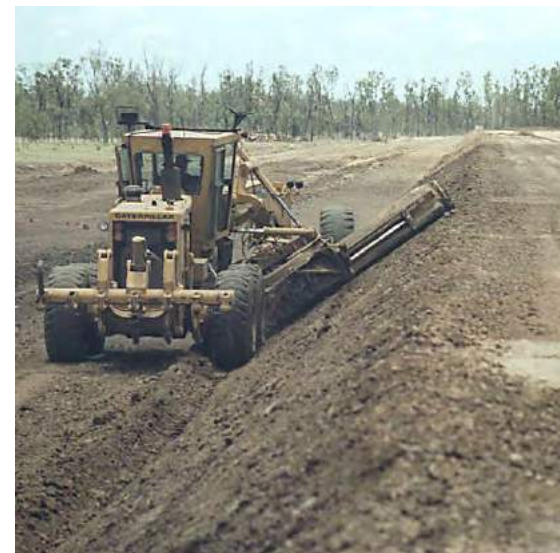
Smoothing embankments with a grader
