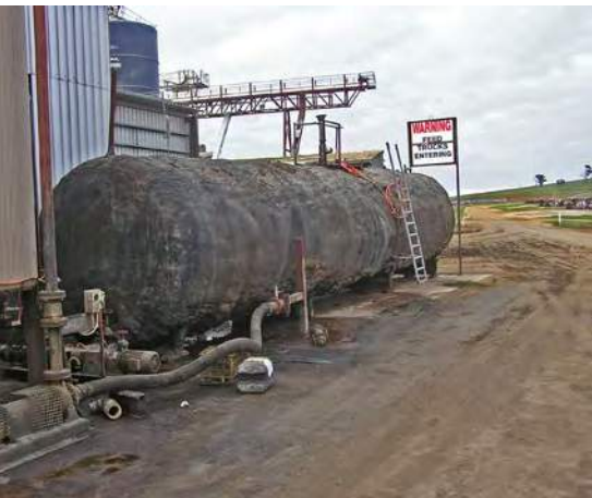
Insulation may be required for those liquids that thicken in low temperatures.
