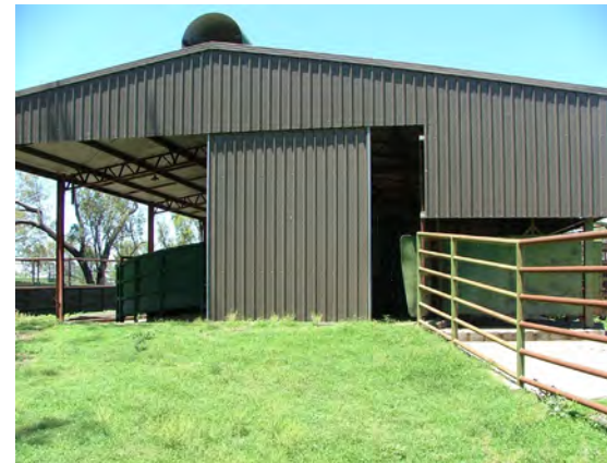
Steel frame building over the entire processing area. It is partially enclosed for protection against rain and wind, with a roof vent for ventilation.
