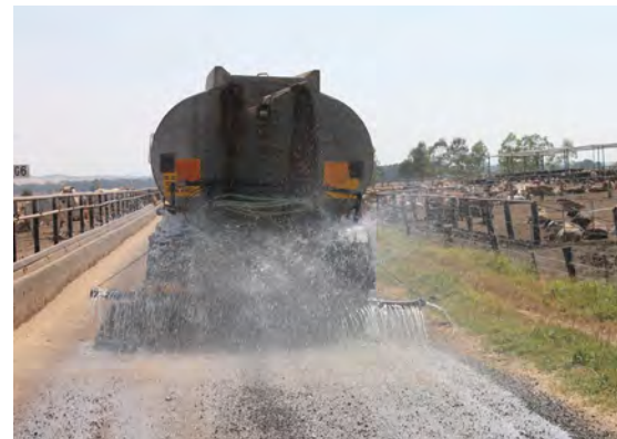
Watering roads will maintain surface integrity, reduce corrugations and reduce dust.
