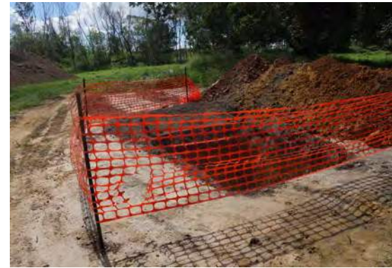
Safety barrier placed around excavated pit
