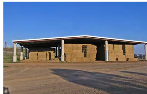
Fixed solid roof, supported by concrete encased steel columns
