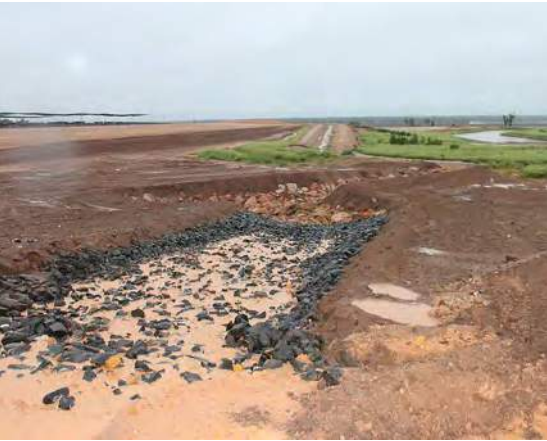
Erosion and sediment controls should be implemented downstream of working areas to prevent off-site impacts.
