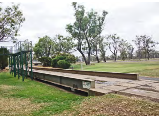
Above-ground truck weighbridge with commodity sampling platform.
