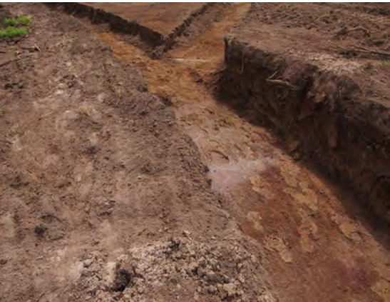
Shallow groundwater intersected during excavation.
