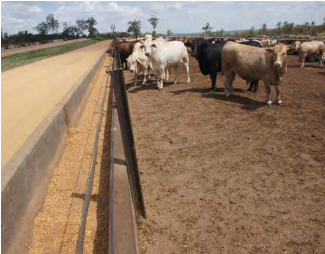
External posts of old cheap railway line will inhibit cleaning along the feed apron and lead to damaged posts and bunks.
