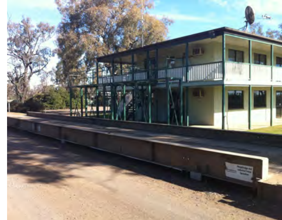
Permanent office and employee amenities building with adjacent weighbridge.
