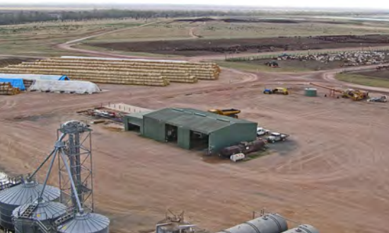
Machinery workshop at large feedlot with drive through design and external storage area for steel.
