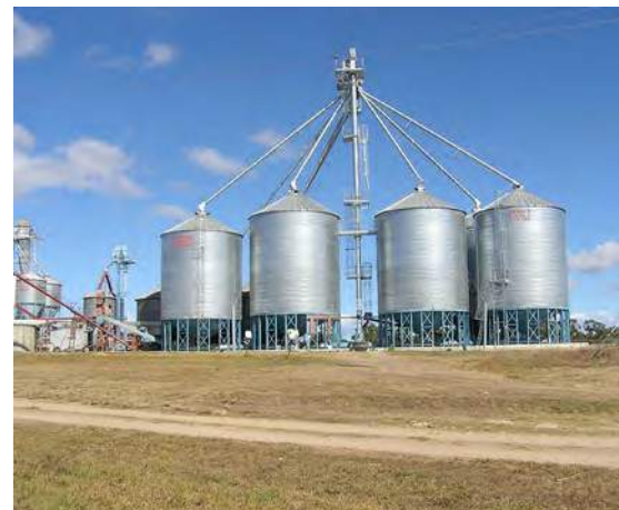
On-site grain storage facility.
