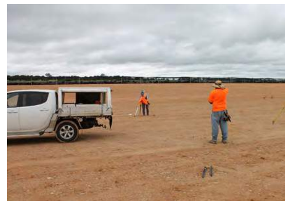
Step 1. Setting out earthworks
