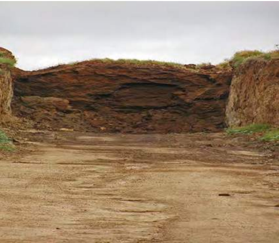
A hillside pit with near vertical walls and covered with soil. The soil type here provides a stable and durable side wall – which may not always be the case.
