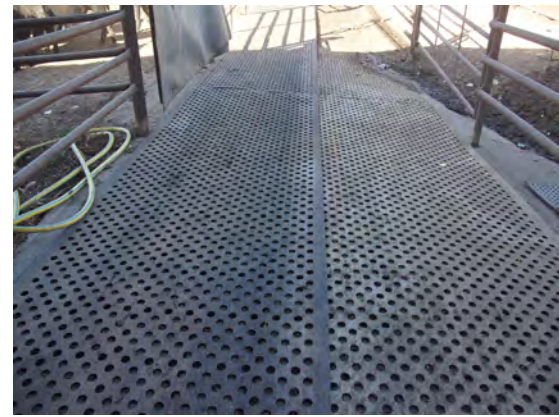
Rubber soft-flooring in handling areas.
