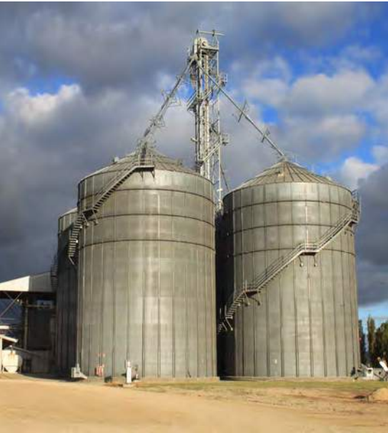
Large-capacity flat-bottomed silos. Note safety handrails are included on the walkway.
