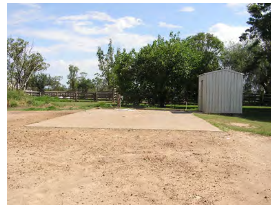
This concrete pad has suitable length and width and equipment storage, but it is flat with no wastewater containment.
