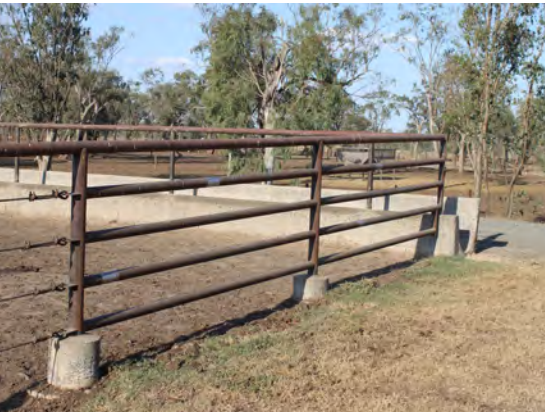
Steel pipe is probably the most common material for fence line posts. Concrete 'post pots' reduce corrosion and also damage by pen cleaning equipment.
