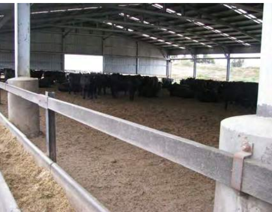
Gable, trussed roof with sheeted end wall
