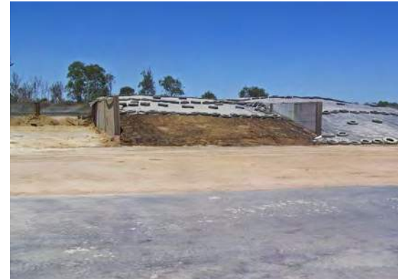
An above ground bunker stack with vertical concrete walls and end wall.
