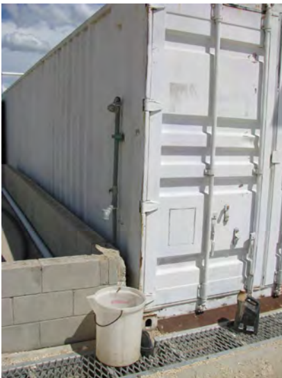
Shipping containers make an excellent storage facility for chemicals. Note the drain at the front of the container and shower on the left.
