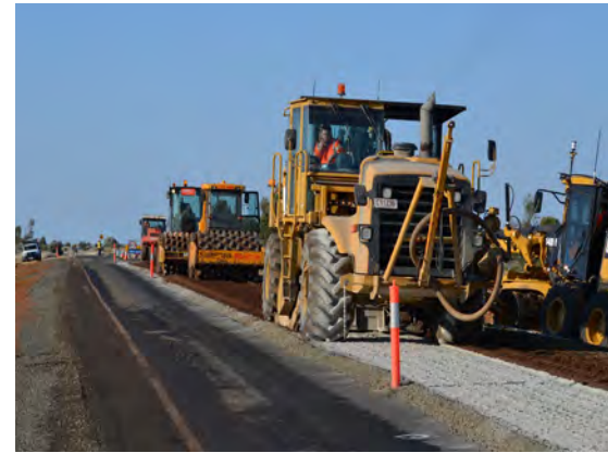
Stabiliser machine mixing binder agent into road base material. The mixed material is being compacted immediately by the sheepsfoot compacters.
