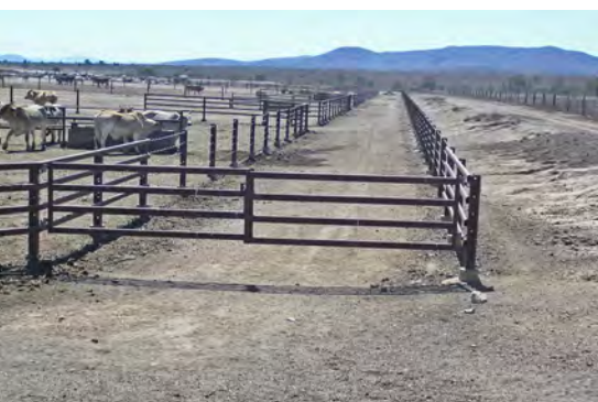
Gates at the top end of a cattle lane allow access for pen cleaning equipment and manure trucks
