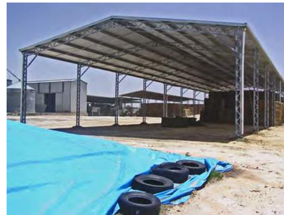
Fixed roof, open sheds vary in structural design and geometry.
