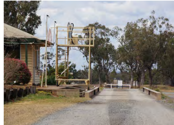
The length of approach will depend on the overall length of the weighbridge. Note proximity to the site office.
