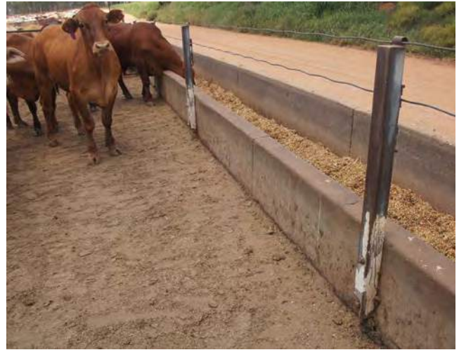
Posts bolted behind the back wall are more readily replaced but can hinder cleaning along the feed apron.
