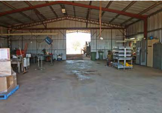
Workshop with space for vehicle and machinery repairs, and with fluorescent and halogen strips for good lighting. Note the wall mounted swing-away jib boom for welder on the left.
