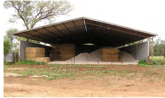
Storage structures for dry feed commodities should be closed or covered to protect the contents from the weather.
