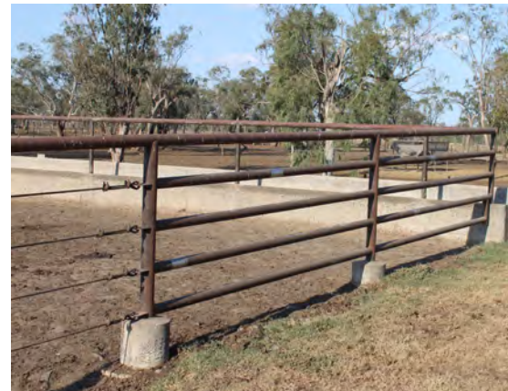
Strainer panels or end assemblies are required at the end of each length of fencing.
