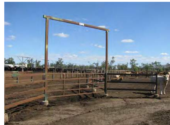
Strainer assemblies across gate openings provide structural stability for both the gateway and cable tension.
