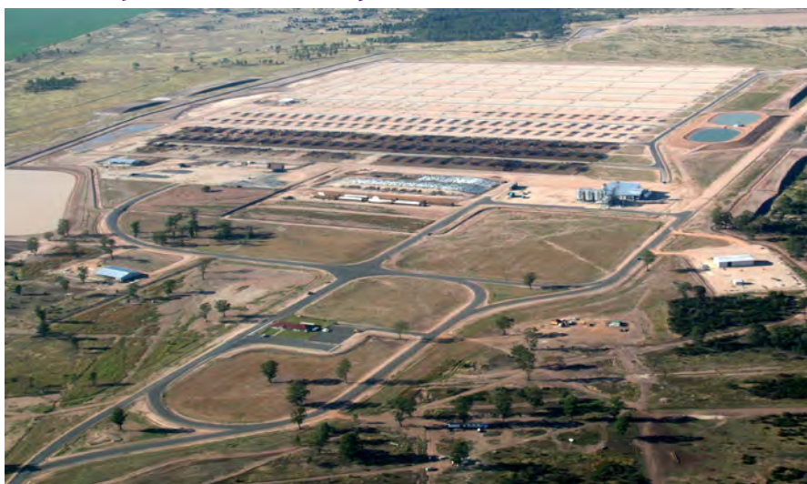
Overall site layout: All vehicles enter from the lower left of the photograph. After going past the office, cattle trucks turn to the left while feed delivery trucks continue straight on.
