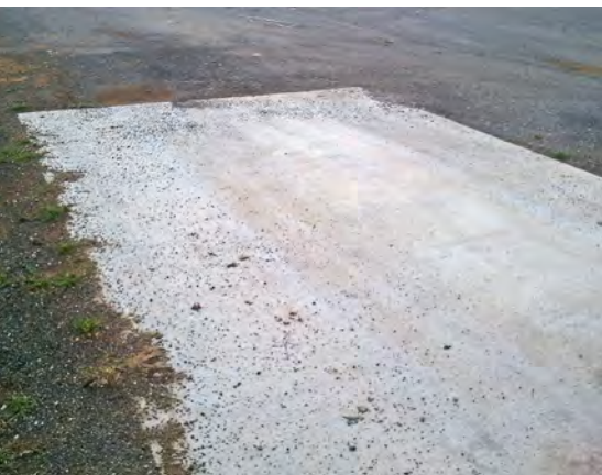
Concrete hardstand in front of loading ramp
