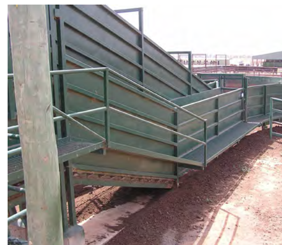
Personnel catwalk along side of the loading ramp.
