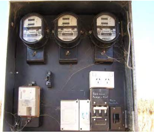
Power authority meters: electromechanical induction-rotating disc meter, with one meter for each phase
