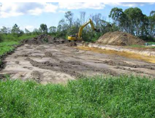
Step 2. Clearing vegetation
