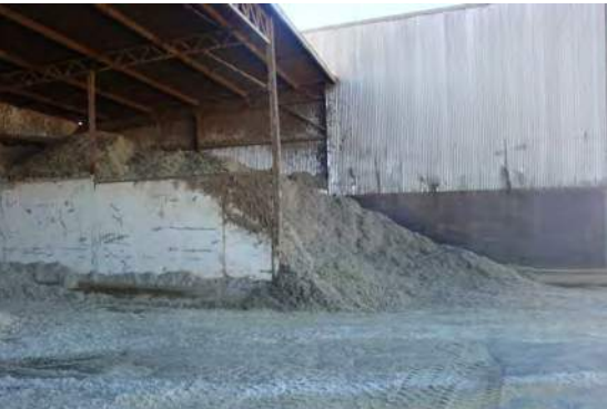
The volume of individual bays should be designed to cater for the volume of delivery vehicles so that all material can be stored under cover.
