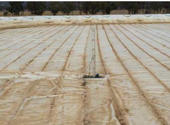
Covering emergency water storages helps reduce water evaporation and prevent access by wildlife and pests.
