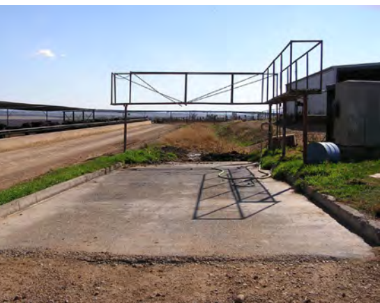
Drive in-reverse out design with platform for elevated access to vehicles. Wastewater drains to feedlot drainage system.
