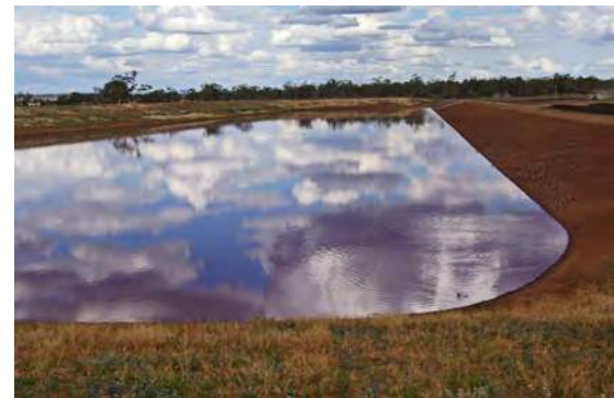
Well-maintained embankment batters with sufficient freeboard
