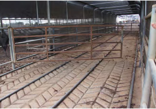
Gates provide access for cattle and equipment; hinged or overhead sliding gates are commonly used in a cattle wash.
