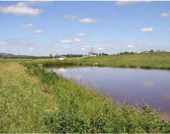
A well-grassed embankment will resist erosion.
