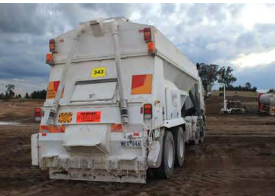
Spreader truck used for spreading dry binder agent onto base material.
