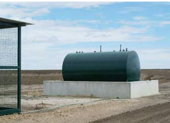
Diesel tank with a good paint coating, free from rust and damage. A more reflective colour (silver or white) would be preferable.
