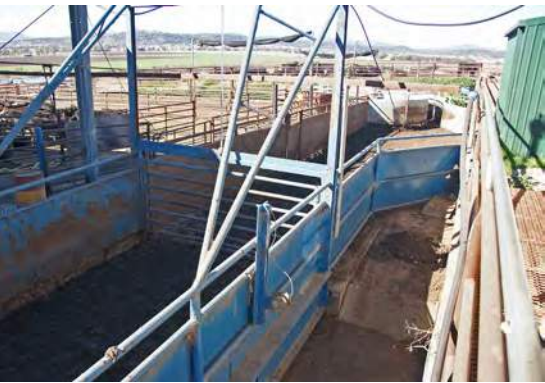
Weighbridge for standing cattle.
