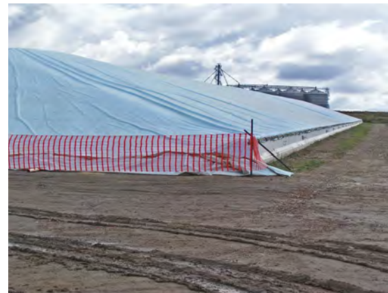
Temporary grain stockpile in a bunker storage with pre-fabricated steel sides.
