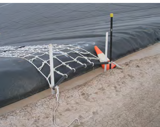
Rope nets are an important safety feature in synthetic-lined storages to allow escape if people or animals fall in the storage.
