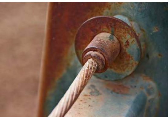
Cable tension control using a wedge-lock system that was developed in the construction of pre-stressed concrete.
