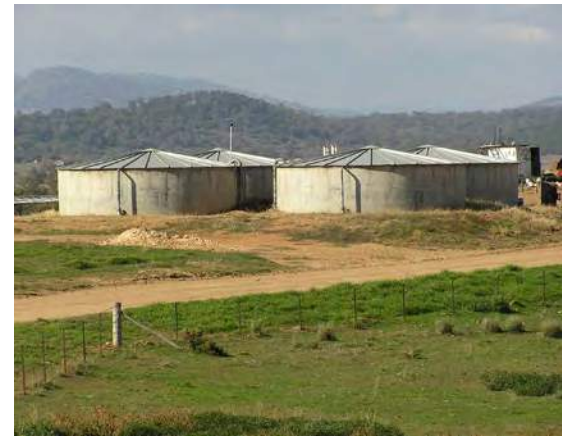
Concrete water storage tanks of various capacities may be cast in-situ. Most have concrete or galvanised iron roofs.
