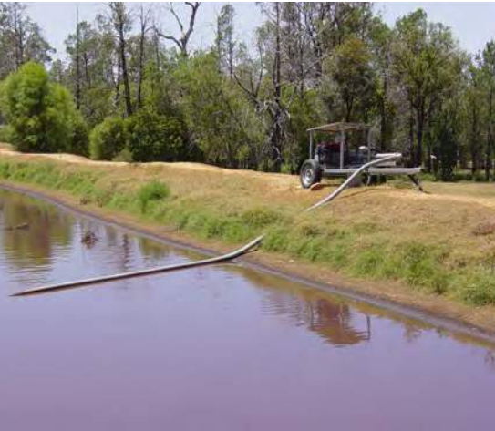
Effluent irrigation pumping site on holding pond embankment.
