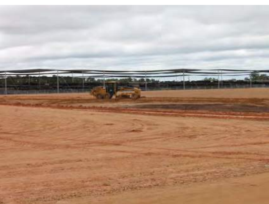
Final trim operations result in a well-prepared pen surface.
