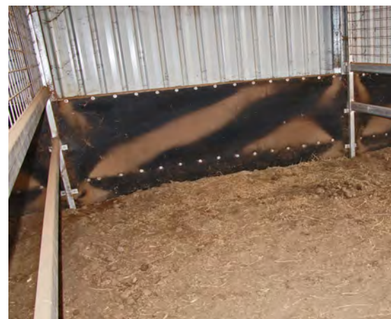
Bedding in stables with no adjoining run-out area. Note conveyor belting covering the iron sheeted wall at the back of the stall.
