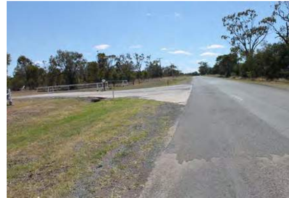
Concrete pavement on feedlot access road to prevent road damage caused by heavy vehicle traffic at turn-in and turn-out
