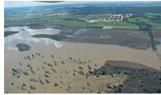
Holding pond located outside of the 1-in-100 year floodplain
