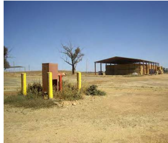
Fire hydrant located near the hay storage area.
