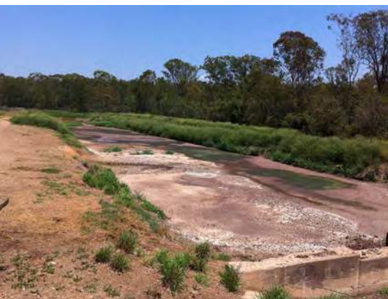
One cell of a sedimentation terrace with multiple cells – drying out after runoff
