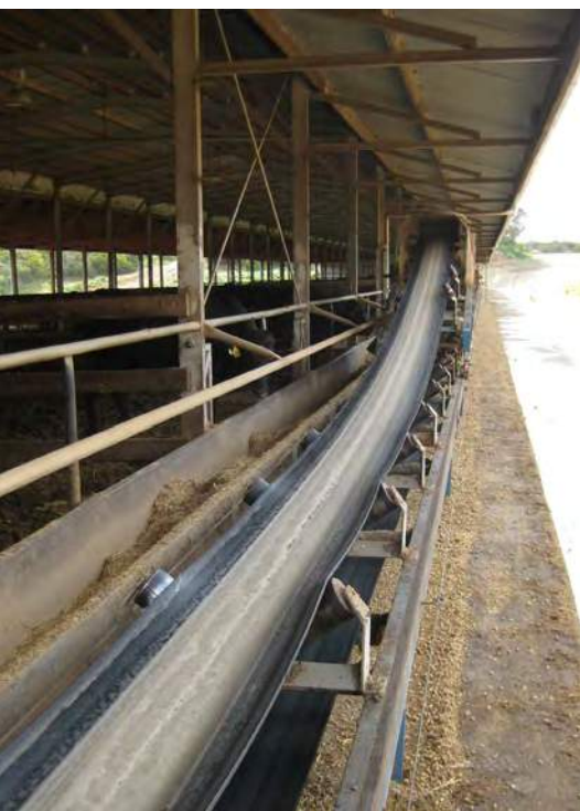
Single row housing with delivery of feed by gantry system running on fixed rails and connected to conveyor belt.
