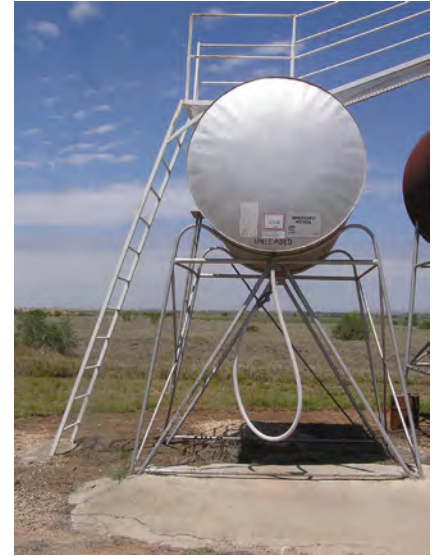
Four legs on support structure with braces close to their base, legs and bracing straight, in good condition and securely attached. Ladder sound and secure, all rungs present, suitable hand holds near ladder.
