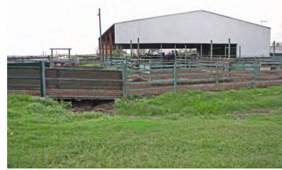
Steel frame building over entire processing area. One third of the shed is fully enclosed for storage and two side walls are half-sheeted from the top for protection against rain and wind. The north-facing wall is not sheeted.
