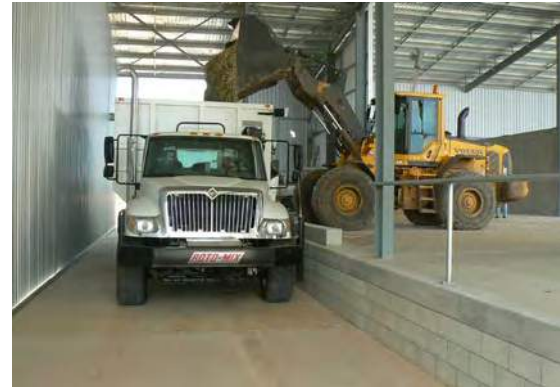
Differing heights between the commodity storage area and the feed vehicle loading bay allow ease of operation and safety.
