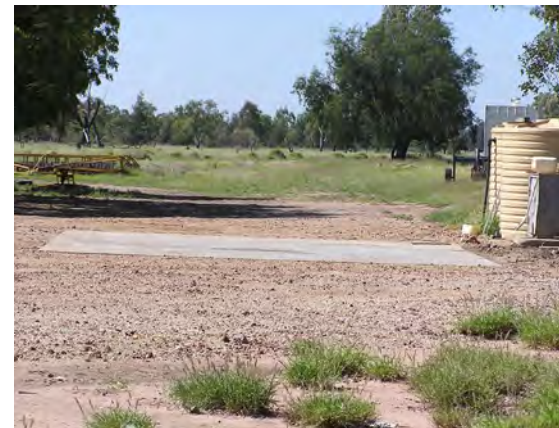
This small concrete pad has limited downslope with no wastewater containment.
