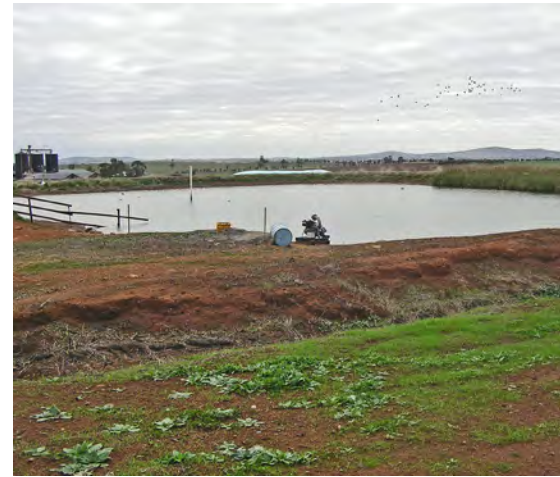
Water storage at a higher elevation than the feedlot allows gravity flow of water.
