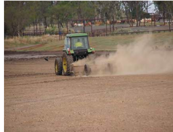
Maintenance of the base of the sedimentation system with a box scraper. Dual sedimentation structures before the holding pond will allow one to be de-silted while runoff is diverted to the other.
