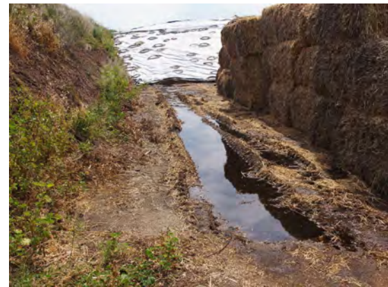
A poorly drained bunker floor allows leachate to remain in the bunker area. The soft floor allows ruts from machinery – exacerbating the problem.
