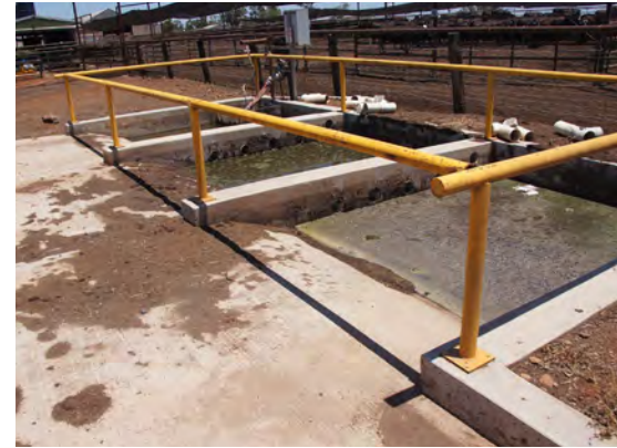
Triple-bay trafficable sediment trap. Drainage water can be directed to other basins to allow sediment to dry out.
