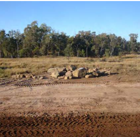
Unsuitable material such as large rocks should be excluded from earthworks.
