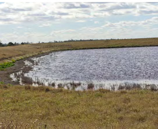
Holding pond with well-grassed batters (to resist erosion) and with sufficient freeboard.
