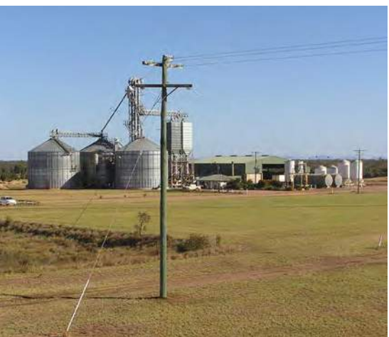
Overhead supply direct to on-site feed processing facility. This is located to avoid accidental contact with high machinery.
