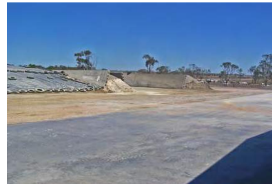
An above ground bunker storage with pre-cast concrete panels laid against the earth embankment. These bunkers are located next to the commodity shed for easy access.
