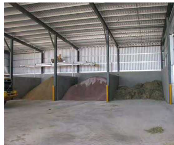
Commodity storage shed with multiple storage bays.
