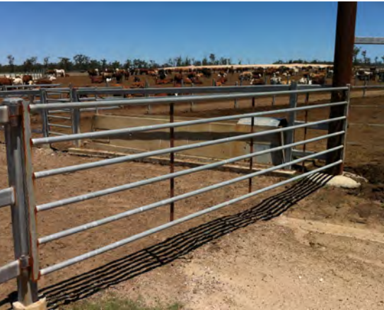
Welded-on round barrel hinges are simple and effective. The swing angle can be limited by the way the hinges are mounted to one side of the post.
