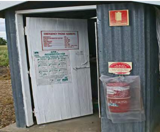
Appropriate signage should be clearly visible on the exterior of the storage facility.
