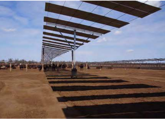
Shade structures – longitudinal rows
