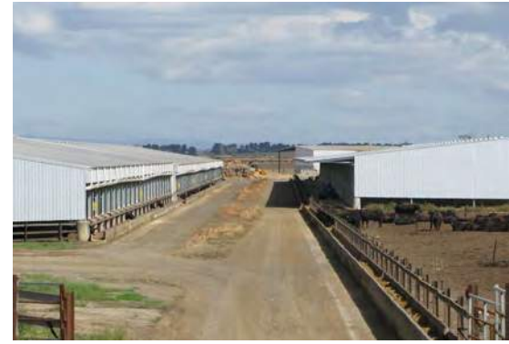
Roof water collection system
