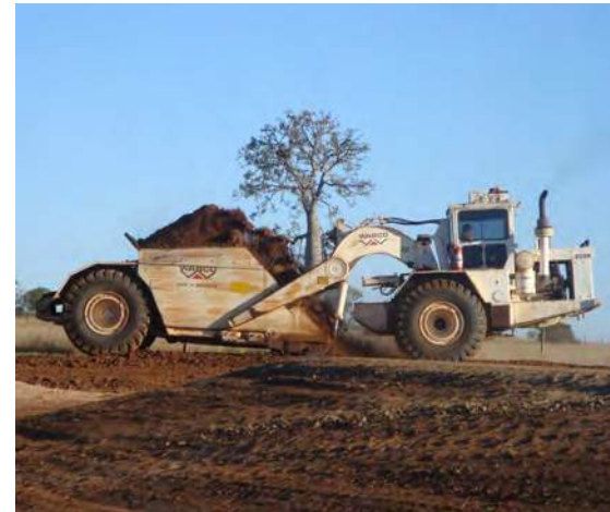
Step 3. Removing topsoil
