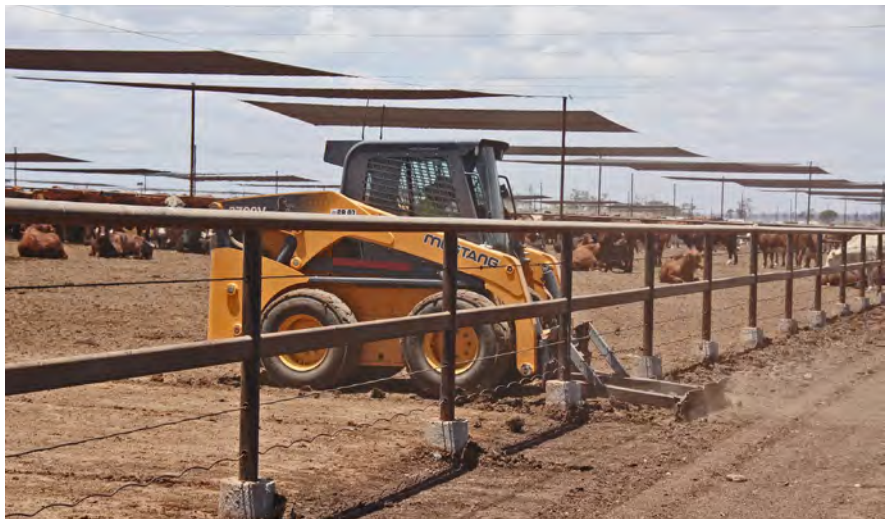
The height of the bottom cable must allow under-fence cleaning, Some flexibility in the strain reduces damage. Here, curly cable is used only in the lowest cable.
