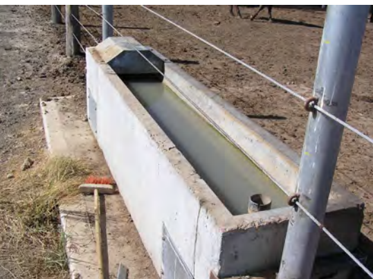
Placing troughs between pens can help secure water supply to cattle. Note good float protection, enclosed sides and an overflow pipe. The trough can be scrubbed with a brush for cleaning.
