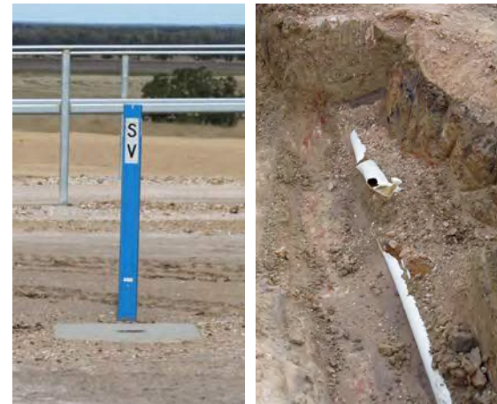
Marking and recording the location and depth of underground mainlines will prevent unnecessary and costly damage.
