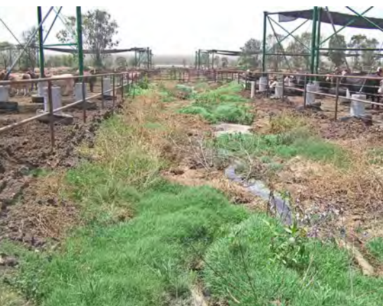
Primary drains with vegetation as surface cover are difficult to maintain as they remain wet, the vegetation grows and manure is deposited. These areas can be a source of excessive odour emission and a fly breeding site.
