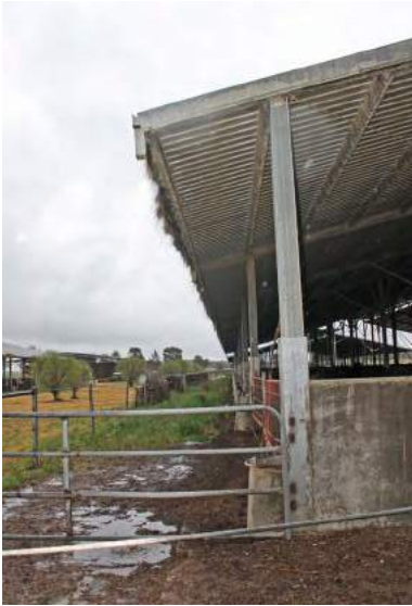
Half-covered cattle lane running length of shed – roof is guttered to prevent runoff directly into cattle lane.
