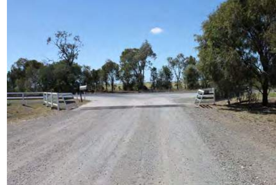
Turn-in and turn-out from feedlot access road onto minor rural road – sufficient area is provided for vehicle turning.
