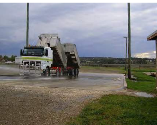
Concrete pad of suitable length and width for semi-trailers; 4% downslope provides excellent self-cleaning and drainage.
