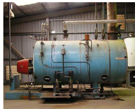
Boiler for the steam-flaking process. Steam generation is the largest single consumer of energy in a feed processing facility.
