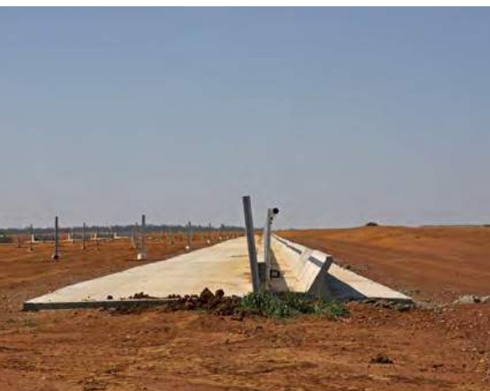
Concrete aprons on pen and feed road sides
