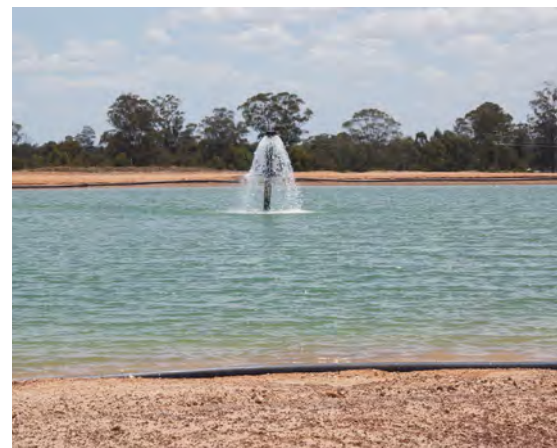
Artesian water may need spray cooling.
