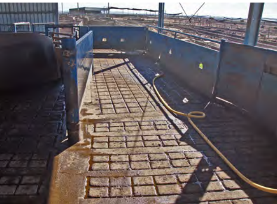
Stamped concrete with square pattern aligned along direction of flow. The lack of grooves on left where cattle turn is not ideal.
