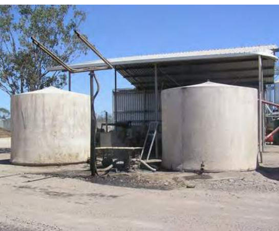
Liquid supplement storage and dispensing system at small feedlot.
