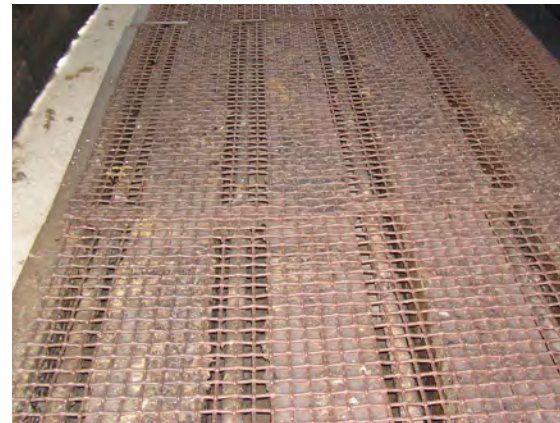
Concrete floor with recessed pipework and mesh to provide non-slip surface
