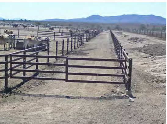
Cattle lane and catch drain – Option 3. The cattle lane and the catch drain are combined, but a control bank on the outside of the cattle lane fence keeps runoff in the lane.
