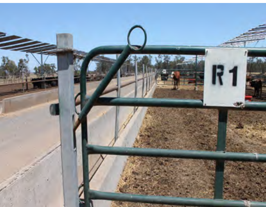
The circular grip on this telescopic pipe latch minimises the risk of pen riders getting snagged. Half circle gate stops prevent cattle damaging the latch when rubbing and allow the gate to be opened in one direction only.
