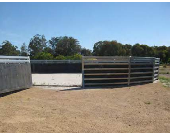
Exercise/training yard with sand bedding and lined inner walls
