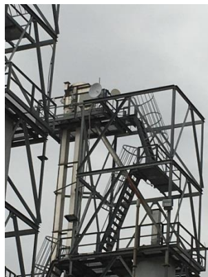
Figure 31 External connectivity. The microwave point-point link from the top of the Mill tower. Voice
