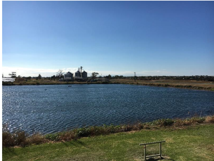
Figure 17 70ML storage dam (foreground) and Mill pump (background) linked to an alert system via the mobile phone network (4G tower ~ 10 km away).
