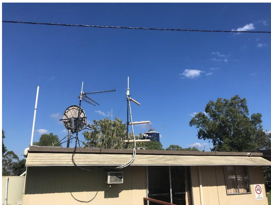
Figure 29 Internal point to point links utilises Wi-Fi operating from the Office. The various receivers show the 'history of connectivity' at L4.
