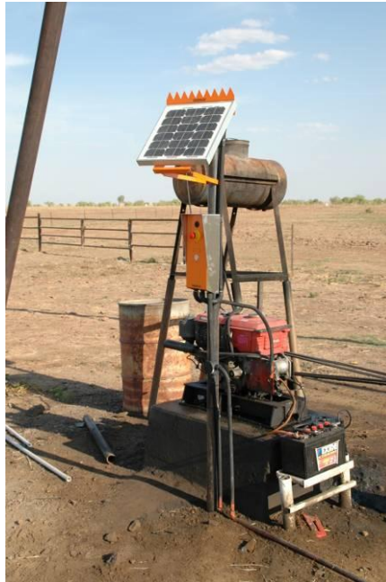
Phase II Trial: M1 Pump Controller installed at No 12
