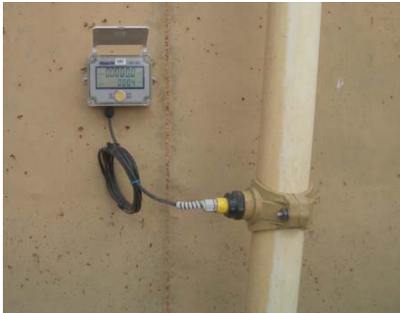
Photograph 29 – Installed water meter M8 at Feedlot B
