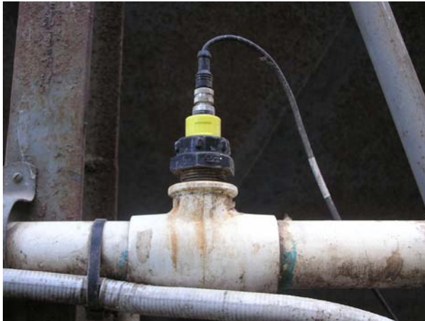
Photograph 37 – Installed water meter M7 at Feedlot E
