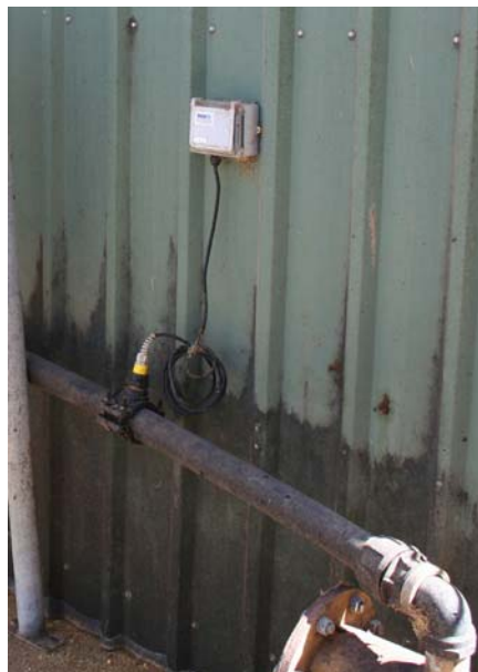
Photograph 24 – Installed water meter M5 at Feedlot A
