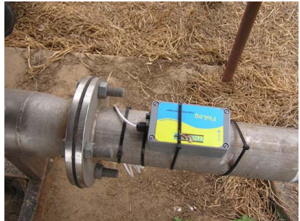
Photograph 44 – Installed water meter M8 and data logger at Feedlot G
