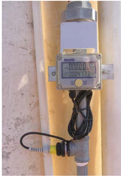
Photograph 43 – Installed water meter M12 at Feedlot F
