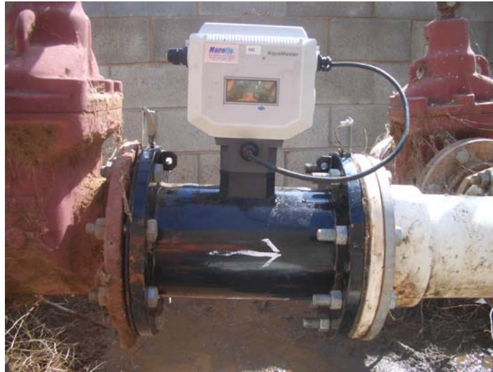
Photograph 31 – Installed water meter M5 at Feedlot C
