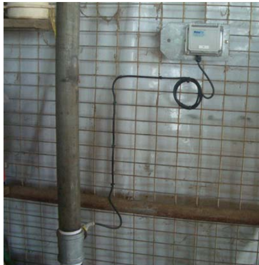
Photograph 41 – Installed water meter M5 at Feedlot F
