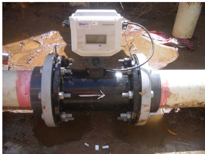
Photograph 30 – Installed water meter M4 at Feedlot C
