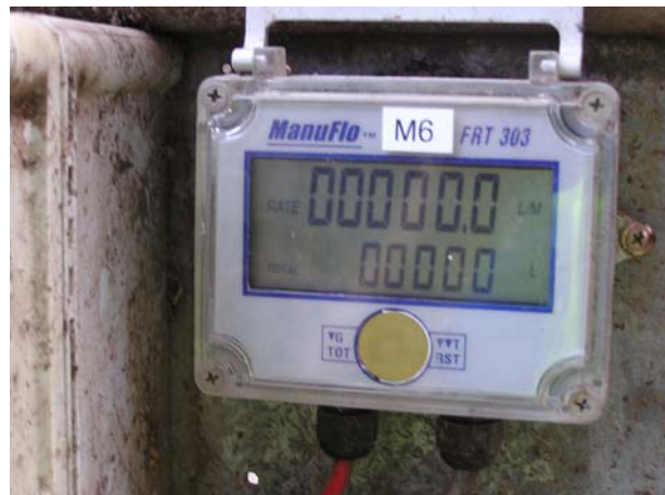
Photograph 36 – Installed water meter M6 at Feedlot E
