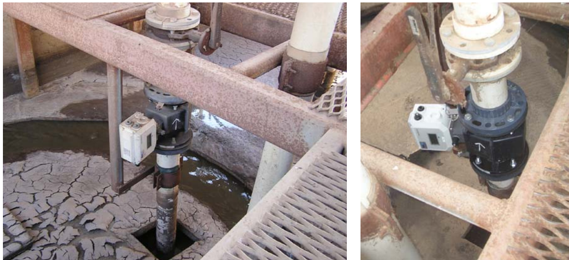
Photograph 34 – Installed water meter M8 at Feedlot C
