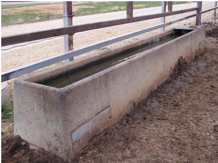
Photograph 61 – Type 3 trough with semi-circular cross-section (Feedlot F)
