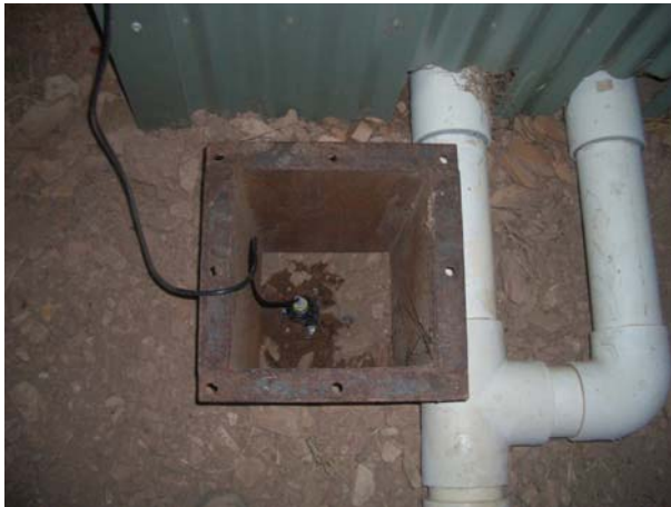
PHOTOGRAPH 27 – INSTALLED WATER METER M4 AT FEEDLOT B
