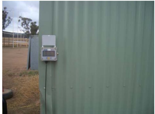
PHOTOGRAPH 27 – INSTALLED WATER METER M4 AT FEEDLOT B
