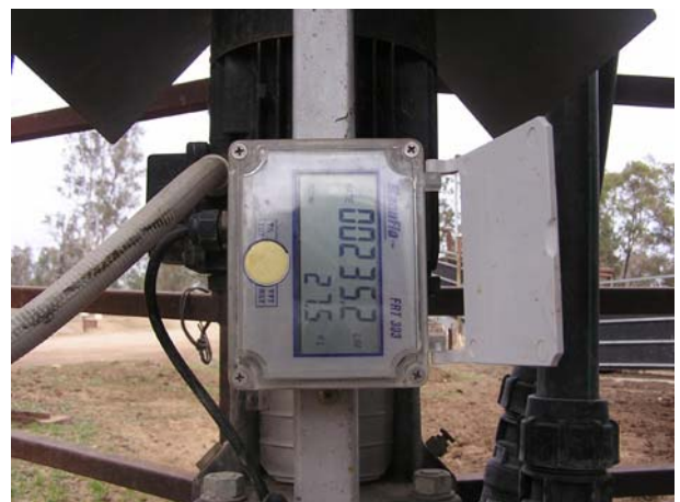
Photograph 47 – Installed water meter M3 at Feedlot H
