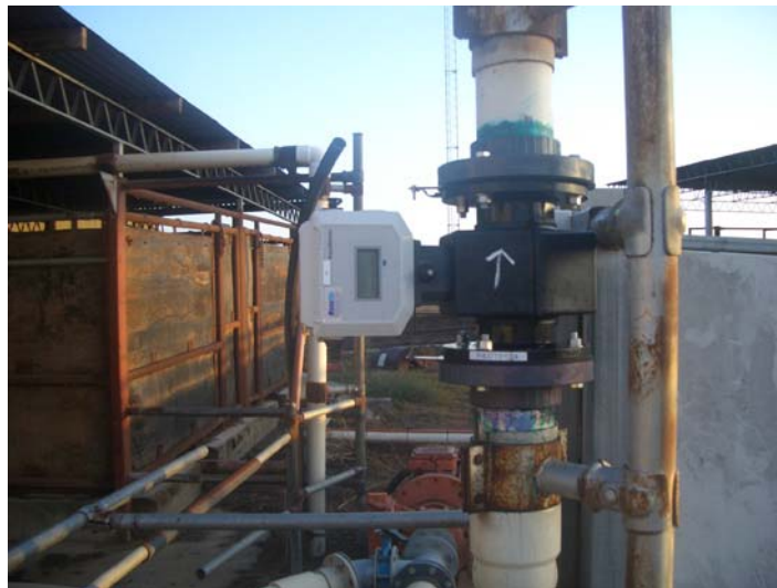
Photograph 33 – Installed water meter M7 at Feedlot C
