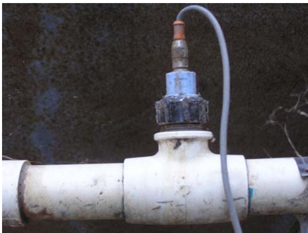
Photograph 36 – Installed water meter M6 at Feedlot E
