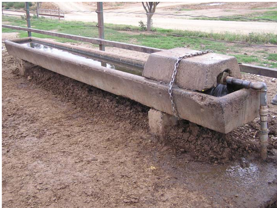
Photograph 59 – Old Type-1 style trough with trapezoidal cross-section and concrete float valve cover (Feedlot F)
