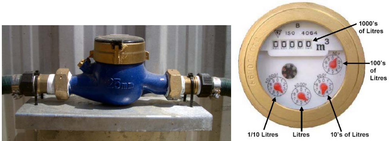
Photograph 18 – ManuFlo MEH Multijet water meter
