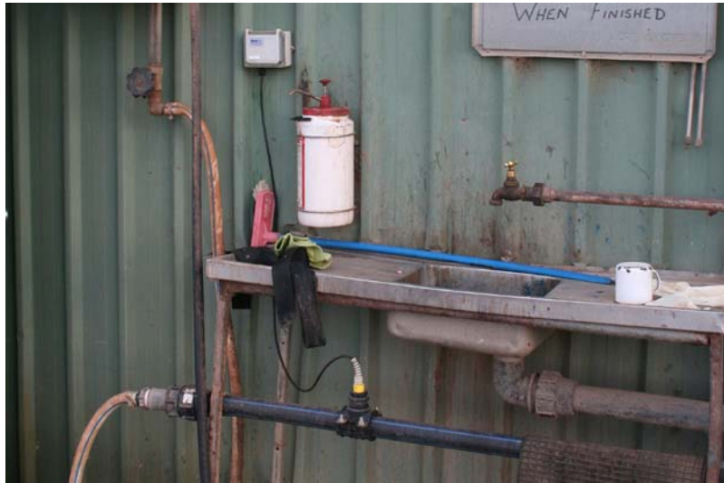
Photograph 23 – Installed water meter M3 at Feedlot A
