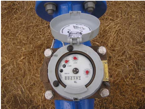
Photograph 44 – Installed water meter M8 and data logger at Feedlot G
