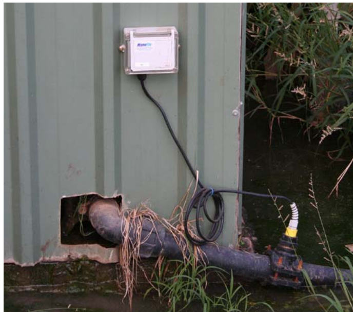
Photograph 25 – Installed water meter M6 at Feedlot A
