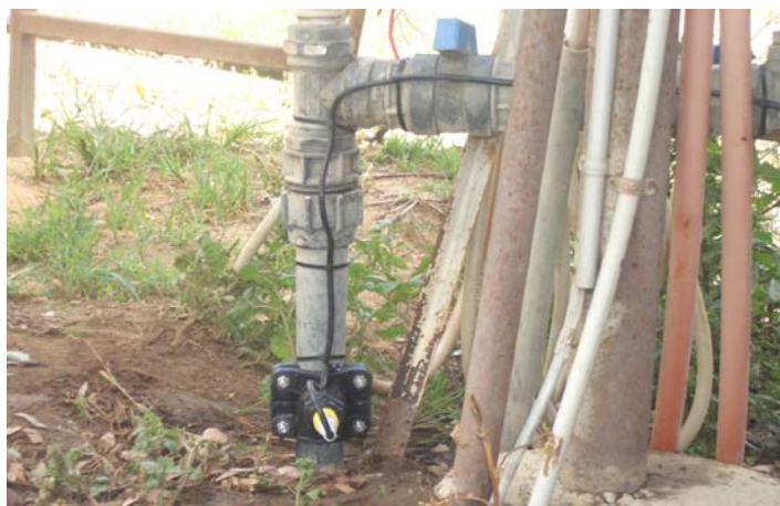
Photograph 47 – Installed water meter M3 at Feedlot H
