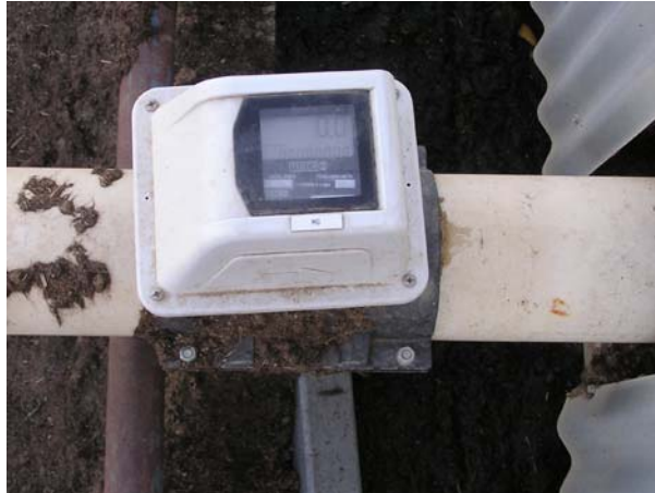
Photograph 42 – Installed water meter M6 at Feedlot F
