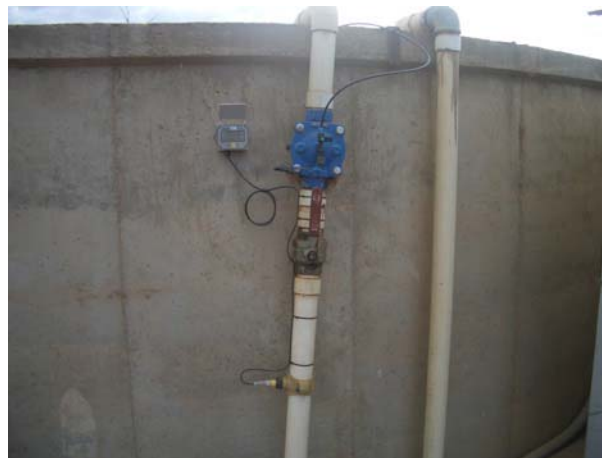
Photograph 28 – Installed water meter M7 at Feedlot B
