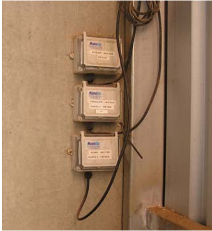
Photograph 35 – Installed water meter M9 at Feedlot C
