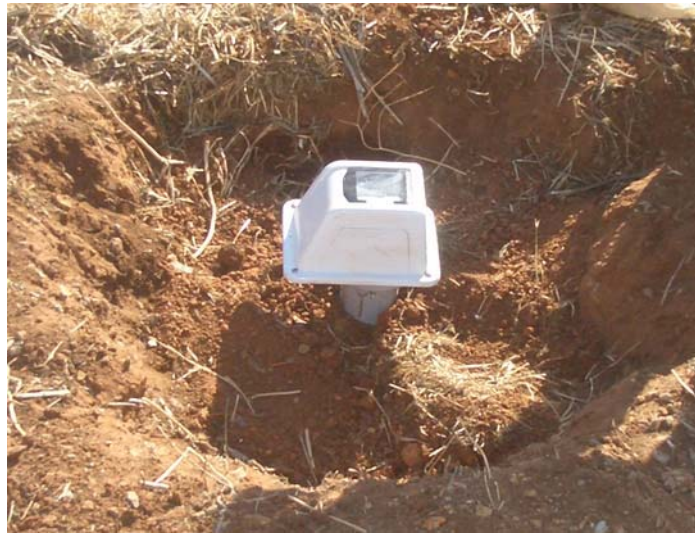
PHOTOGRAPH 32 – INSTALLED WATER METER M6 AT FEEDLOT C
