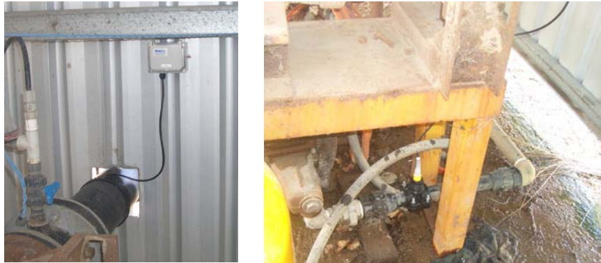
Photograph 39 – Installed water meter M3 at Feedlot F
