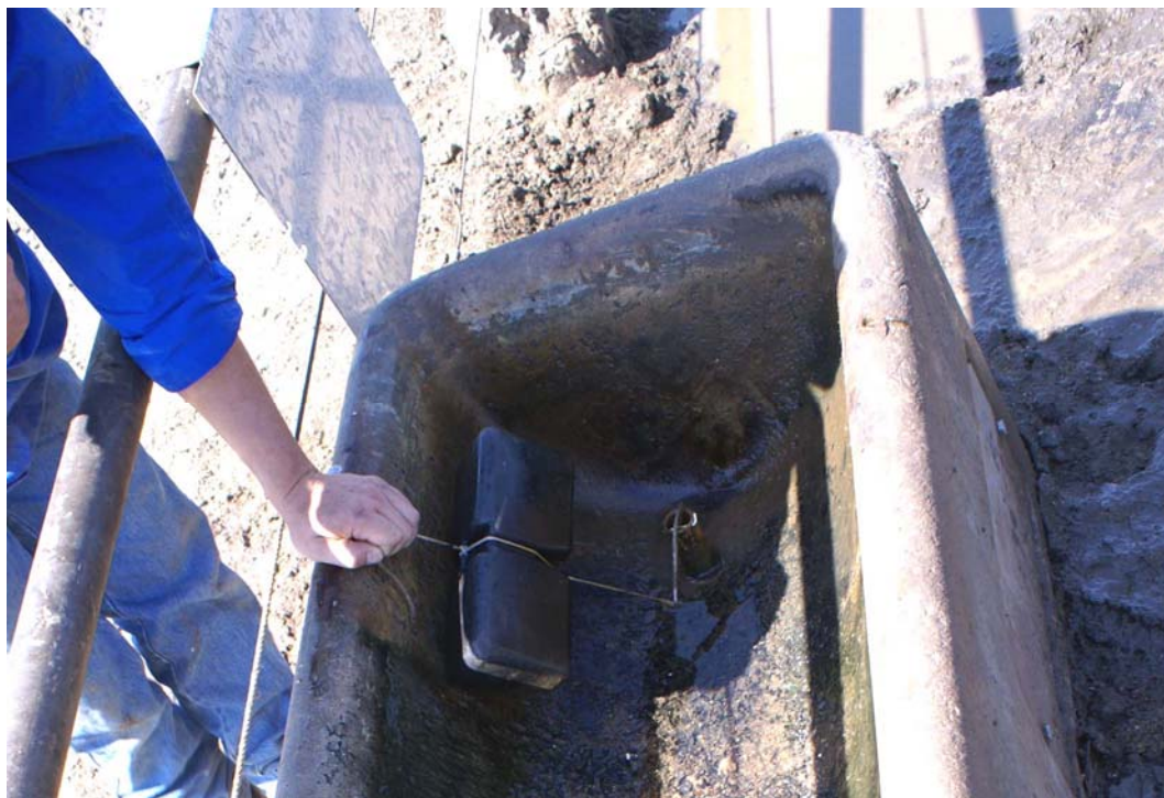
Photograph 51 – Float valve – plastic float on a rope – valve sprays upwards (Feedlot B)
