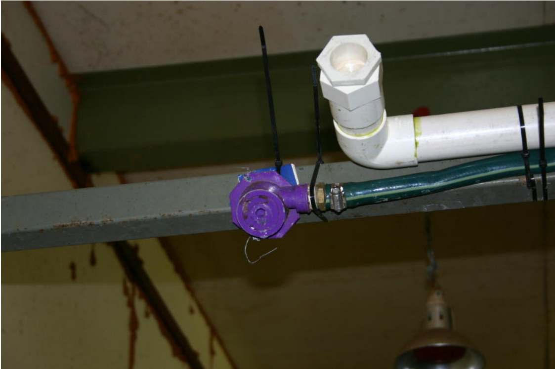
Photograph 4 Overhead sprinkler system (large droplet garden sprinkler)
