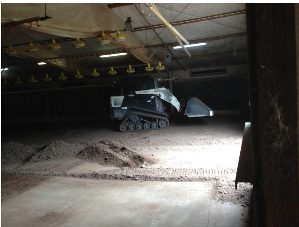
Photograph 2 – Machinery working on cement stabilised broiler shed floor
