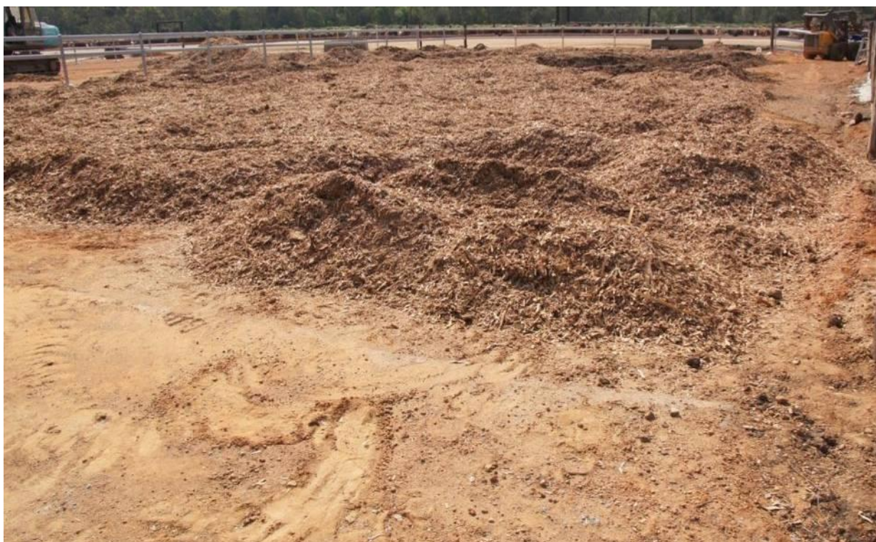
Photograph 4 – Fresh woodchips being distributed to achieve 150-200 mm coverage
