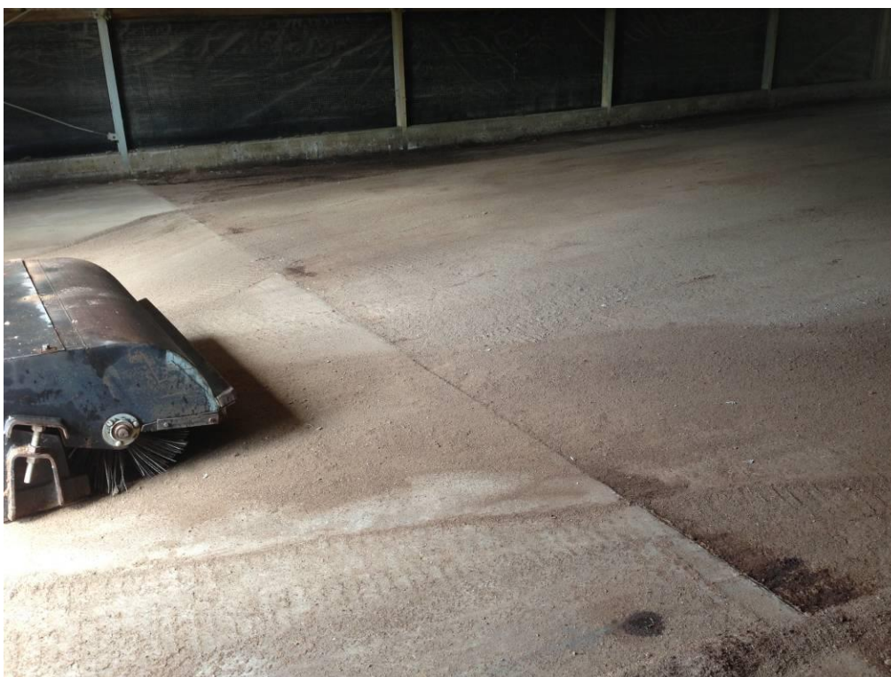
Photograph 3 – Cement stabilised floor surface adjacent to concrete apron
