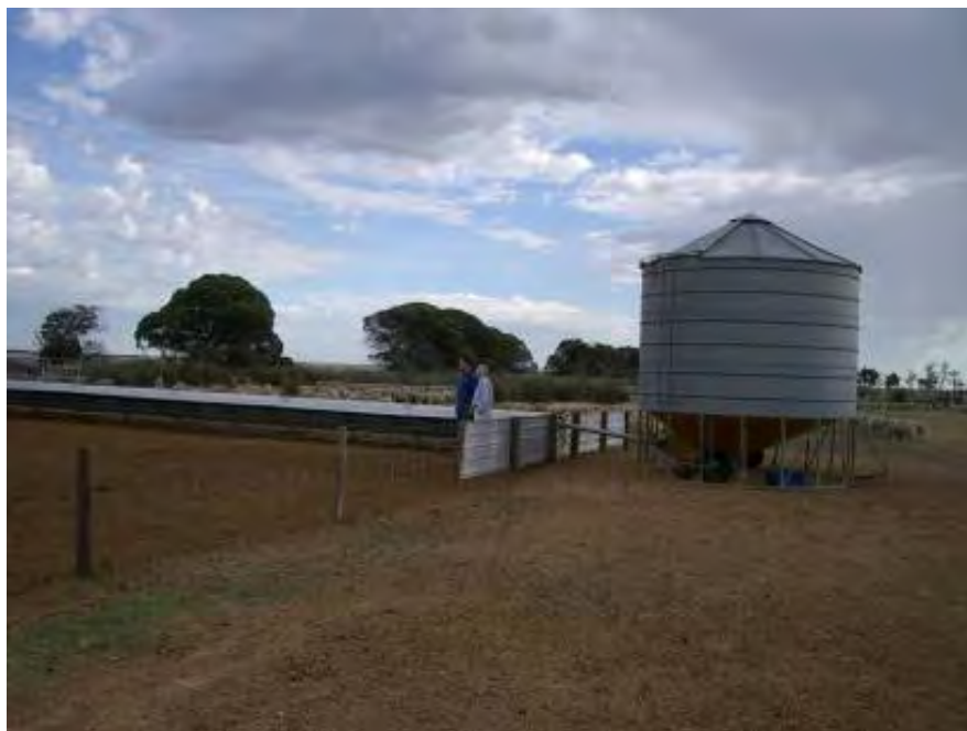
Figure 18 Automated outdoor pellet delivery system, WA (Source: Productive Nutrition Pty Ltd)
