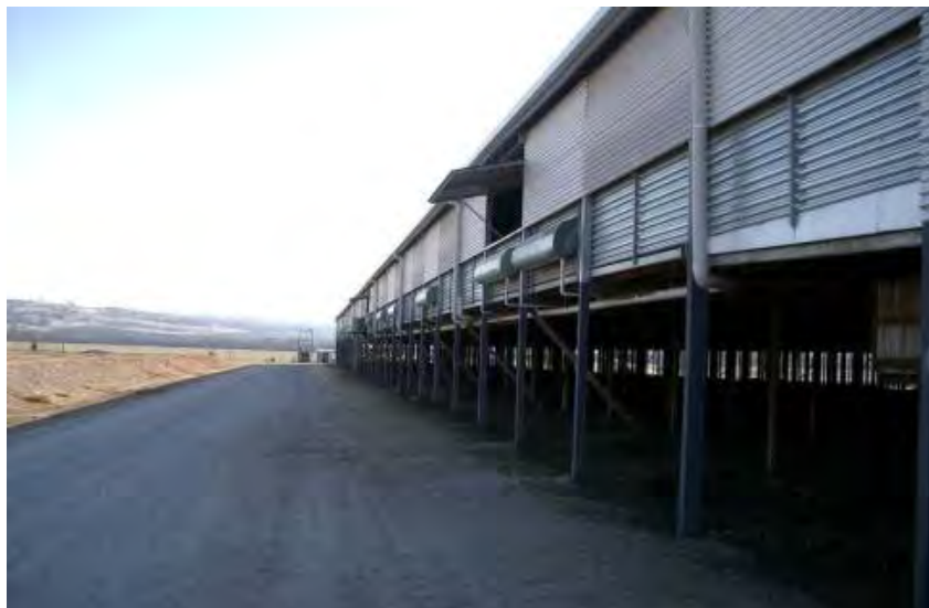
Figure 26 Externally mounted moulded water troughs (Source: Productive Nutrition P/L)
