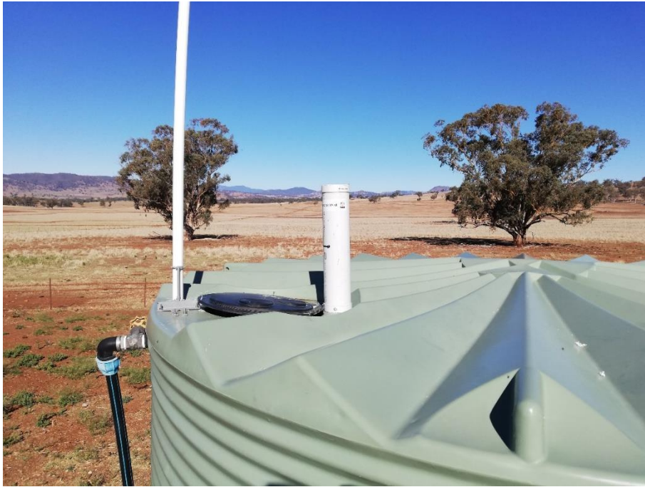
Figure 3-5: Tank Level Installation
