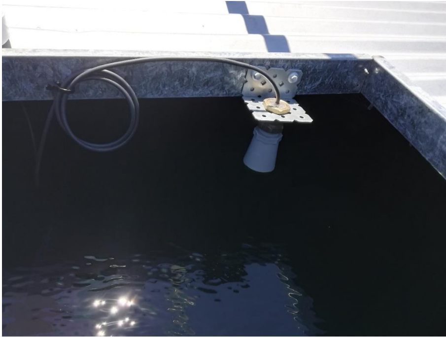
Figure 3-3: Tank Level Installation
