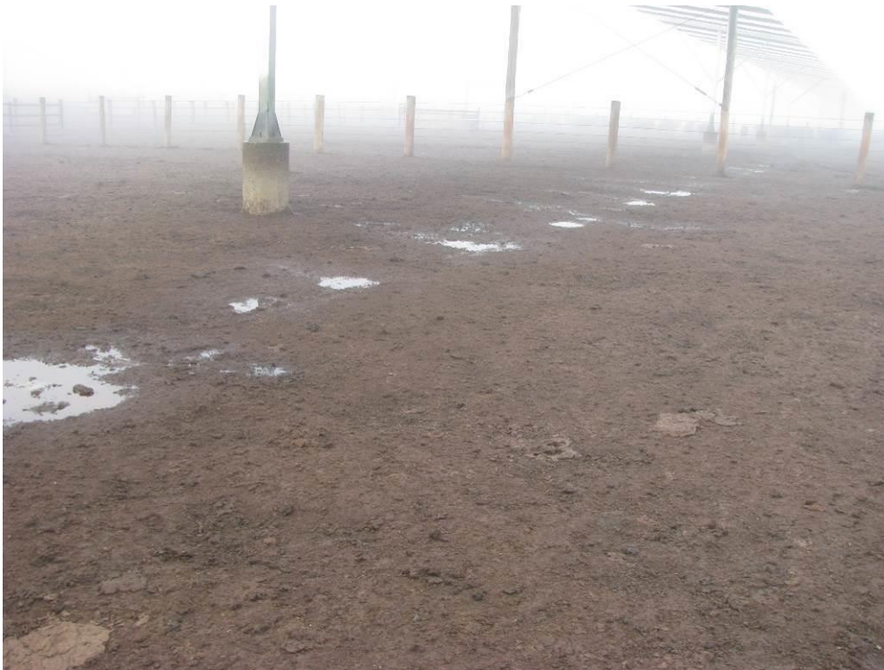
PHOTOGRAPH 50 – POTHOLES DUE TO IRON SHEETING SHADE DRIPPING ONTO THE PEN SURFACE IN THE SAME PLACE
