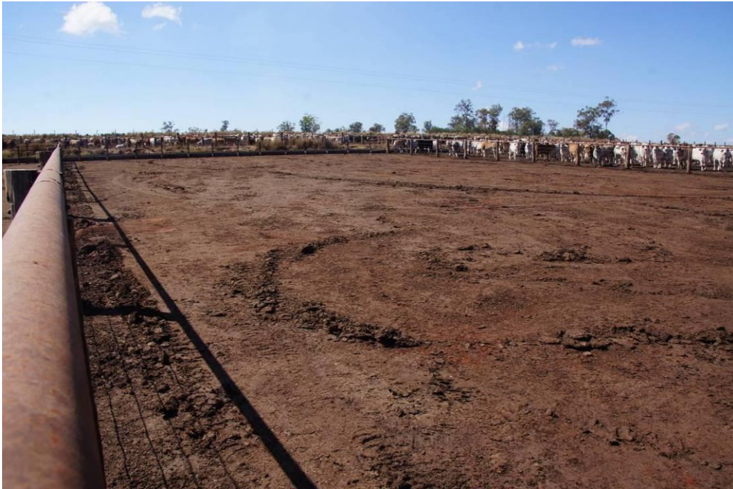
PHOTOGRAPH 30 – TRIAL 1A - PEN AFTER CLEANING AND PRIOR TO WOOD CHIP PLACEMENT
