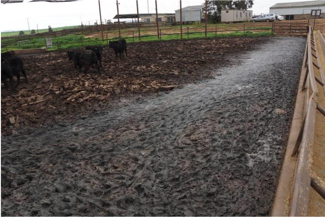
PHOTOGRAPH 13 –TIMBER OFF-CUTS AND CONCRETE FEED BUNK APRON
