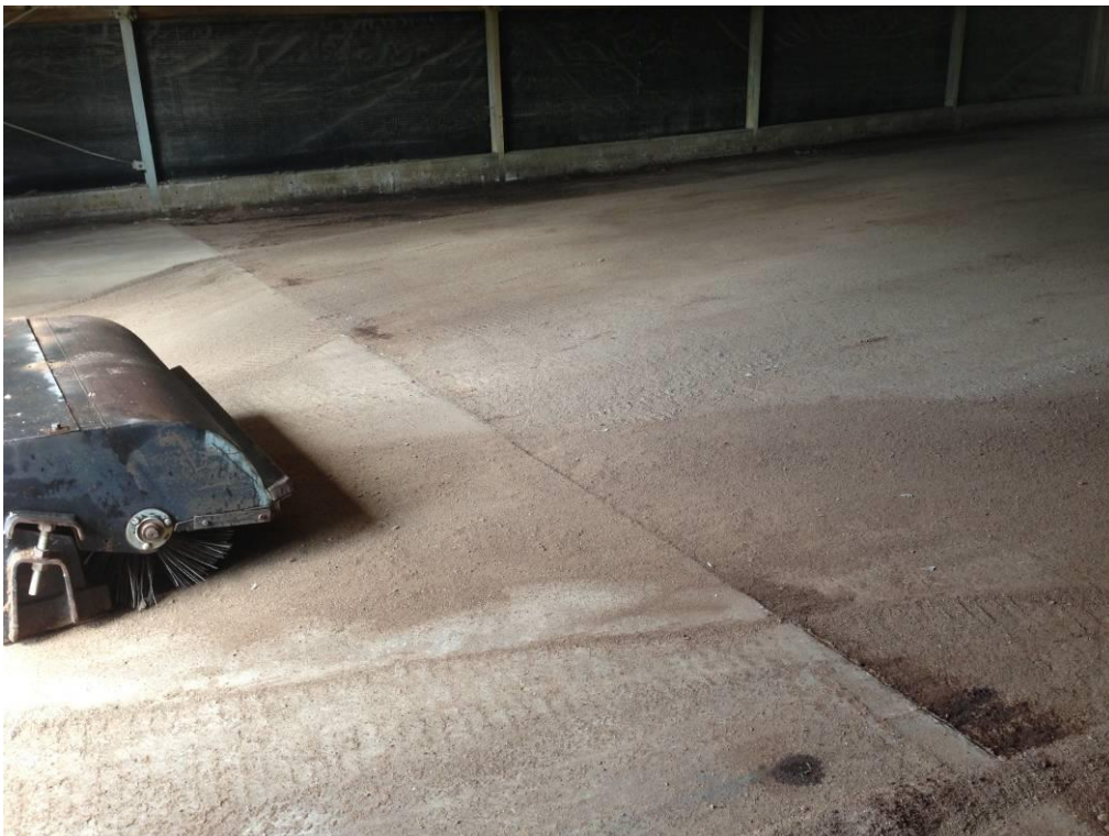
PHOTOGRAPH 3 – CEMENT-STABILISED FLOOR SURFACE ADJACENT TO CONCRETE APRON
