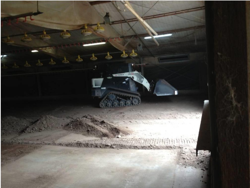
PHOTOGRAPH 2 – MACHINERY WORKING ON CEMENT-STABILISED BROILER SHED FLOOR
