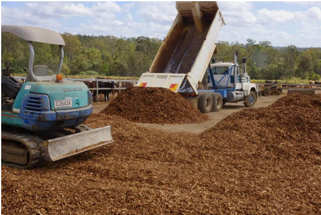
PHOTOGRAPH 61 – FEEDLOT C – PLACEMENT OF 200 MM WOOD CHIPS – PEN 6 (4 SEP 2013)
