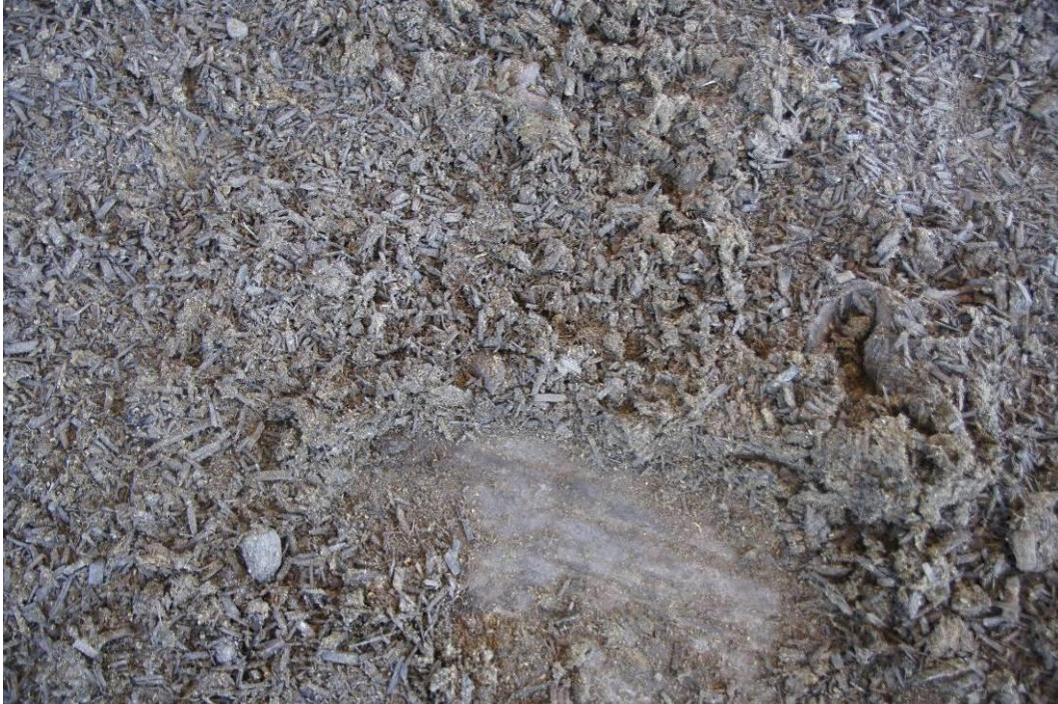
PHOTOGRAPH 40 –TRIAL 2D– THIN LAYER OF WOOD CHIP OVER CONCRETE FLOOR IN COVERED SHEDS
