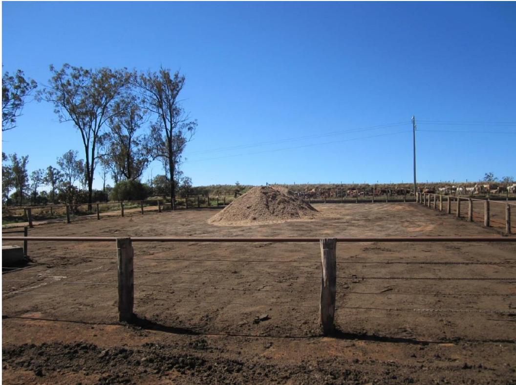
PHOTOGRAPH 32 – TRIAL 3A– 200 M 3 WOOD CHIP MOUND (19 AUG 2013)
