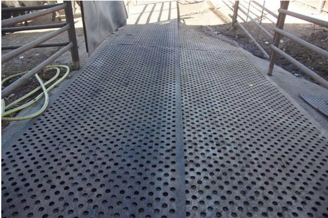
PHOTOGRAPH 29– PERFORATED RUBBER MATTING
