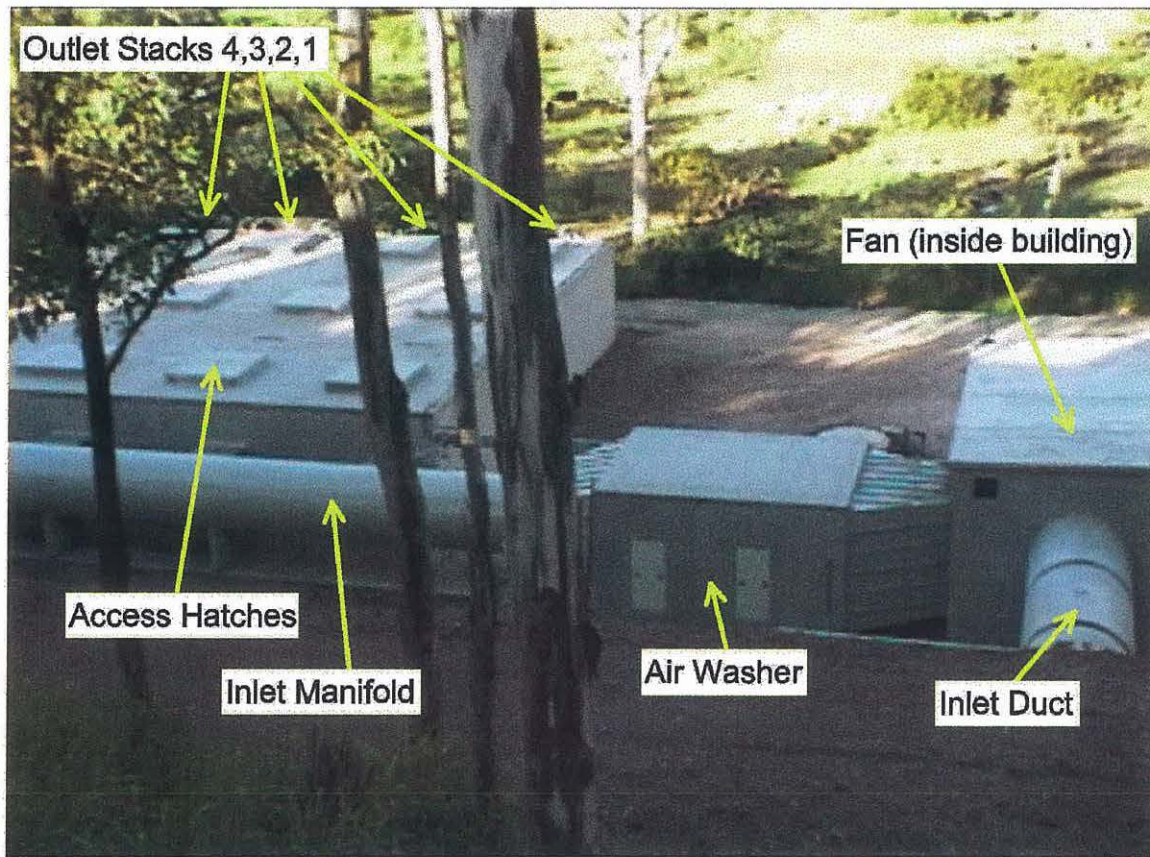
Figure 1 Major Components of the ACC Biofilter
