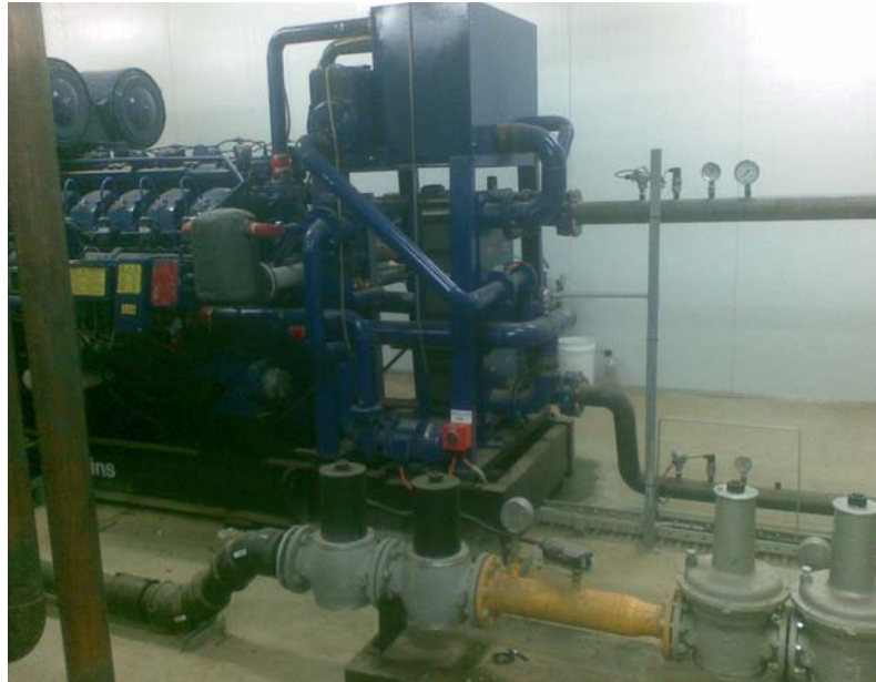
Figure 8 Plate heat exchanger (centre) generating hot water from gas engine water jacket cooling
