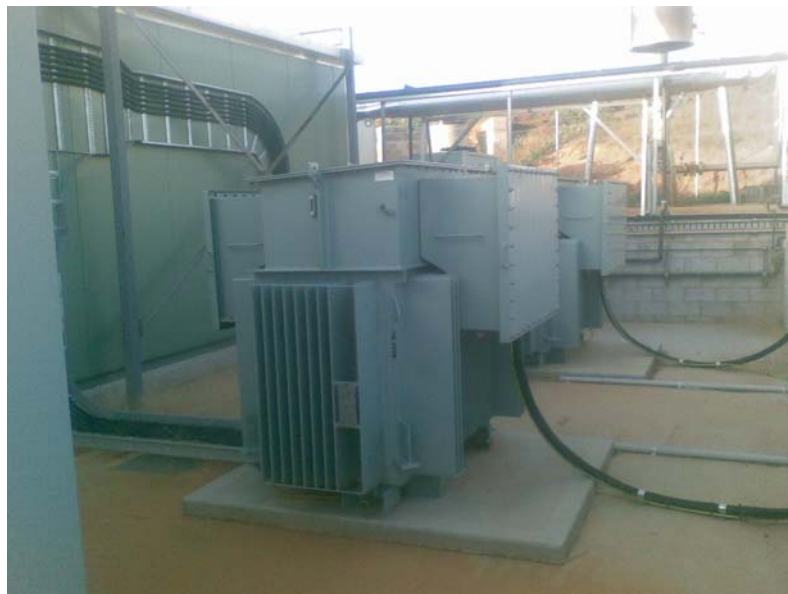
Figure 6 Genset Step-up Transformers
