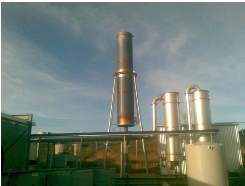
Figure 5 ABM enclosed flare with caustic desulphurisation scrubbers (right)
