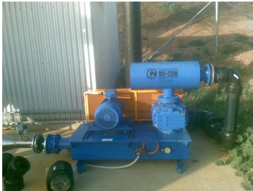
Figure 4 Biogas blower pumping gas to the engines
