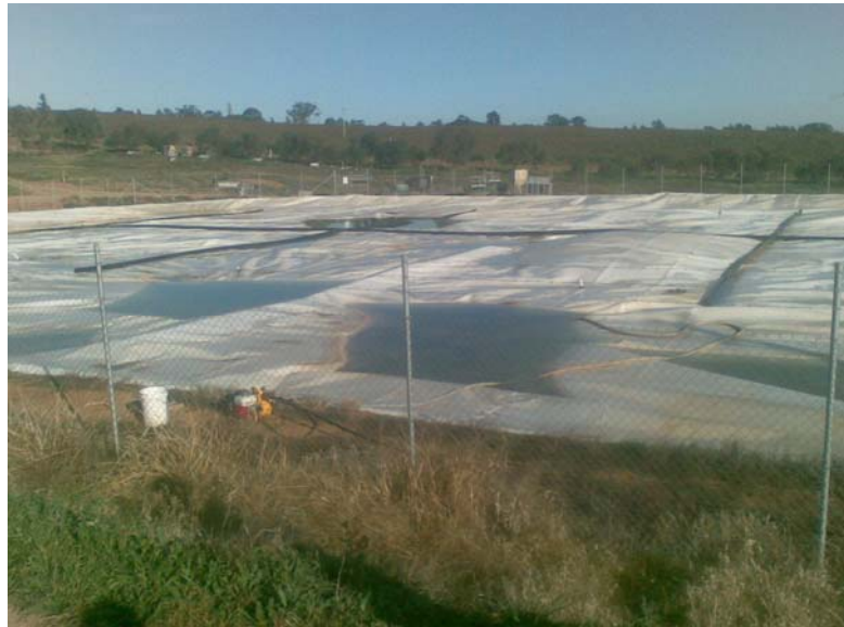
Figure 2 BMP CAL stormwater removal via portable pump.
