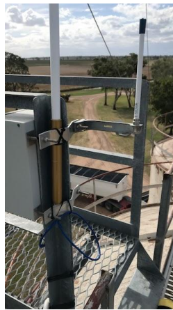
Fig. 5: Box secured to scaffold
