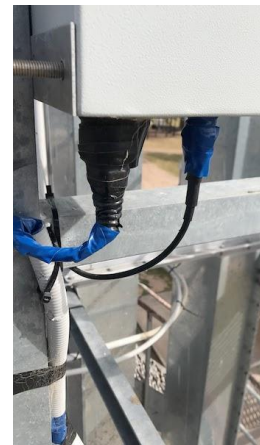
Fig. 6: Wire protection with tape
