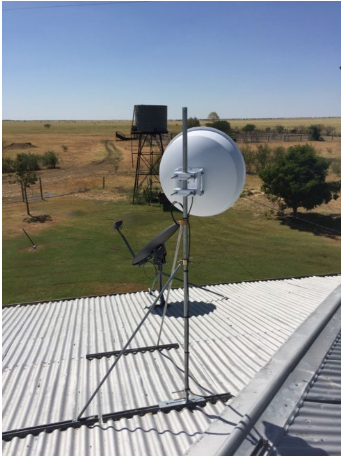
Figure 4: Typical receiving house installation for WiSky solution
