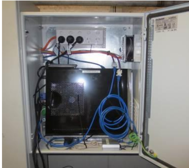
Fig.2 New PC mounted in roof space
