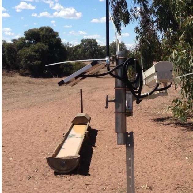
Fig. 4 Remote camera used to monitor a water trough at the Katanning Research Facility.
