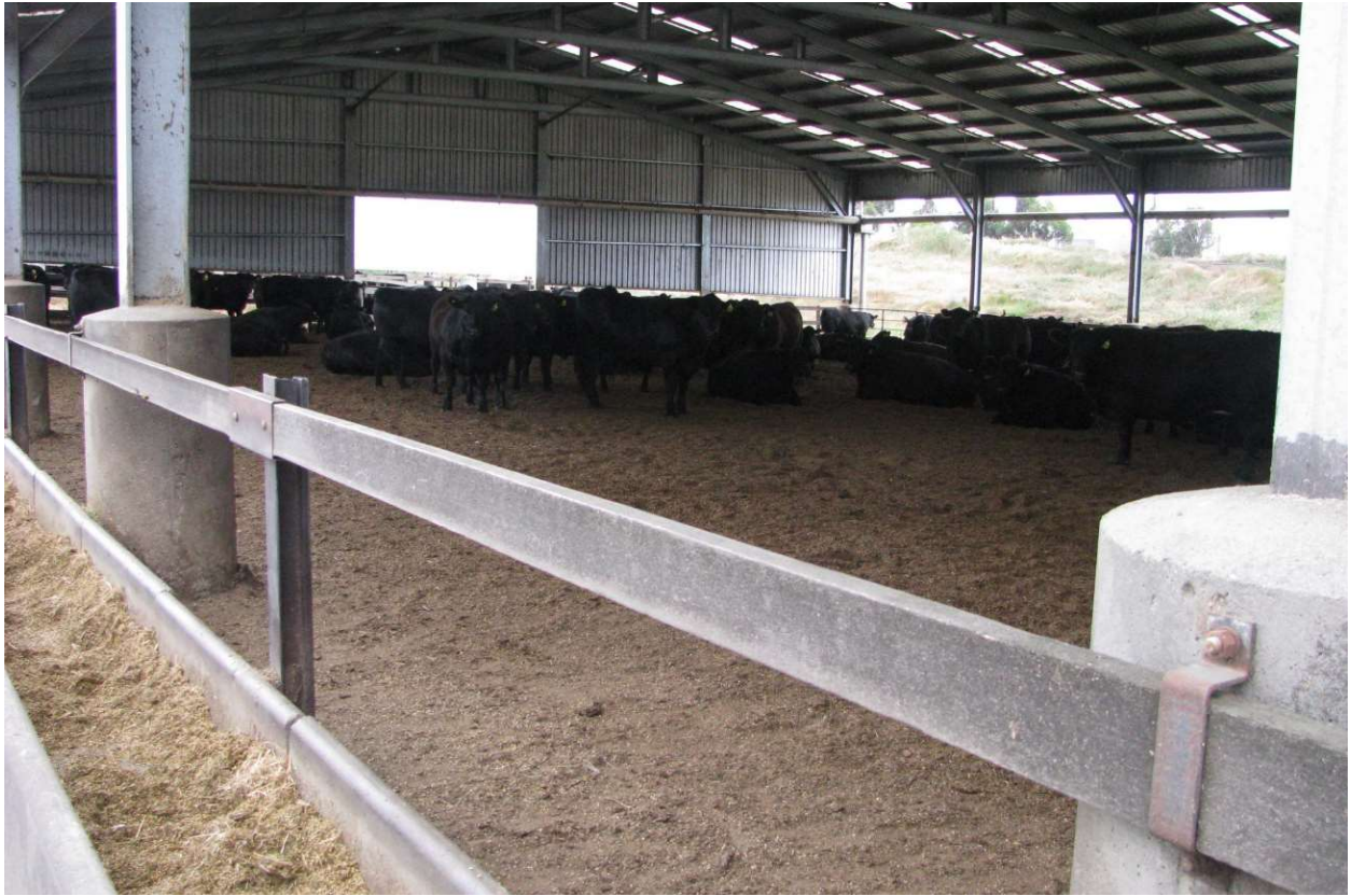
Figure 3-7 – Inside a covered feedlot with 'A Frame' roof. Source: Davis, Watts and Stafford (2016)
