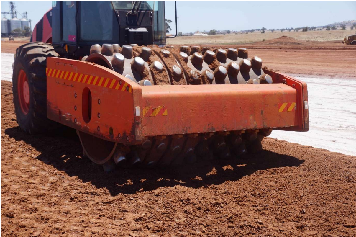
Figure 3. Roller compacting the blended lime and pen surface post mixing. Source Premise Agriculture
