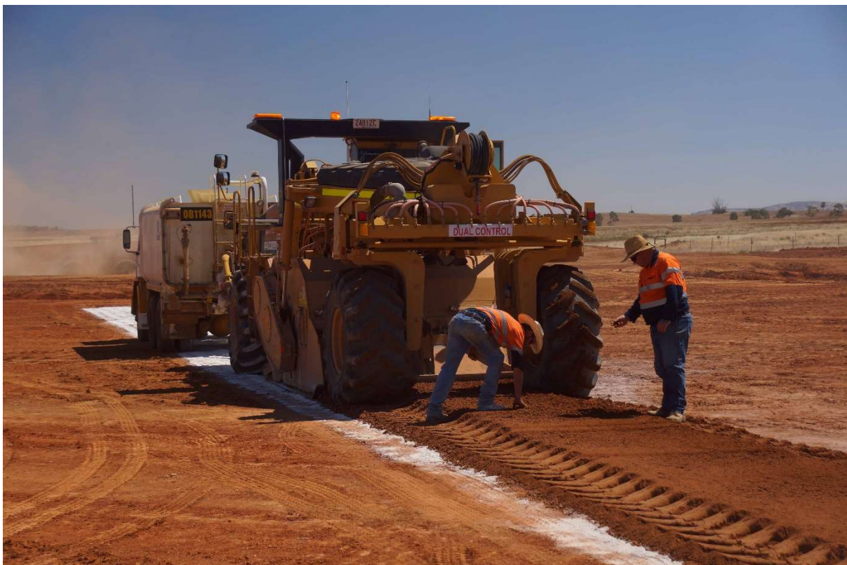
Figure 2. Blending lime into the top 200 mm of the pen surface. Source Premise Agriculture
