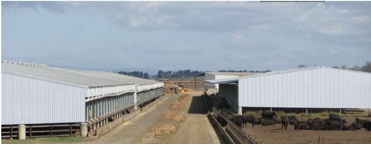
Figure 3-6 – Covered feedlot with 'A Frame' roof. Source: Davis, Watts and Stafford (2016)
