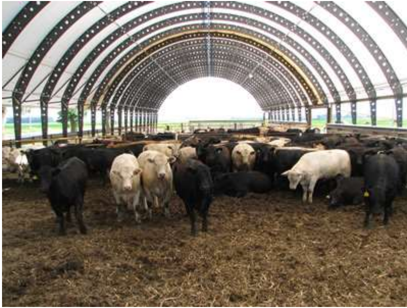
Figure 3-5 – Covered feedlot using a hoop barn structure. Source: Iowa State University of Science and Technology (2018).
