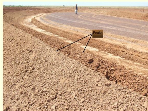
Photo 6. This bank is not domed at the top. This is undesirable, as water will pool between peaks, blow out at the weakest point, and cause the bank wall to wash away.
