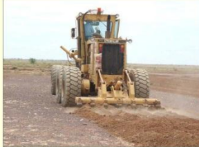
Photo 2. Ripping before bank construction with 16G grader.
