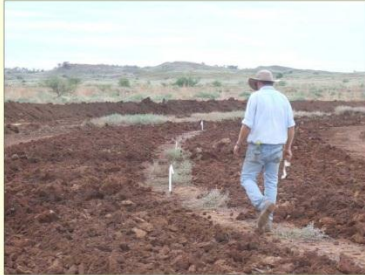
Photo 4. Collecting markers between rip lines before building bank. The non-ripped area between rip lines will form the bank base.
