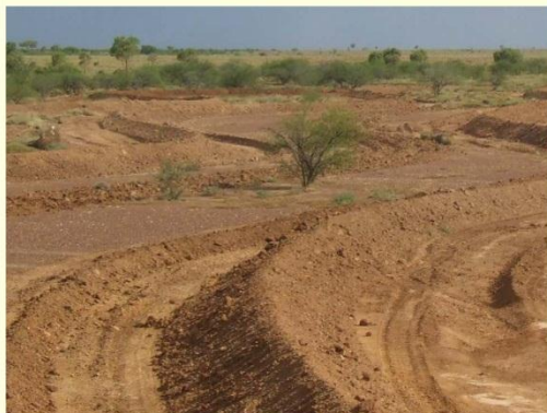
Photo 5. The bank base is 2 m wide and the top is domed. Having a wide base is an important aspect of the design criteria, providing a strong foundation that will reduce the incidence of soil slumping (banks subsiding).
