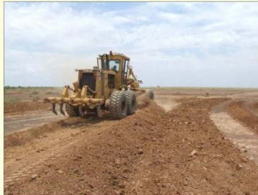
Photo 5. Taking first blade of soil to form bank, starting on outside of pond.
