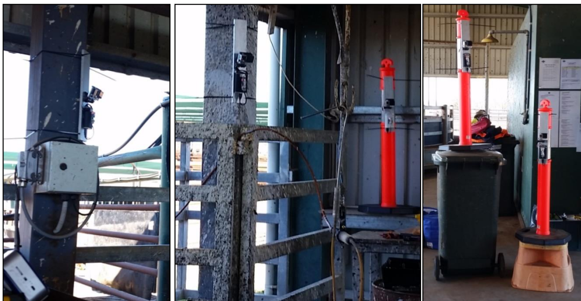
Figure 2. Camera units on posts or portable bollards at an induction facility.
