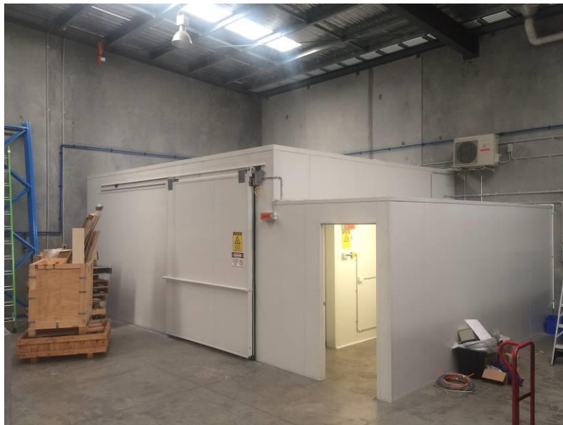
Figure 5: Outside view of room inside Tullamarine facility (Bottom).
